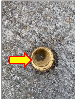
Non-asbestos roofing materials, Roof (Location 0-00).
