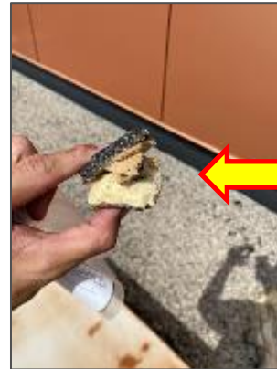
Non-asbestos roofing materials, Roof (Location 0-00).
