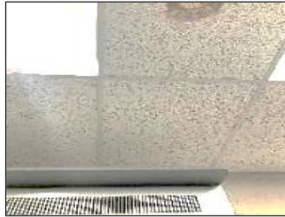
Non-asbestos acoustic ceiling tiles (ACT01).
