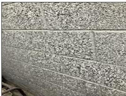
Non-asbestos mortar on masonry wall, Generator Room (Location 1-02).
