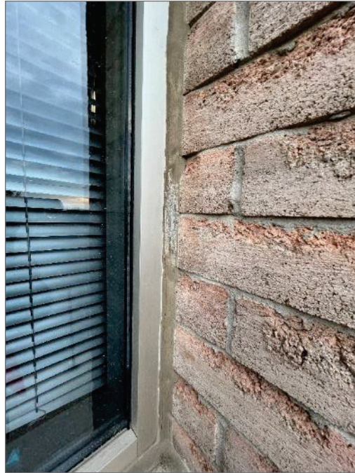
Photo 1 - Non-asbestos light grey caulking around exterior window frame.
