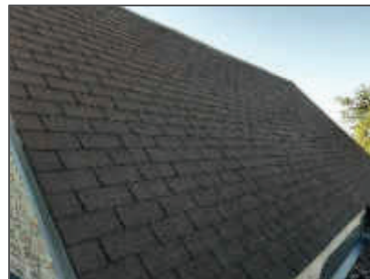
Non-asbestos roof shingles on sloped roof section M (Loc. 5).
