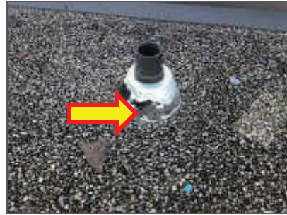
Non-asbestos black mastic on roof penetration (Loc. 4).
