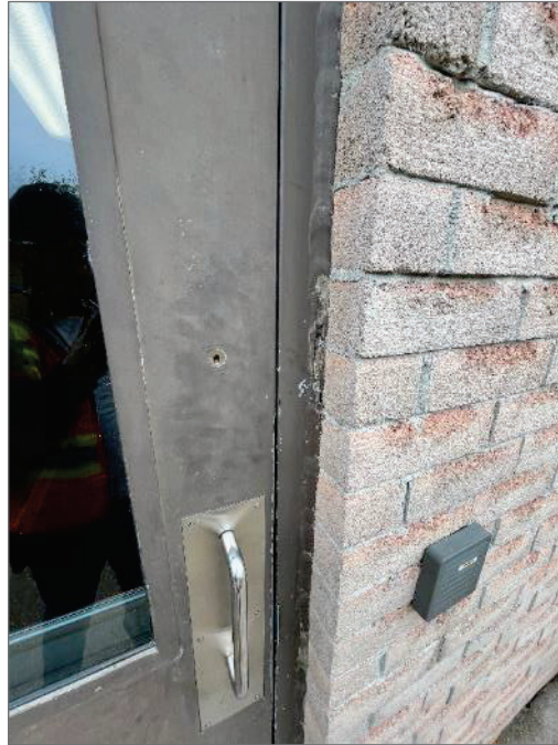
Photo 5 - Non asbestos brown and grey caulking around door frame.
