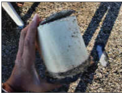
Non-asbestos roofing material on built-up roof section A (Loc. 1).
