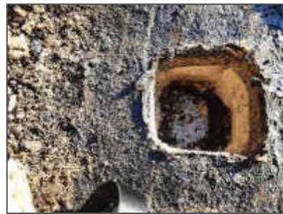
Non-asbestos roofing material on built-up roof section E1 (Loc. 1).
