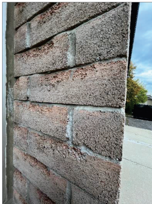
Photo 4 - Non-asbestos mortar between bricks.
