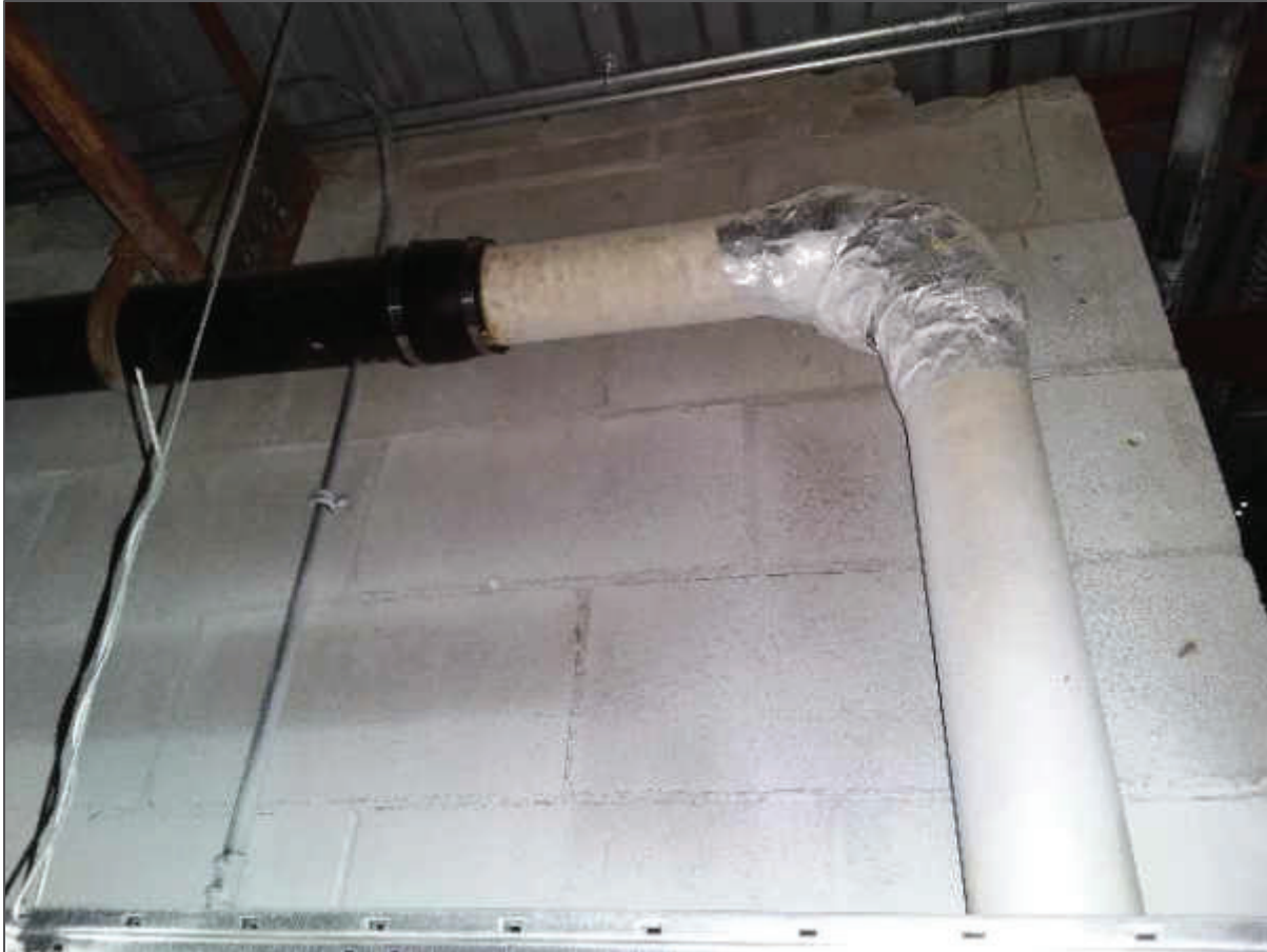
V9000, Cement Product, Front Reception, Offices; Waiting Area (Loc. 8).
