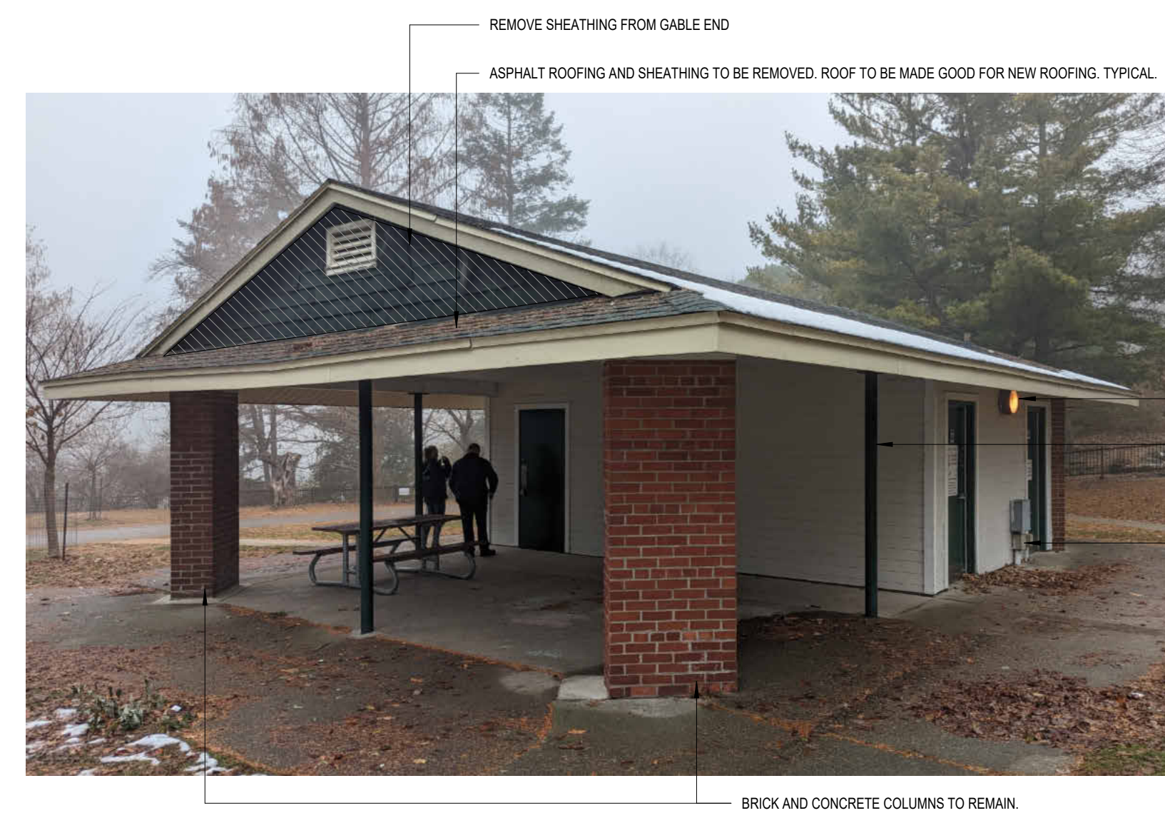
3 EXISTING EXTERIOR VIEW A201 1:10
