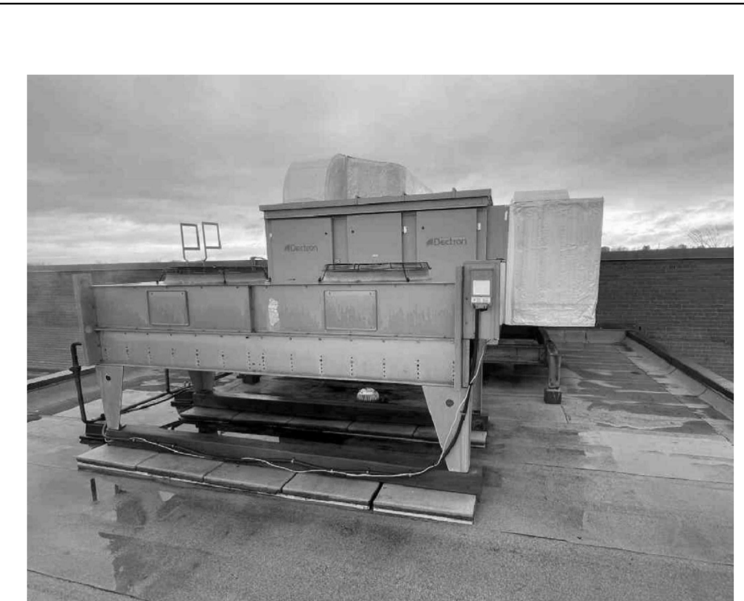
GENERAL PHOTOGRAPH OF MECH. UNITS TO BE REMOVED AND REPLACED
