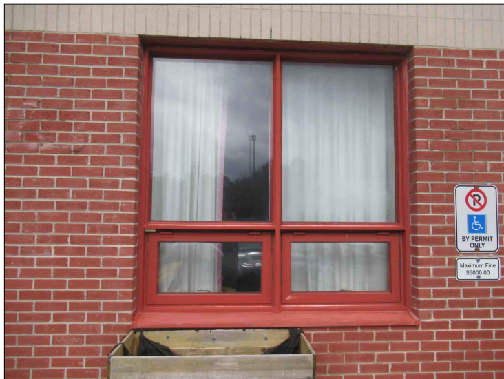
PHOTO 4: VIEW OF EXISTING WINDOW W03A
