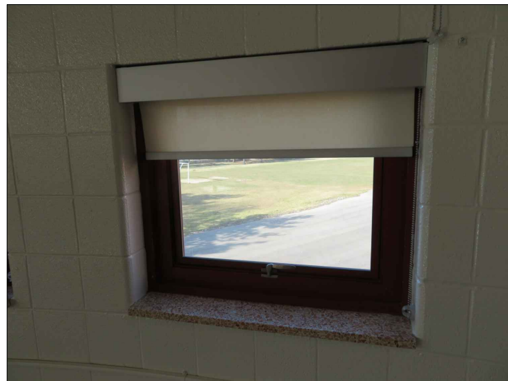
PHOTO 17: ADDITIONAL VIEW OF EXISTING SILL AND BLINDS.
