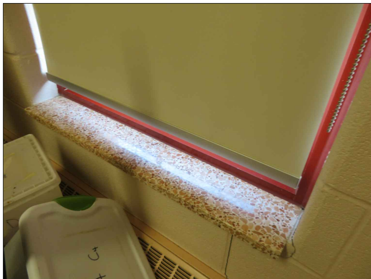
PHOTO 16: TYPICAL VIEW OF EXISTING SILL.
