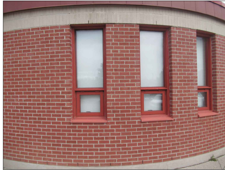
PHOTO 11: VIEW OF EXISTING WINDOW W10
