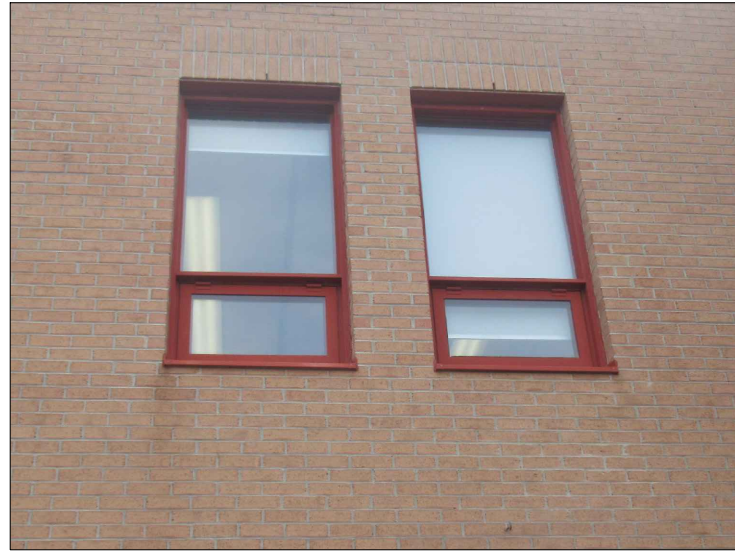
PHOTO 2: VIEW OF EXISTING WINDOW W02
