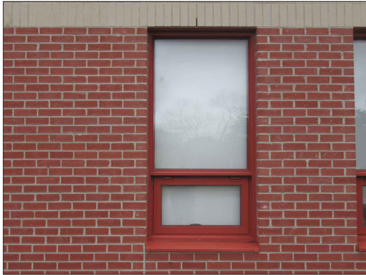
PHOTO 10: VIEW OF EXISTING WINDOW W09
