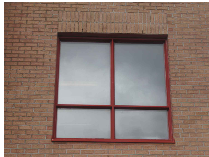
PHOTO 9: VIEW OF EXISTING WINDOW W08
