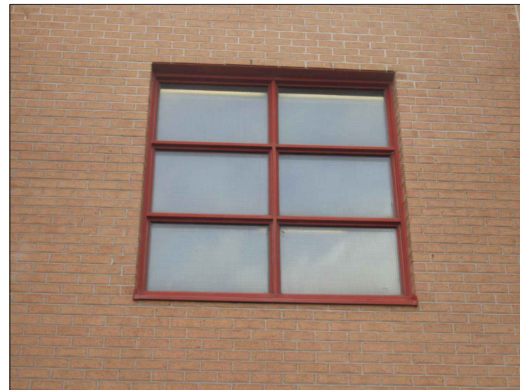
PHOTO 6: VIEW OF EXISTING WINDOW W04
