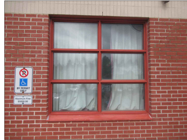
PHOTO 12: VIEW OF EXISTING WINDOW W11
