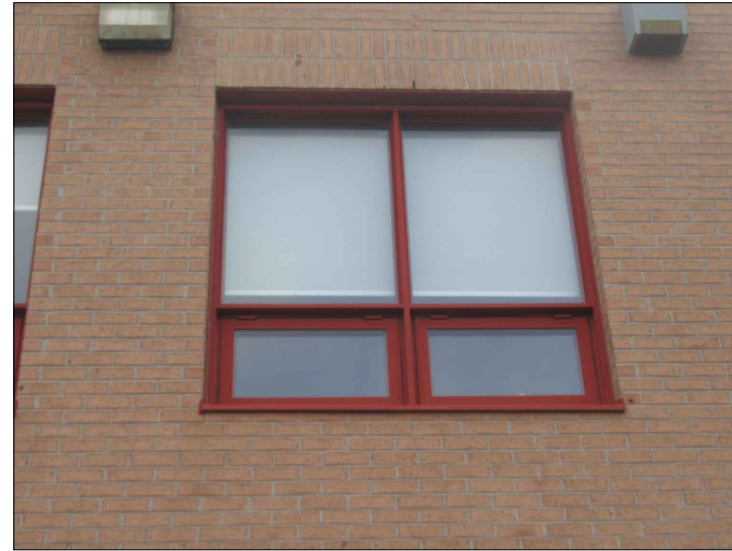
PHOTO 3: VIEW OF EXISTING WINDOW W03
