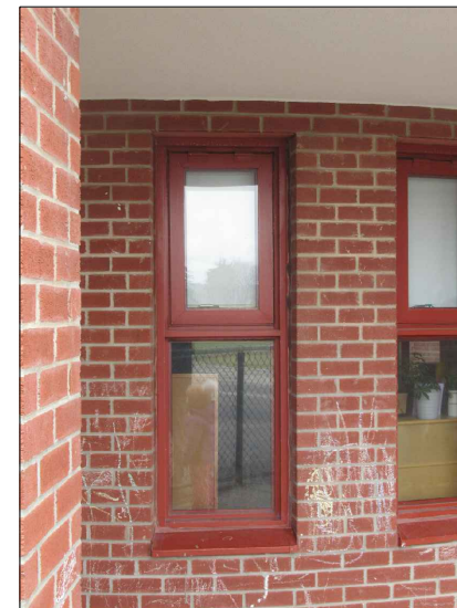
PHOTO 15: VIEW OF EXISTING WINDOW W14
