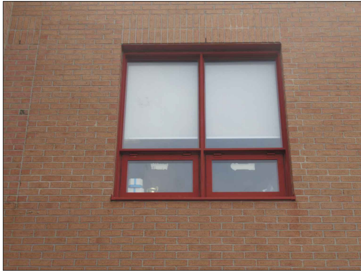
PHOTO 1: VIEW OF EXISTING WINDOW W01
