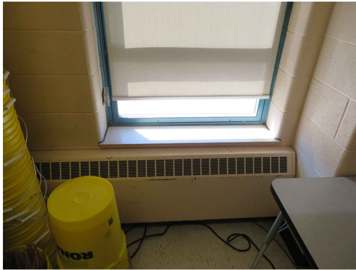
PHOTO 10: TYPICAL VIEW OF EXISTING SILL CONDITIONS.
