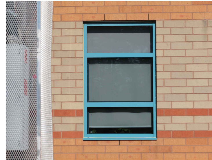
PHOTO 3: VIEW OF EXISTING WINDOW W02
