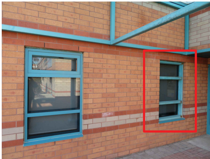
PHOTO 4: VIEW OF EXISTING WINDOW W02A (OUTLINED IN RED)
