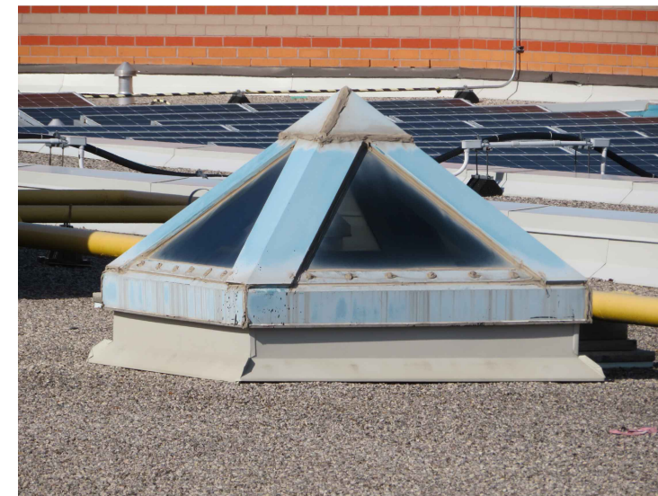
PHOTO 9: TYPICAL VIEW OF EXISTING PYRAMIDAL SKYLIGHT
