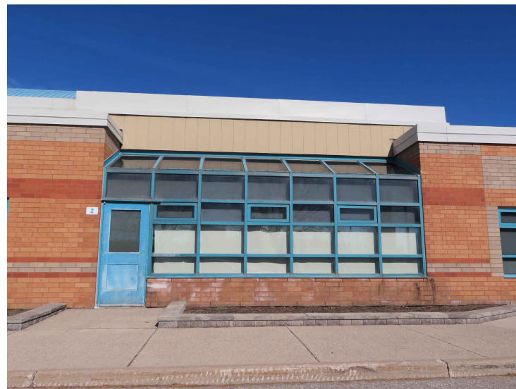
PHOTO 8: VIEW OF EXISTING WINDOW W06 AND DOOR D01
