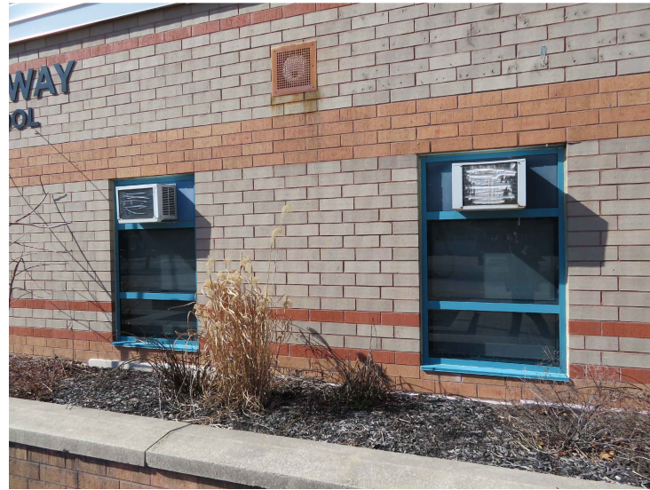
PHOTO 2: VIEW OF EXISTING WINDOW W01A
