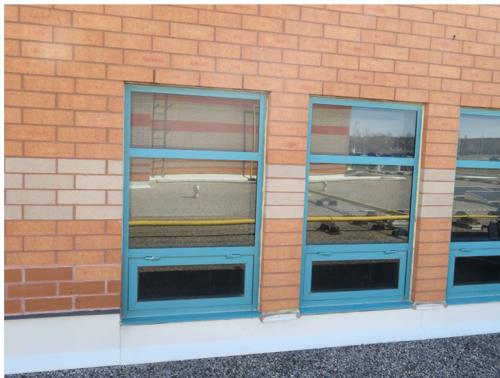
PHOTO 7: VIEW OF EXISTING WINDOW W05
