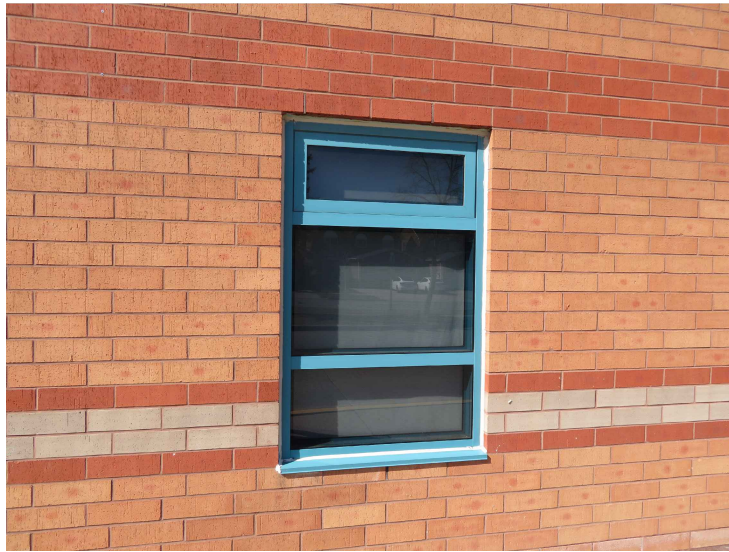
PHOTO 1: VIEW OF EXISTING WINDOW W01
