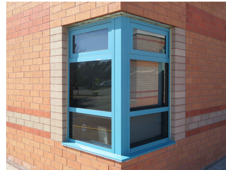
PHOTO 6: VIEW OF EXISTING WINDOW W04
