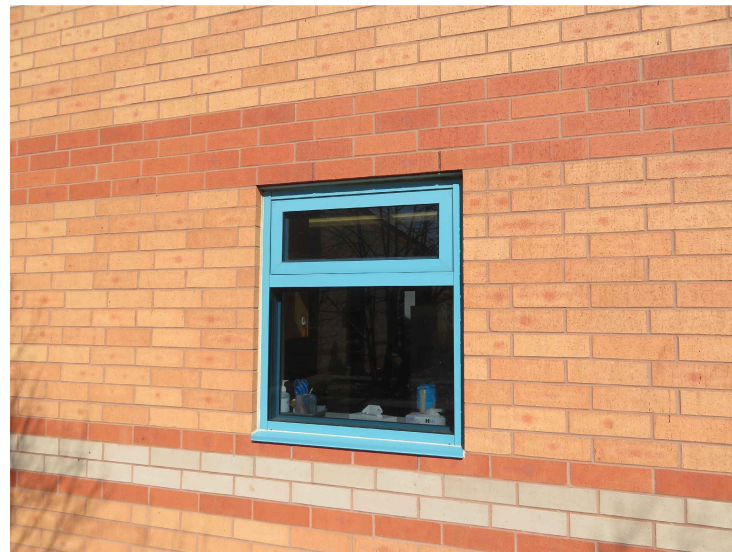
PHOTO 5: VIEW OF EXISTING WINDOW W03
