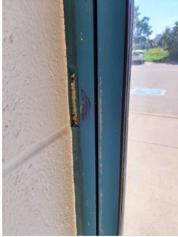
Photograph No. 1 – Green sealant on the interior and exterior perimeter of the windows was sampled and found to be non-asbestos. Sampling also confirmed the sealants as non-PCB.
