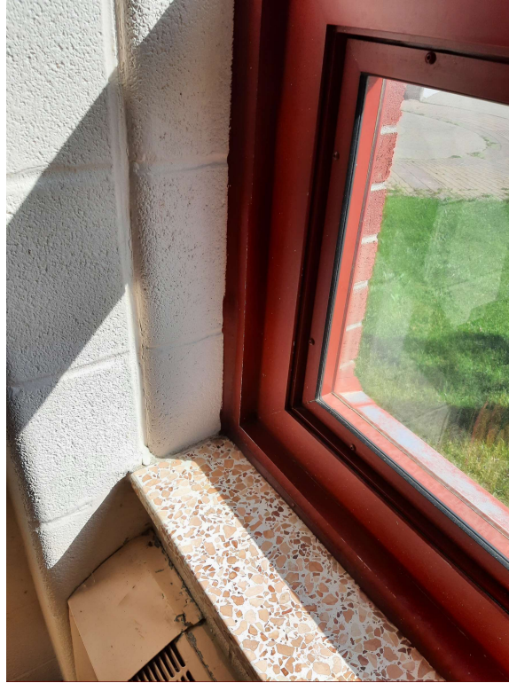
Photograph No. 1 – Red sealant on the interior perimeter of the windows was sampled and found to be non-asbestos. Sampling also confirmed the sealants as non-PCB.
