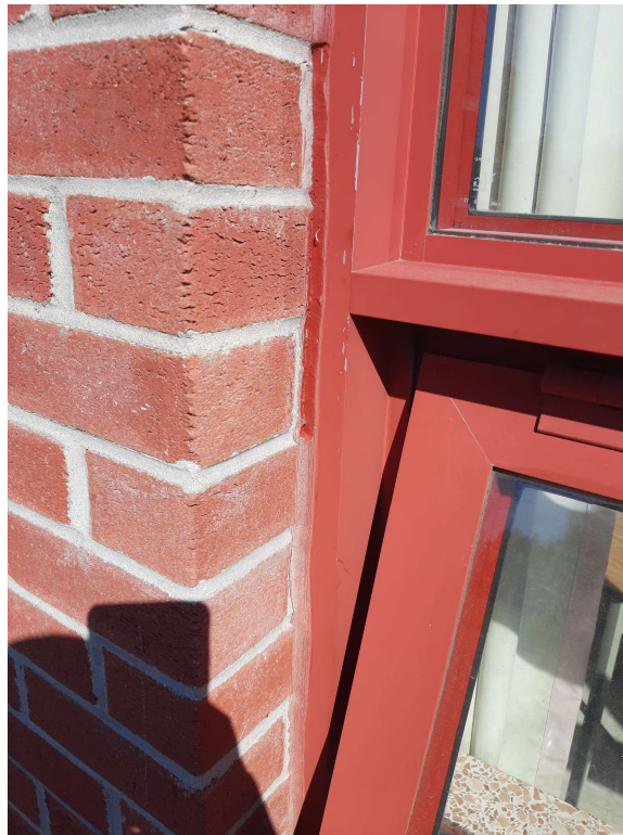
Photograph No. 2 – Red sealant on the exterior perimeter of the windows was sampled and found to be non-asbestos. Sampling also confirmed the sealants as non-PCB.
