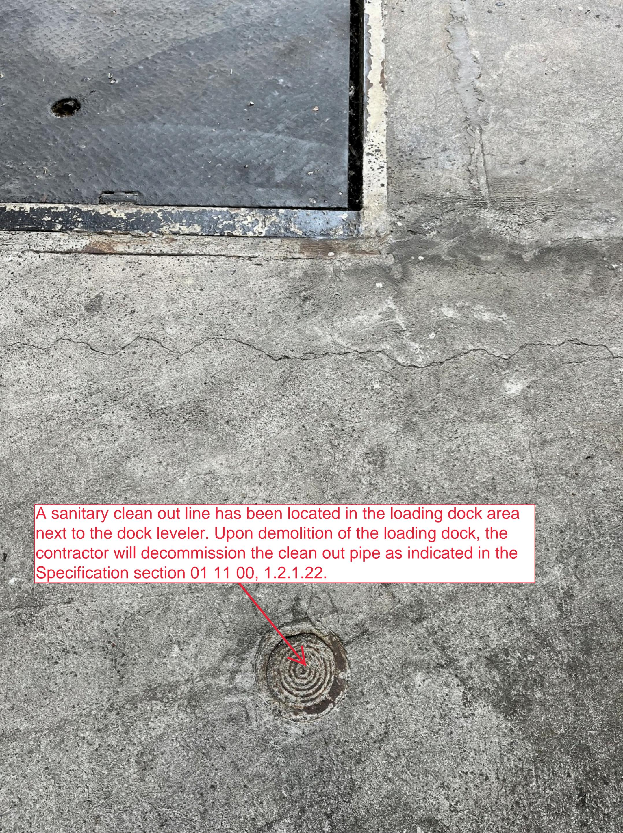
A sanitary clean out line has been located in the loading dock area next to the dock leveler. Upon demolition of the loading dock, the contractor will decommission the clean out pipe as indicated in the Specification section 01 11 00, 1.2.1.22.
