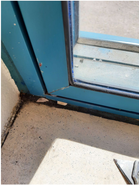
Photograph No. 2 – Black sealant on the interior side of the window was sampled and found to be non-asbestos and non-PCB.
