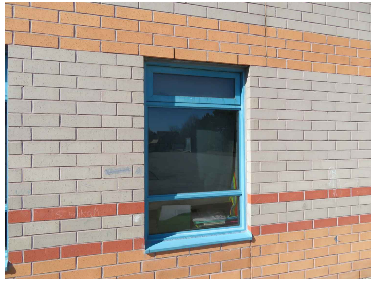
PHOTO 2: VIEW OF EXISTING WINDOW W01A
