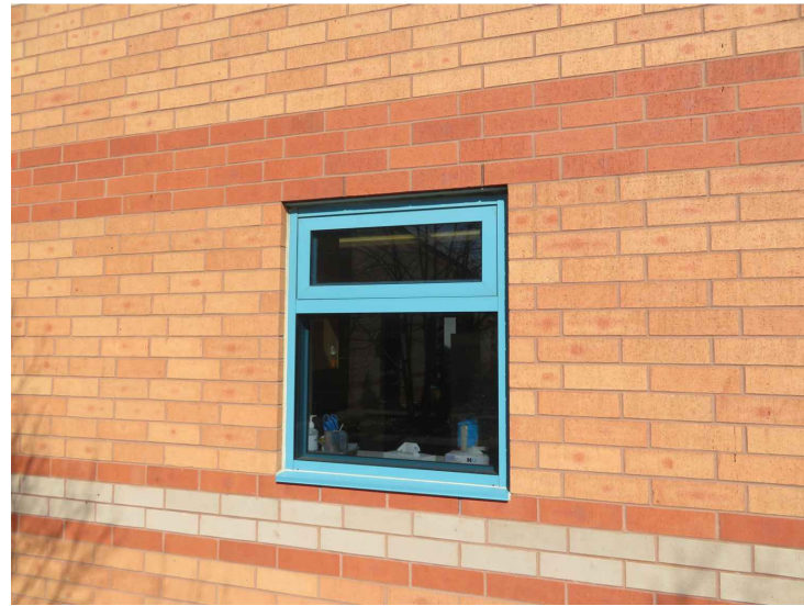
PHOTO 5: VIEW OF EXISTING WINDOW W03
