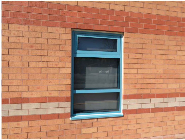
PHOTO 1: VIEW OF EXISTING WINDOW W01
