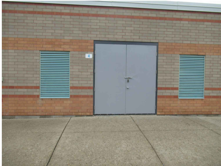
PHOTO 16: VIEW OF LOUVERS/VENTS FOR PERIMETER CAULKING REPLACEMENT.
