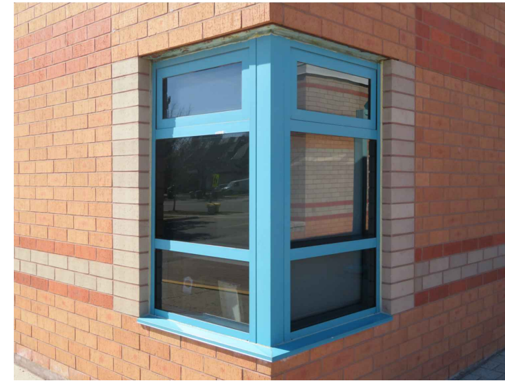
PHOTO 6: VIEW OF EXISTING WINDOW W04
