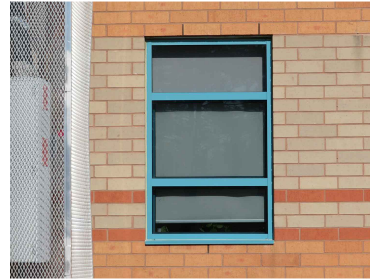
PHOTO 3: VIEW OF EXISTING WINDOW W02
