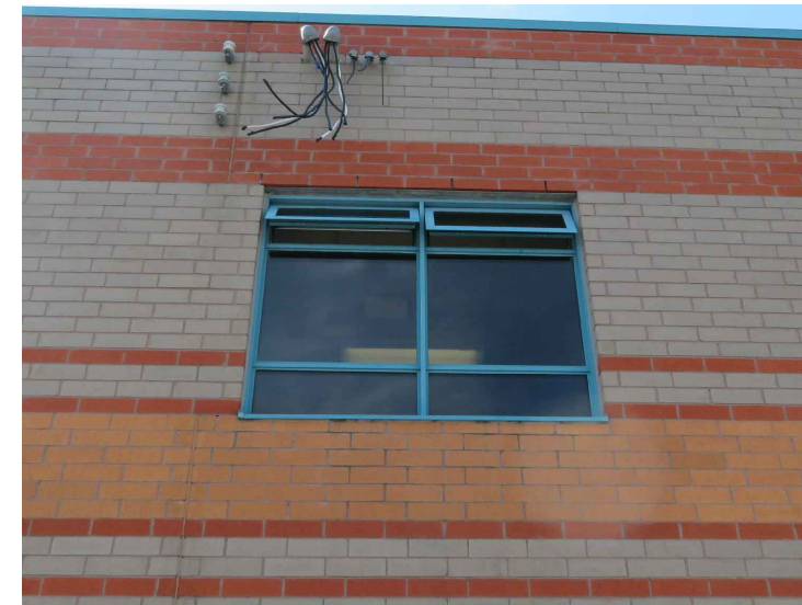
PHOTO 9: VIEW OF EXISTING WINDOW W07
