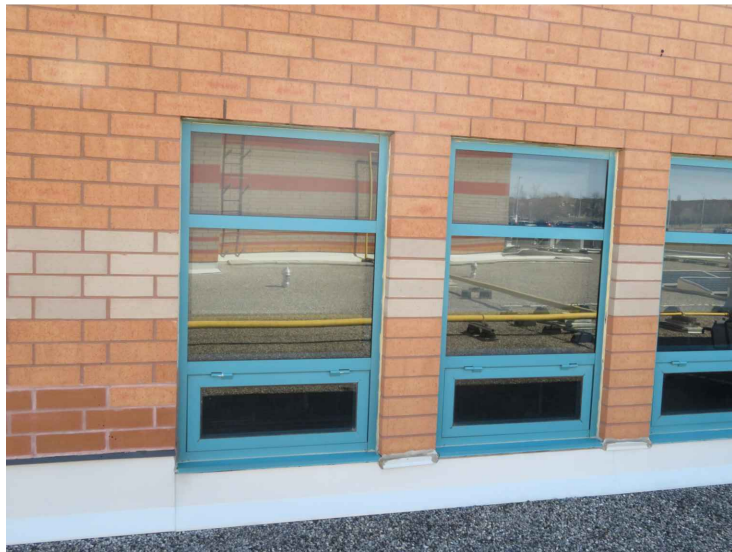
PHOTO 7: VIEW OF EXISTING WINDOW W05
