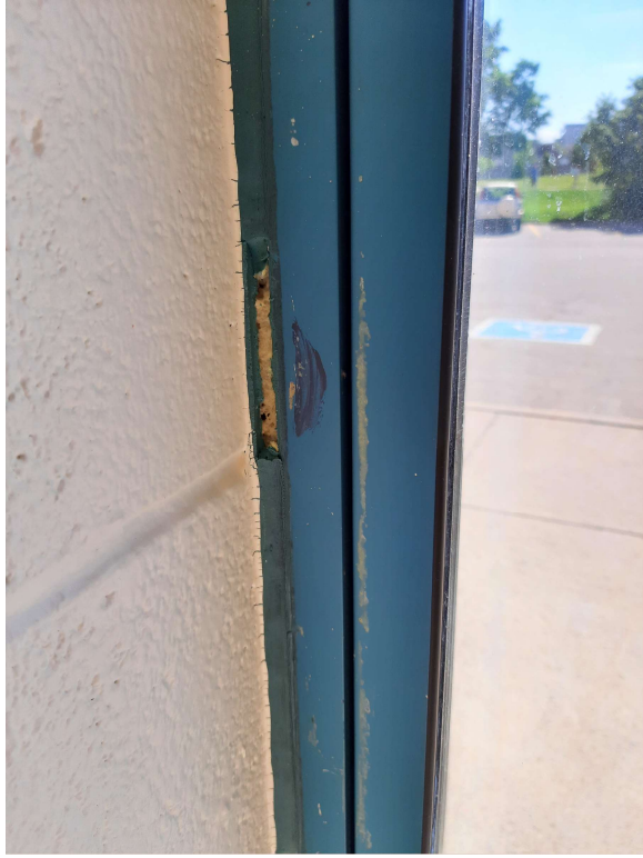
Photograph No. 1 – Green sealant on the interior and exterior perimeter of the windows was sampled and found to be non-asbestos. Sampling also confirmed the sealants as non-PCB.
