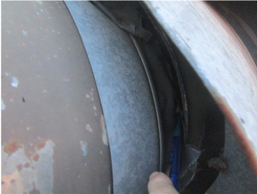
Close-up of the open and deteriorated flex connection at the fan unit.
