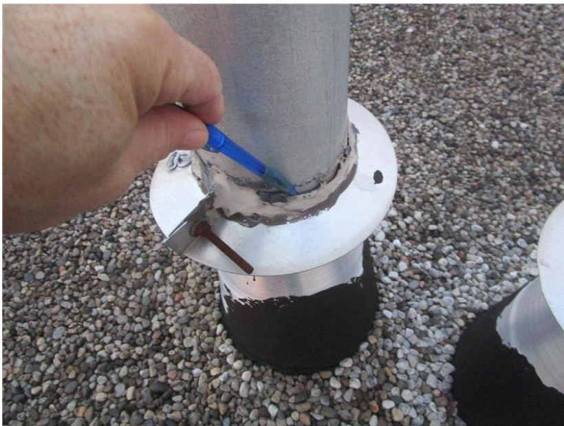
The sealant used to seal this furnace stack rain collar is open and deteriorated. This condition may be allowing water to enter the roofing assembly and/or building.
