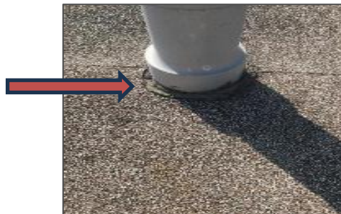
Caulking, South roof section.
