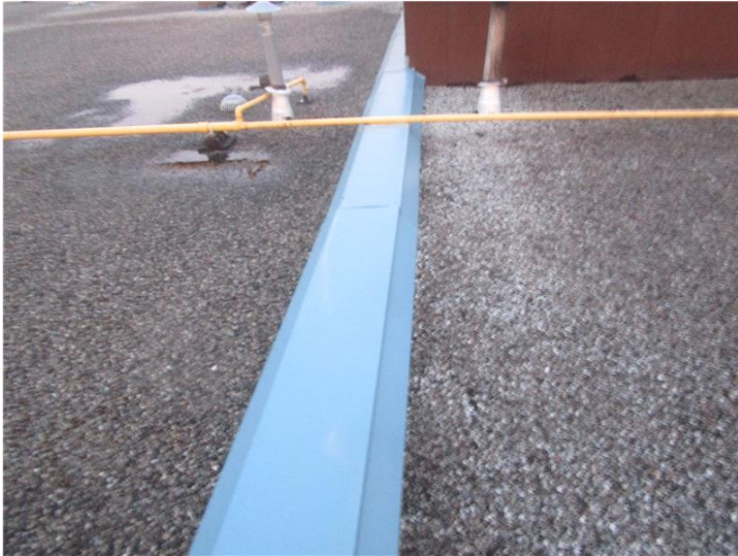
View of the expansion joint.
