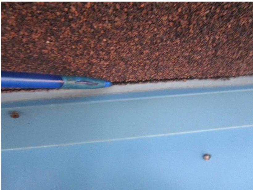
More open sealant at the perimeter metal flashings.
