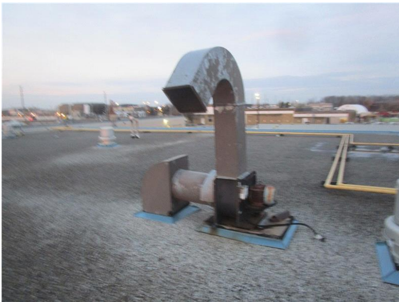
Open and deteriorated flex connection was noted at the fan unit.
