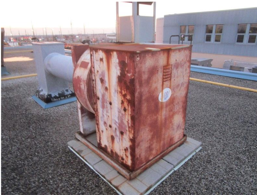
View of the corroded fan unit.
