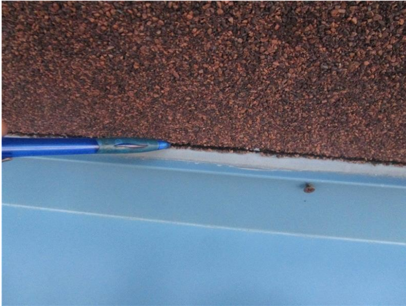
Close-up of the open sealant at the perimeter metal flashings.
