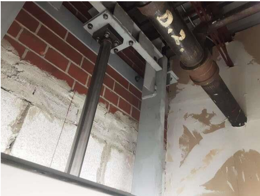
V0034 (None), Wall, Mortar, Elevator Pit (Location #: 50).
