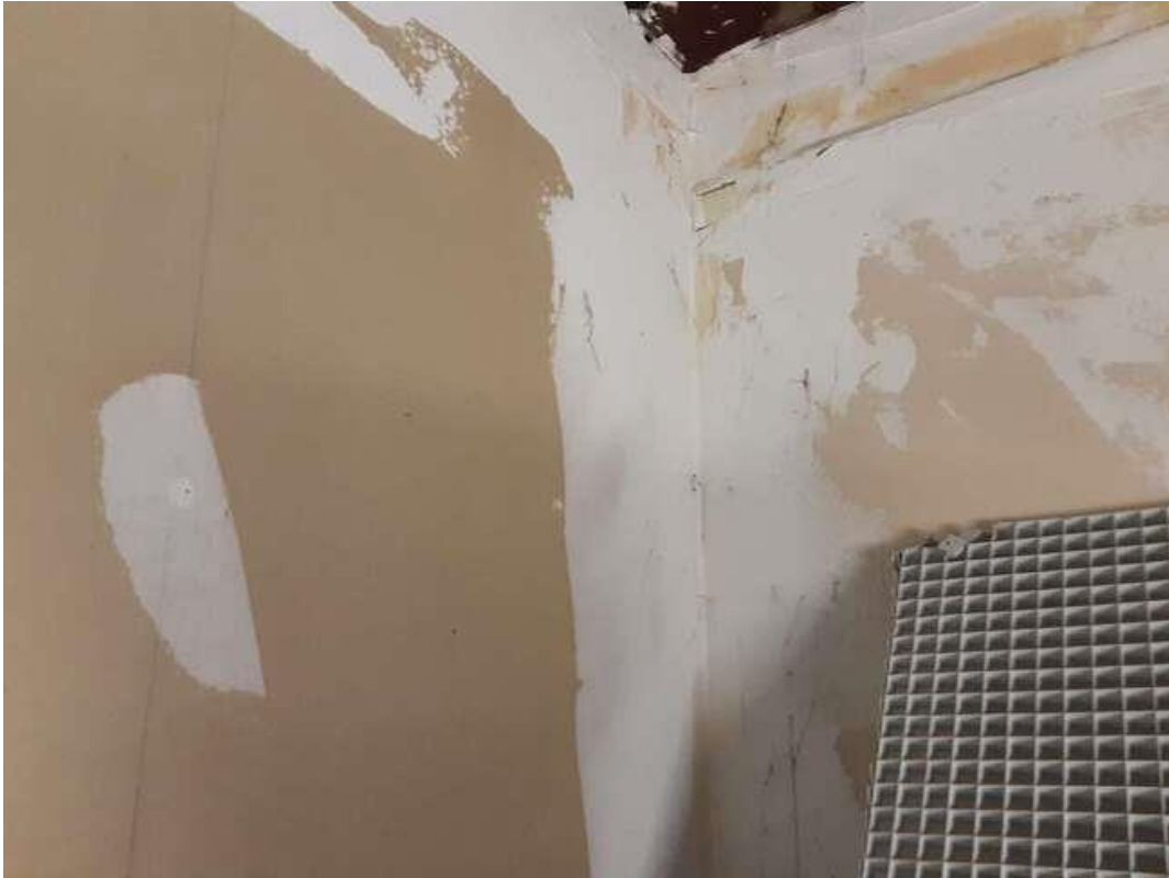
S0033A (None), Wall, Drywall and joint compound, Elevator Pit (Location #: 50).
