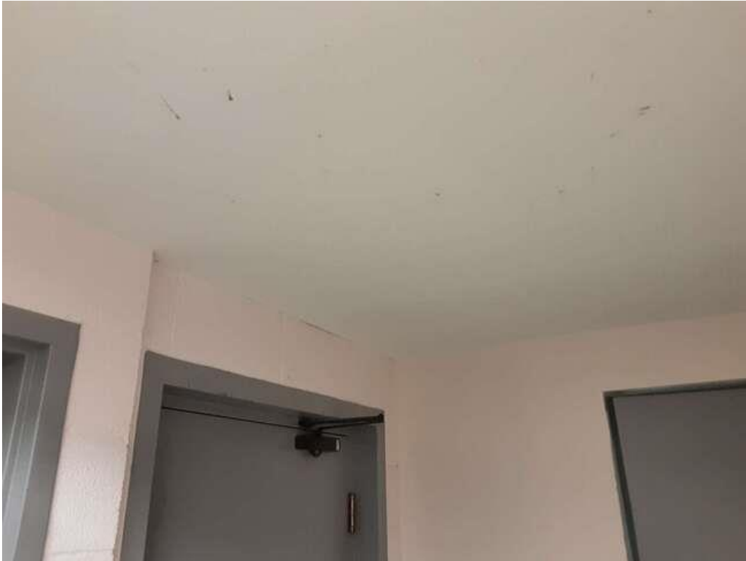
S0031A (None), Ceiling, All, Drywall and joint compound, Corridor Men's (Location #: 47).
