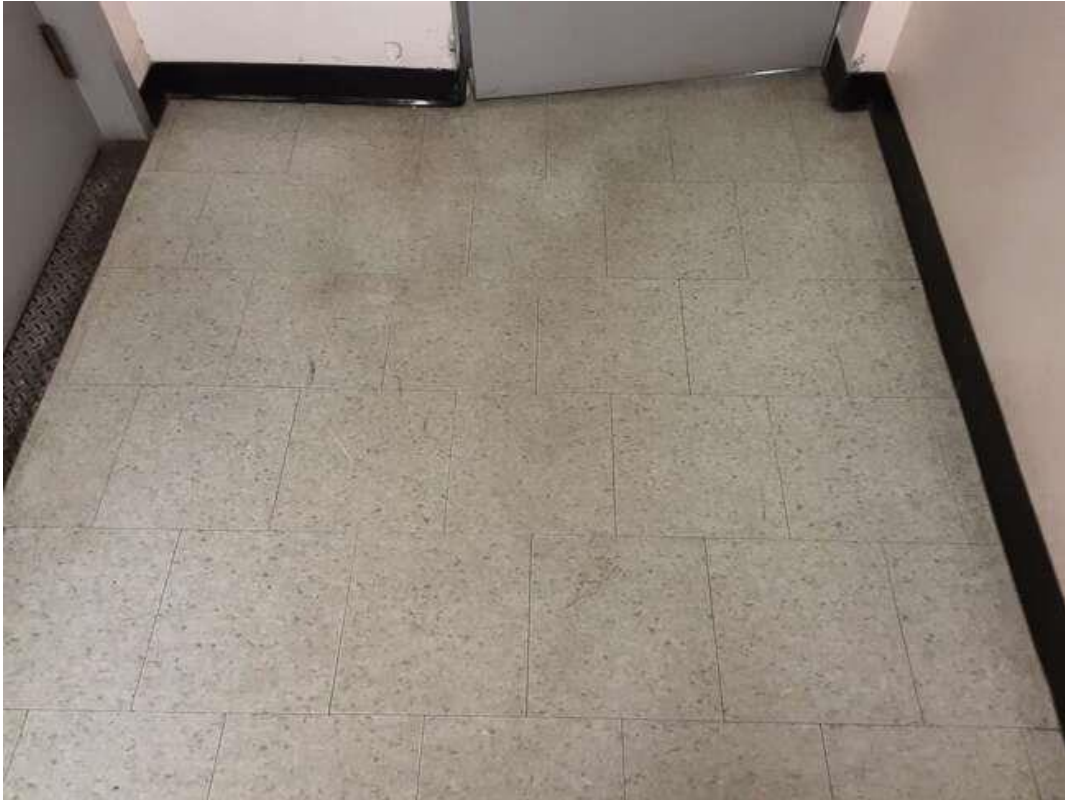
V0018 (None), 12 x 12 green with dark green flecks, Floor, All, Vinyl Floor Tile and Mastic, Corridor Men's (Location #: 47).
