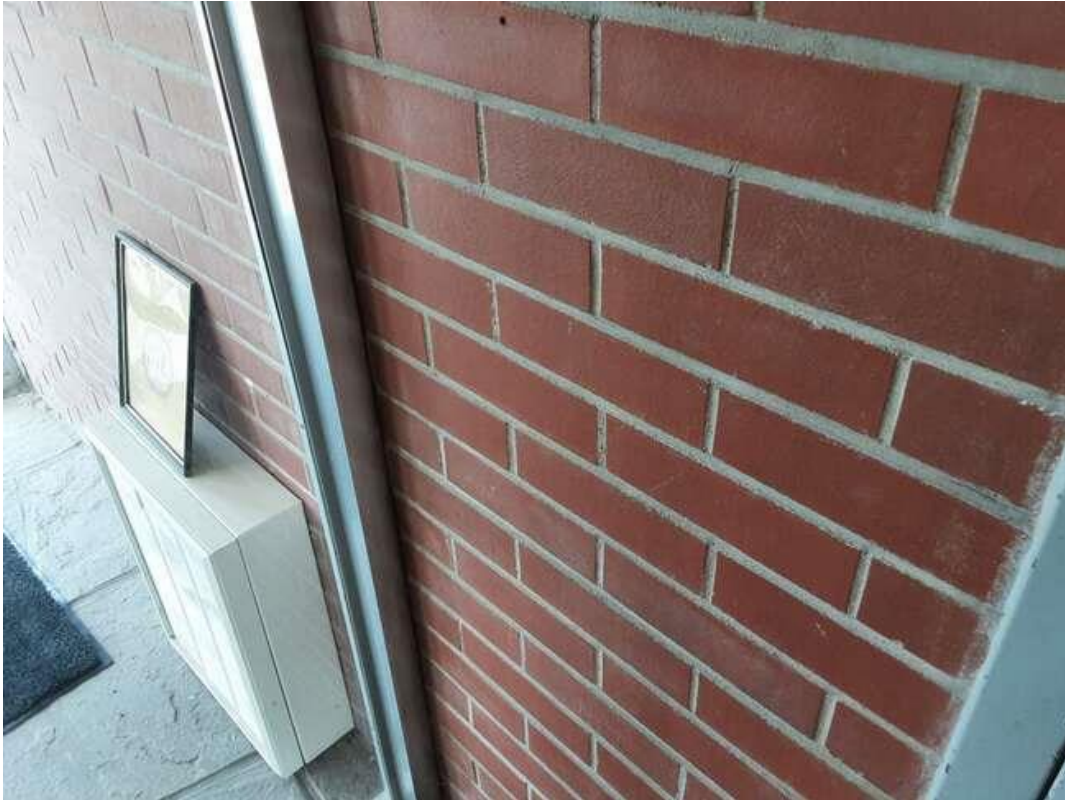
S0034A (None), Wall, Mortar, Entrance Vestibule (Location #: 48).
