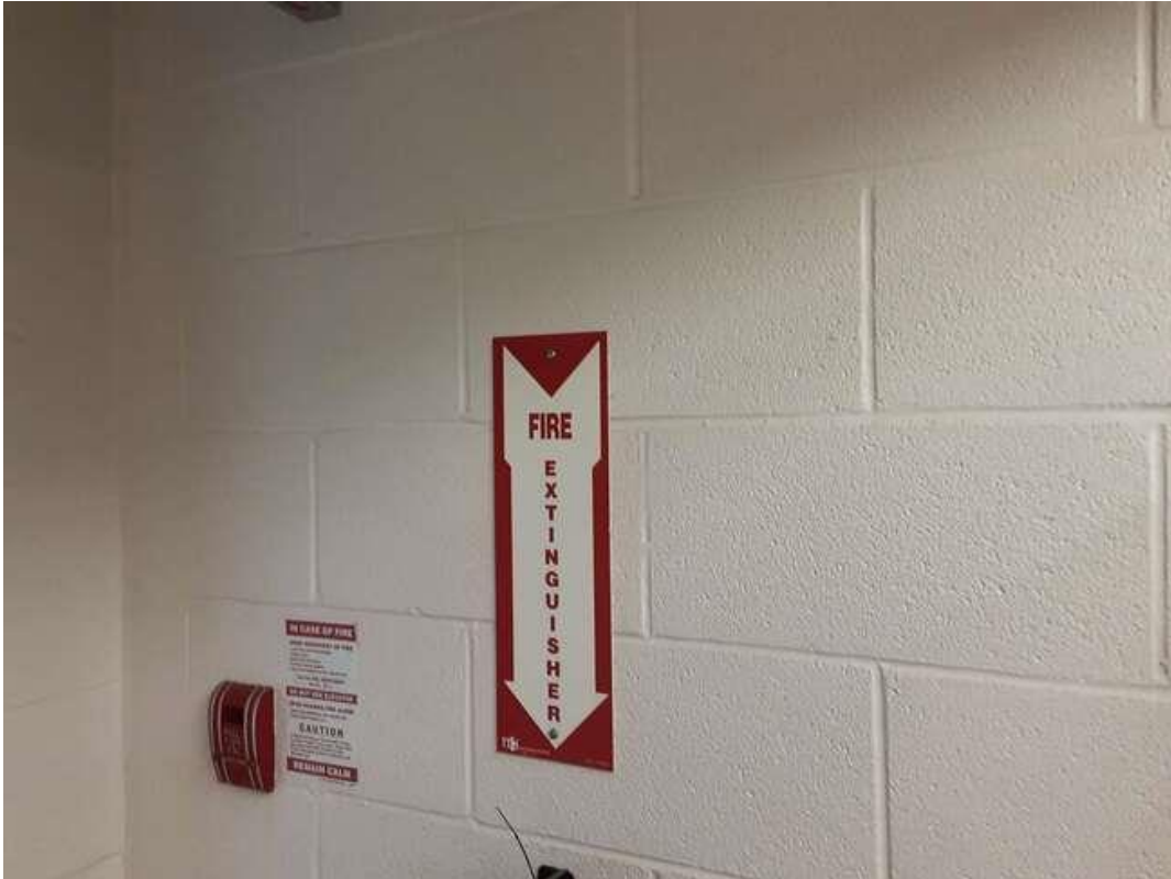
V0000 (None), Block wall, Wall, Masonry, Corridor Men's (Location #: 47).
