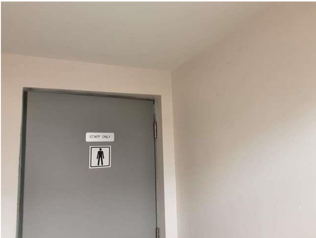
S0030A (None), Wall, Drywall and joint compound, Corridor Men's (Location #: 47).
