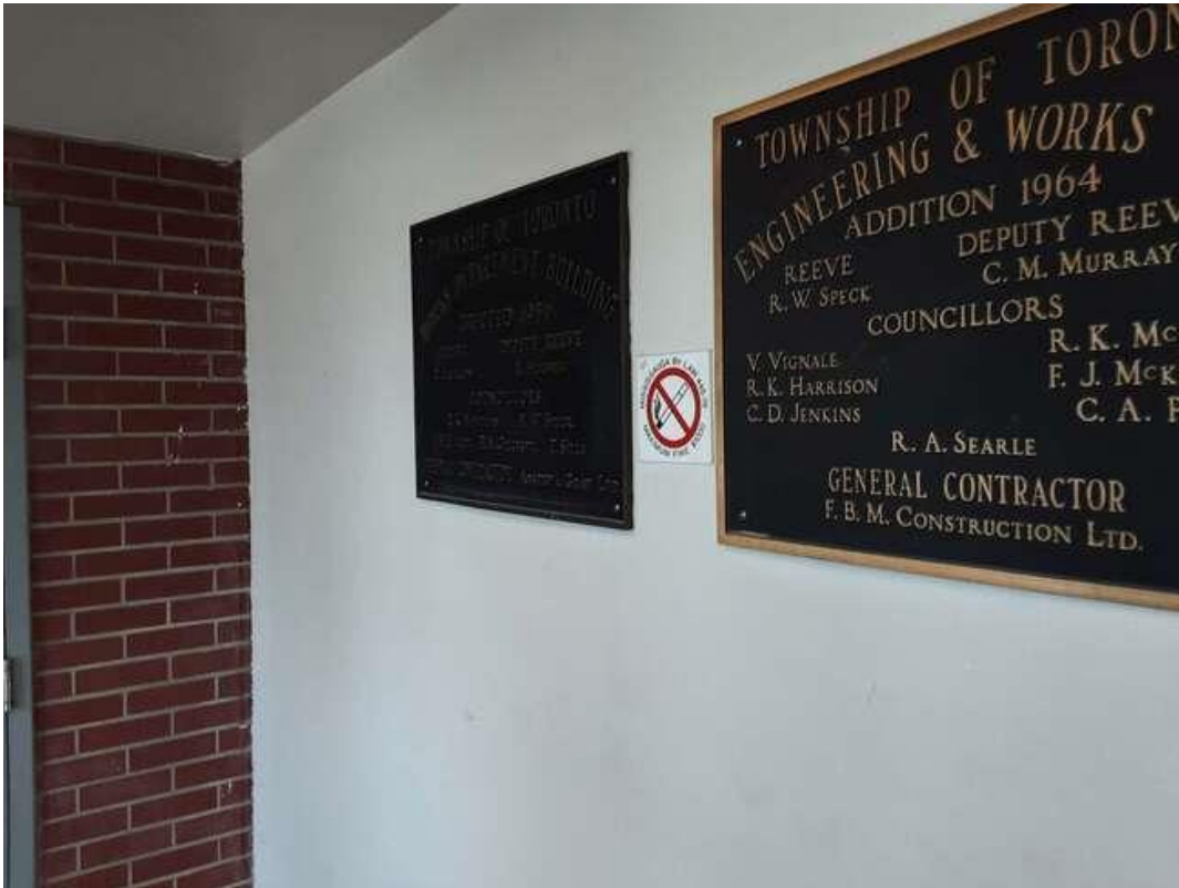
V0013(Lead, None), White, Wall, Entrance Vestibule (Location #: 48).
