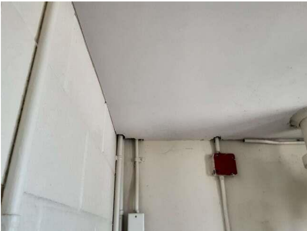
S0031B (None), Ceiling, All, Drywall and joint compound, Sprinkler Room (Location #: 49).
