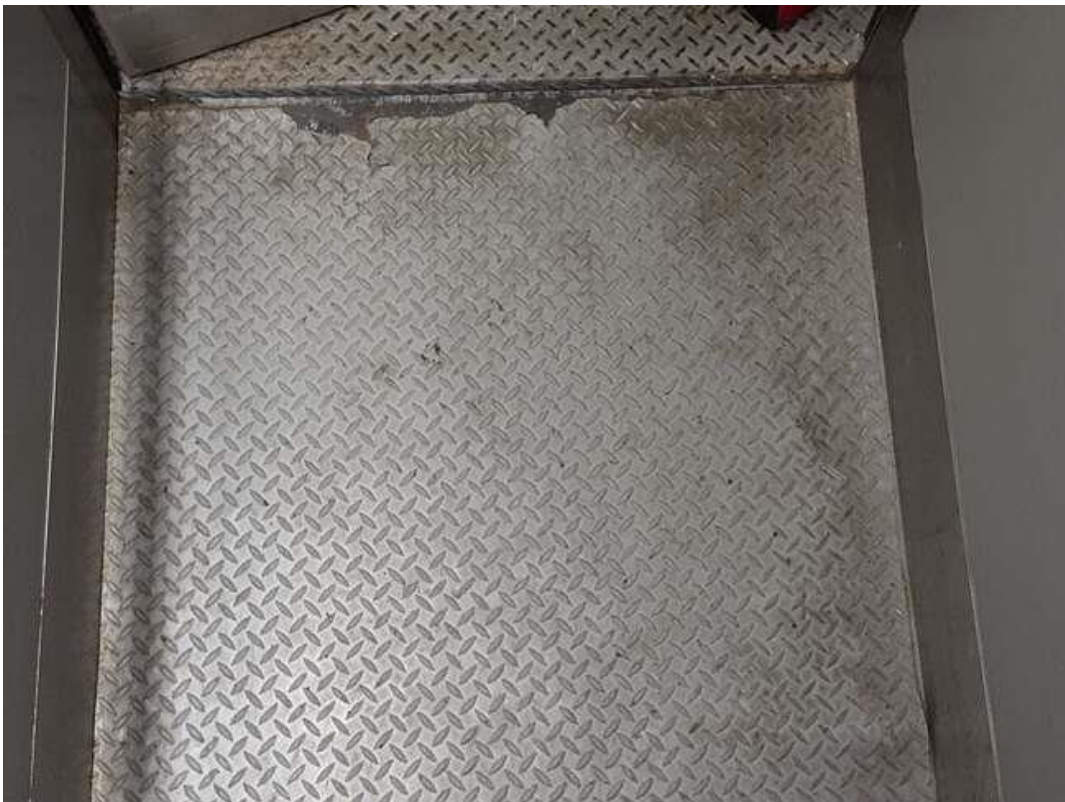
V0000 (None), Floor, Metal, Elevator Pit (Location #: 50). Elevator floor
