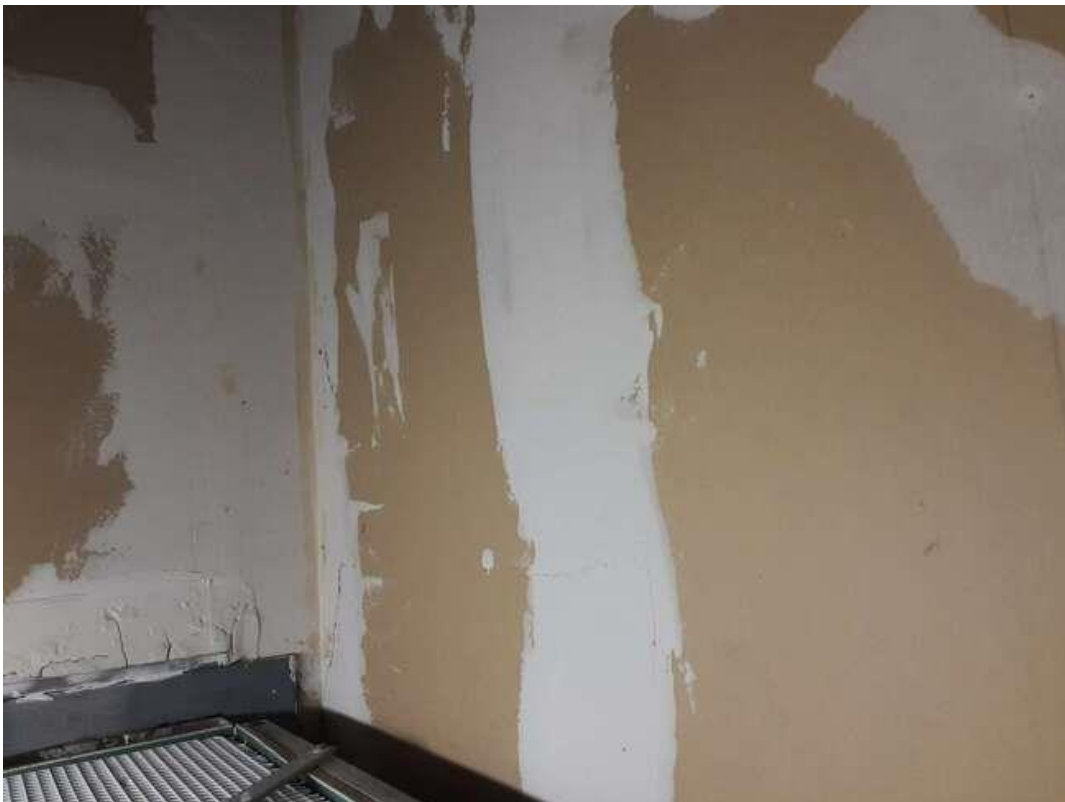
S0033C (None), Wall, Drywall and joint compound, Elevator Pit (Location #: 50).
