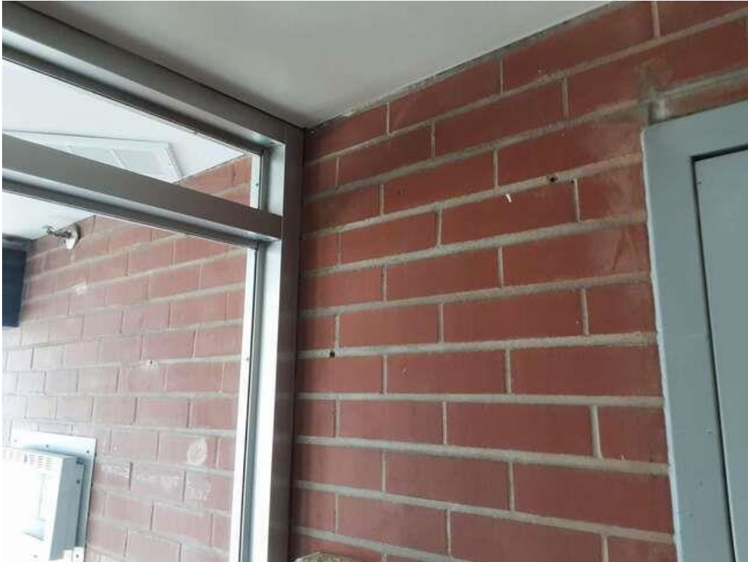
V0000 (None), Brick wall, Wall, Masonry, Entrance Vestibule (Location #: 48).
