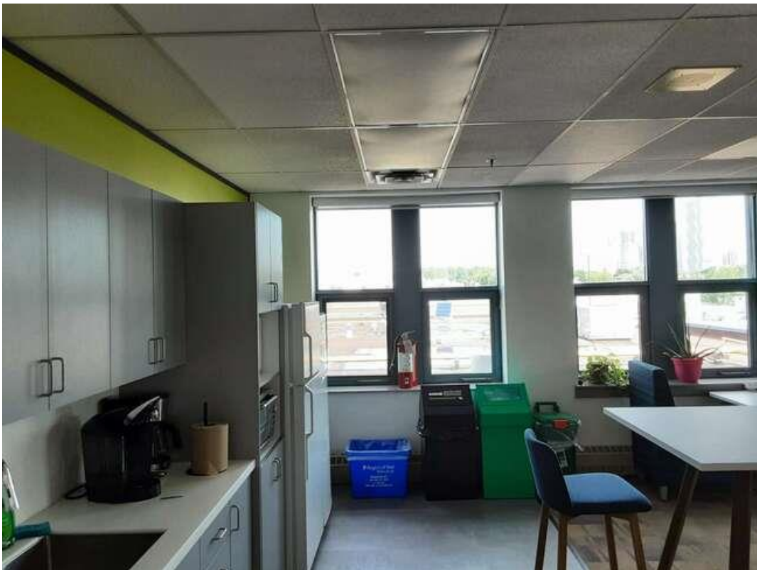
S0021A (None), Perimeter wall, Wall, Drywall and joint compound, Open Office Area (Location #: 27).
