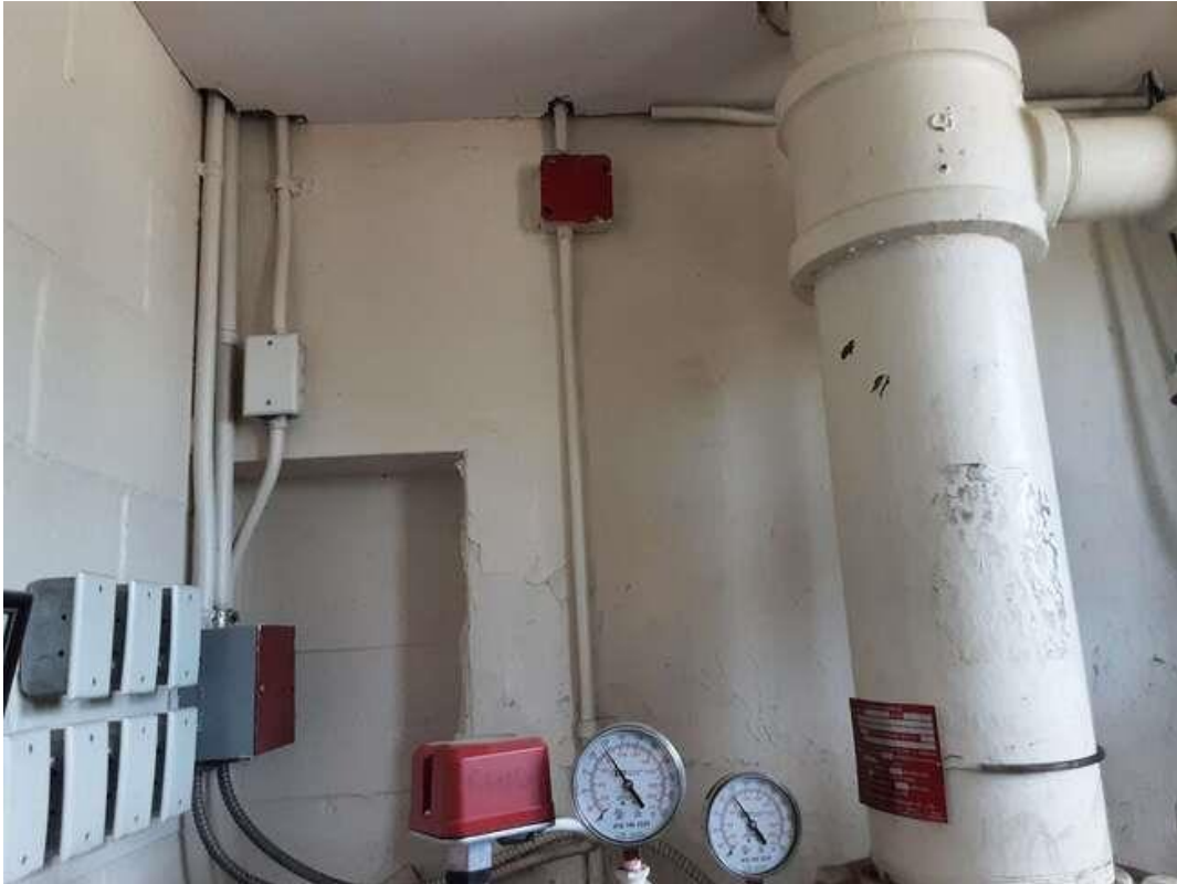
V0000 (None), Wall, Concrete (poured), Sprinkler Room (Location #: 49). Behind sprinkler
