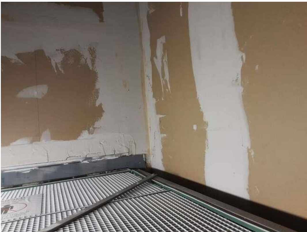
Elevator Pit (Location #: 50).
