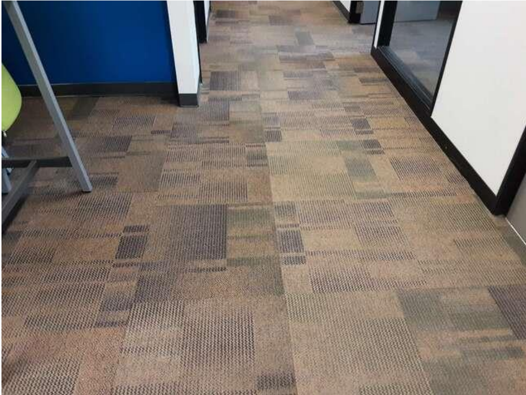
V0000 (None), Floor, Carpet, Open Office Area (Location #: 27).
