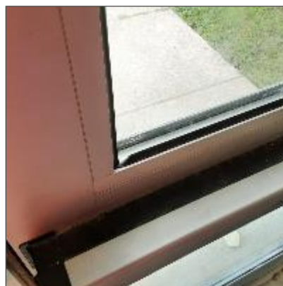
Non-PCB black butyl sealant, Entrance Vestibule (Loc. 48).
