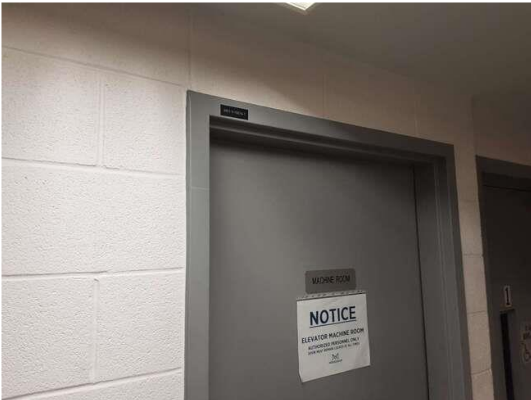
V0017 (None), Block wall, Wall, Mortar, Corridor Men's (Location #: 47).
