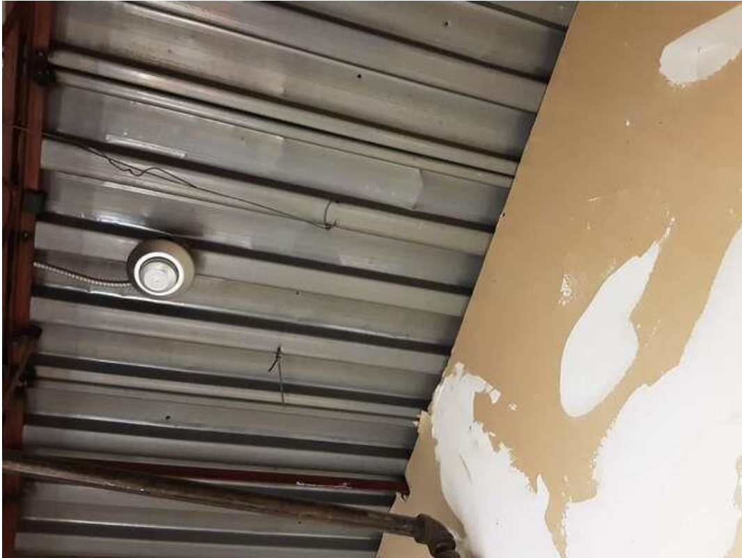
V0000 (None), Structure, All, Metal, Elevator Pit (Location #: 50).
