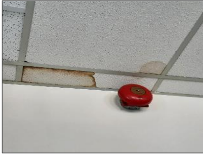
Water-stained acoustic ceiling tiles in the Office (Location 5).
