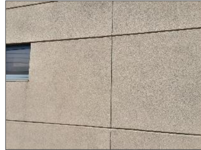
Non-asbestos stucco exterior cladding (Location 41).
