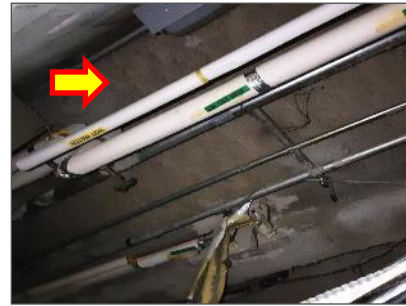
Non-asbestos fireproofing on structure in the Reception and Corridor (Location 1).
