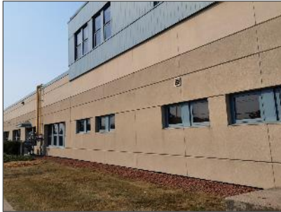
Non-asbestos stucco exterior cladding (Location 41).
