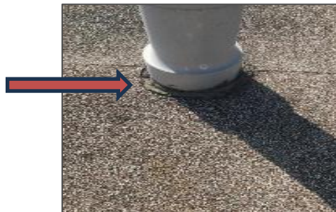
Caulking, South roof section.
