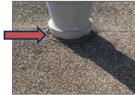
Caulking, south roof section.
