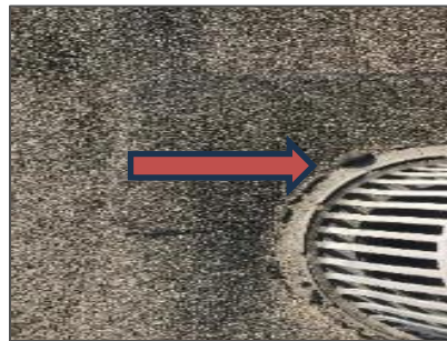
Tar, south roof section.
