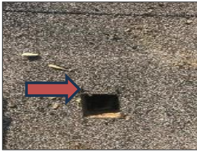
Built-up roof materials, south roof section.
