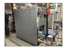
Uninsulated boiler – Boiler Room (Location B-014).
