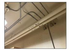
Pipes insulated with fibreglass and jacketed in paper— Cleaner Storage (Location B-004).
