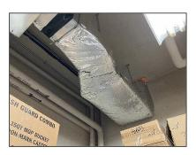
Duct insulated with fibreglass and jacketed in foil – Central Files Storage (Location B-007).
