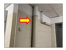
Presumed asbestos-containing Transite pipe – Corridor (Location 1-098).
