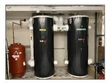
Hot water tanks insulated with fibreglass – Storage Cages (Location B-002).
