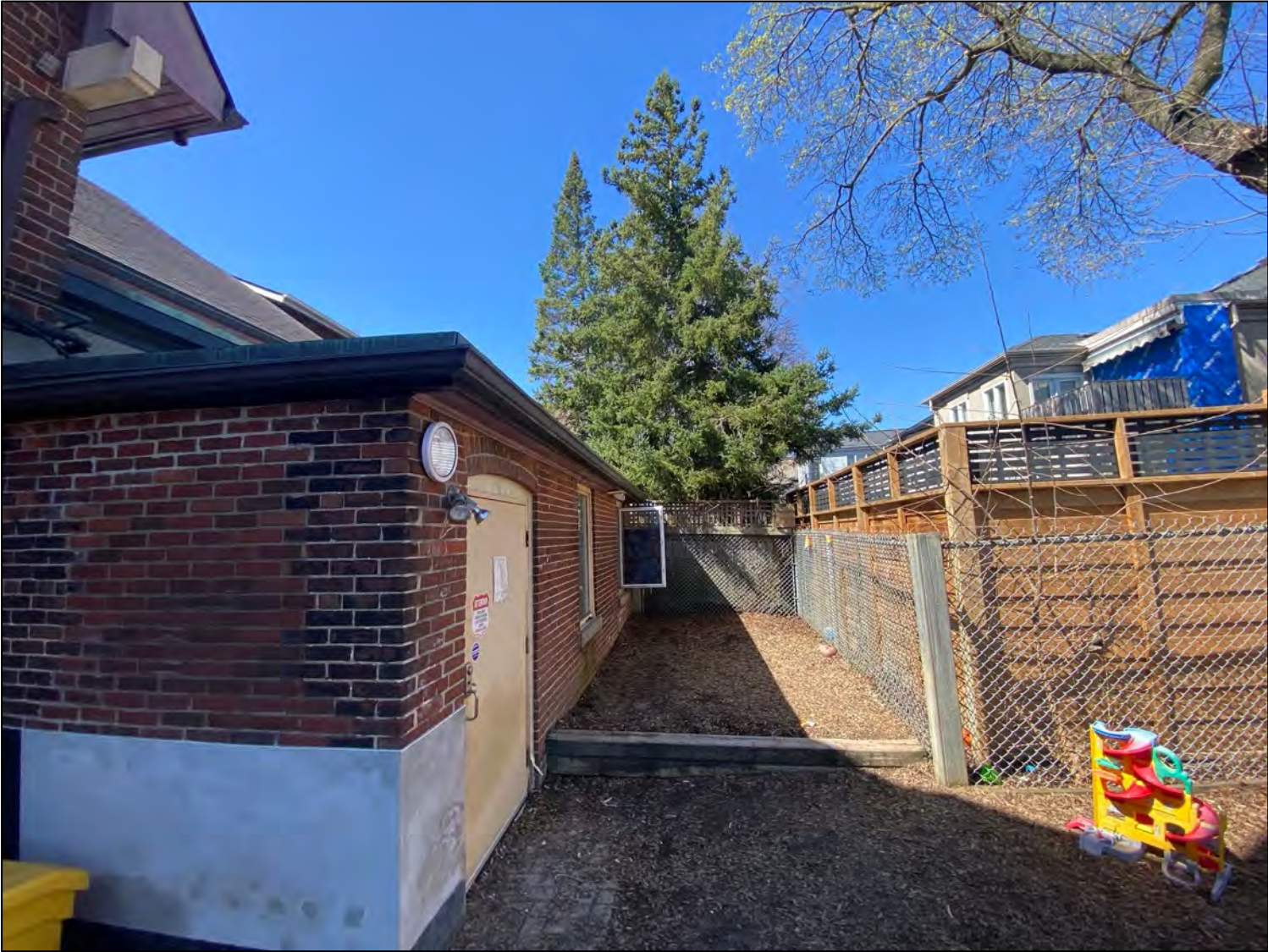
Existing conditions within daycare.
