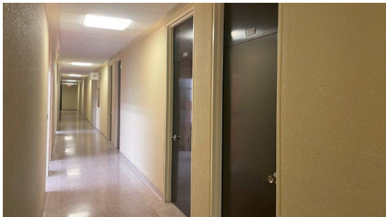
Photo 1: Entrances to office spaces, first floor corridor.
