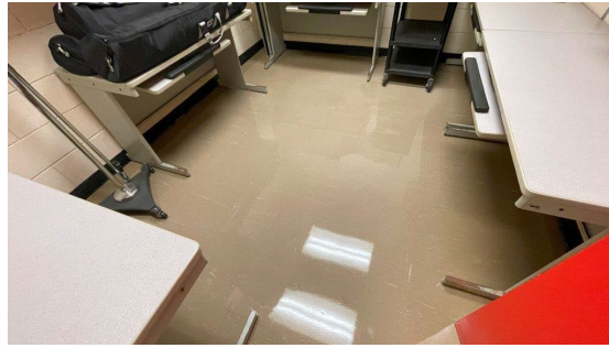
Photo 4: Typical finishes within second floor offices (Room #2024).
