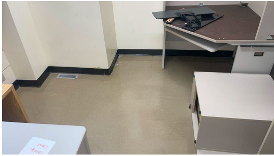
Photo 3: Typical finishes within first floor offices (Room #1033).
