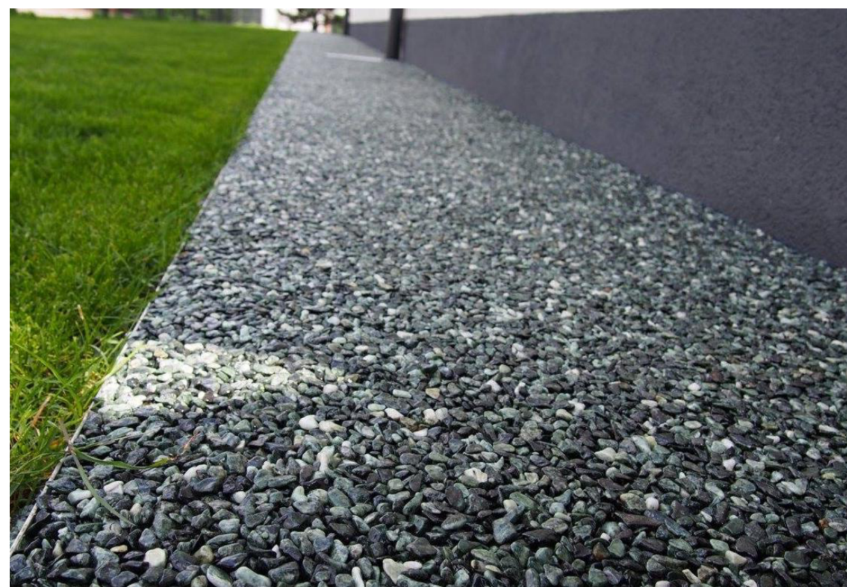
PH.1 PERMEABLE GRAVEL BINDING FOR KENNEL PAVING ALONG PERIMETER
