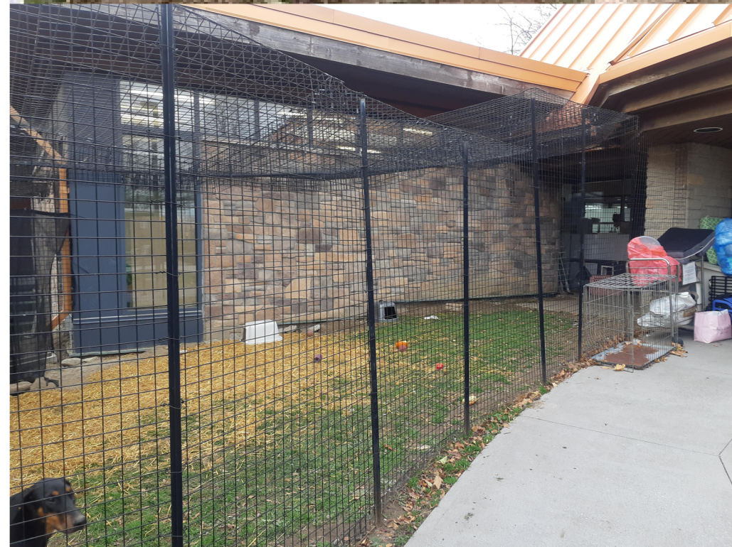
PH.5 EXISTING ENCLOSURE TO BE DEMOLISHED AND REPLACED
