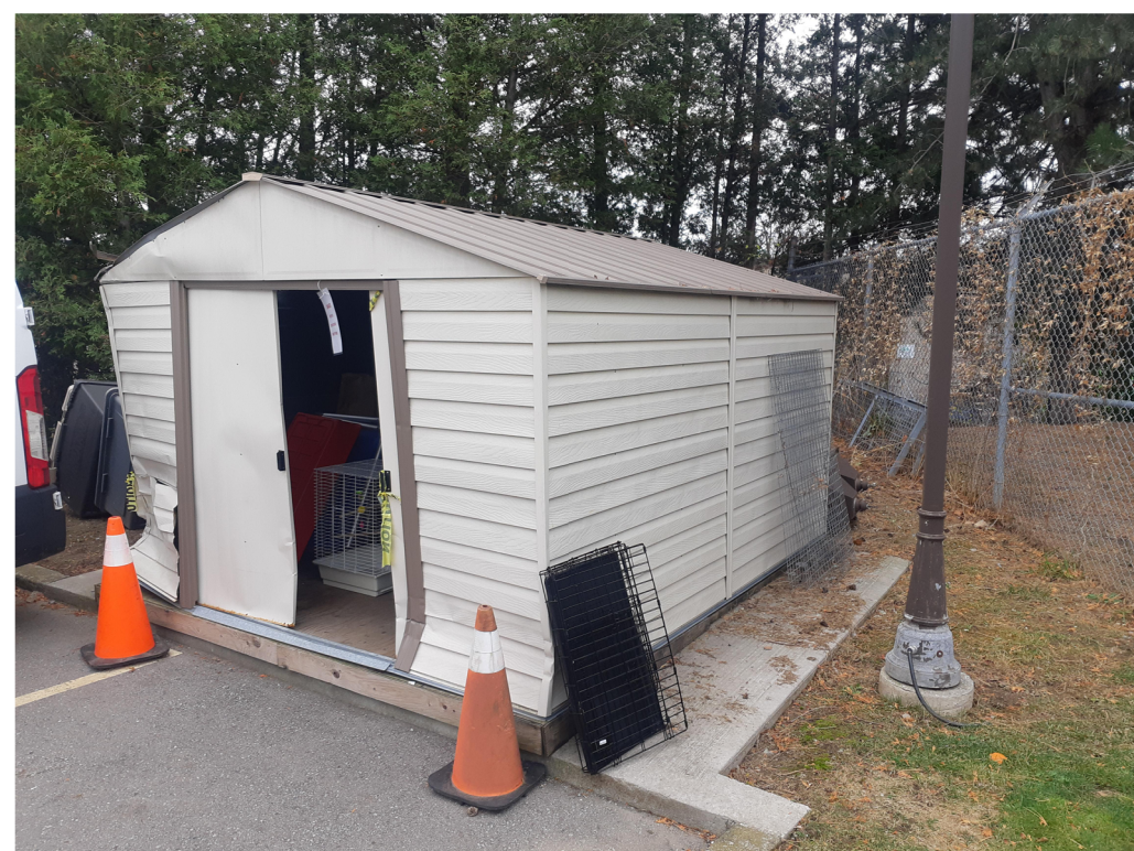
PH.6 EXISTING SHED AND CONC. PAD TO BE DEMOLISHED AND REPLACED
