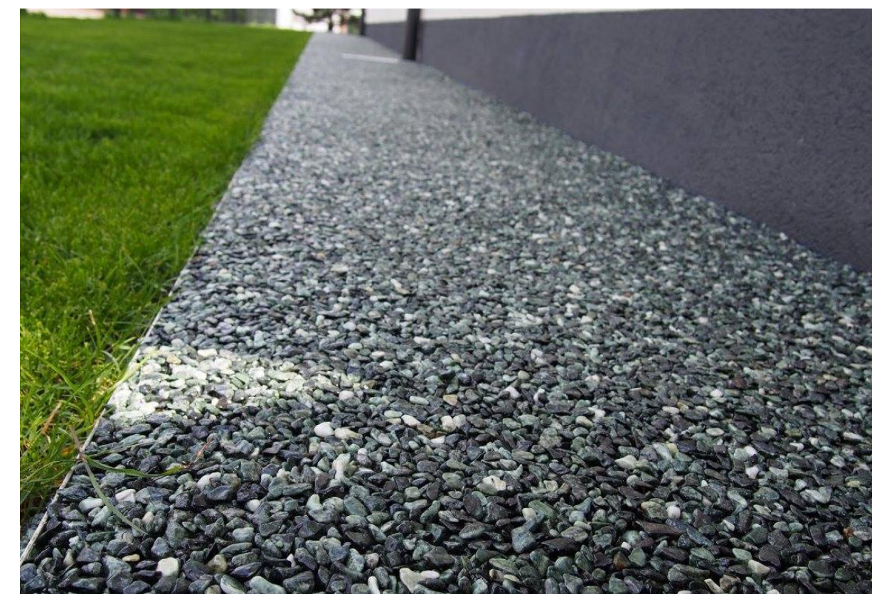
PH.1. PERMEABLE GRAVEL BINDING FOR KENNEL PAVING ALONG PERIMETER
