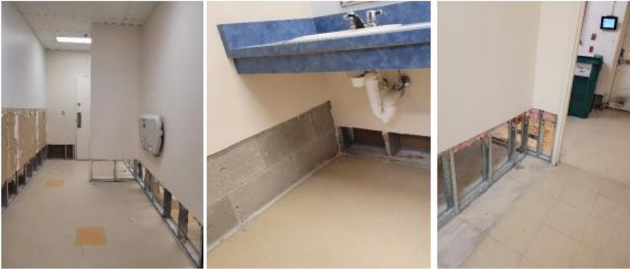
New drywall work required, typ.
