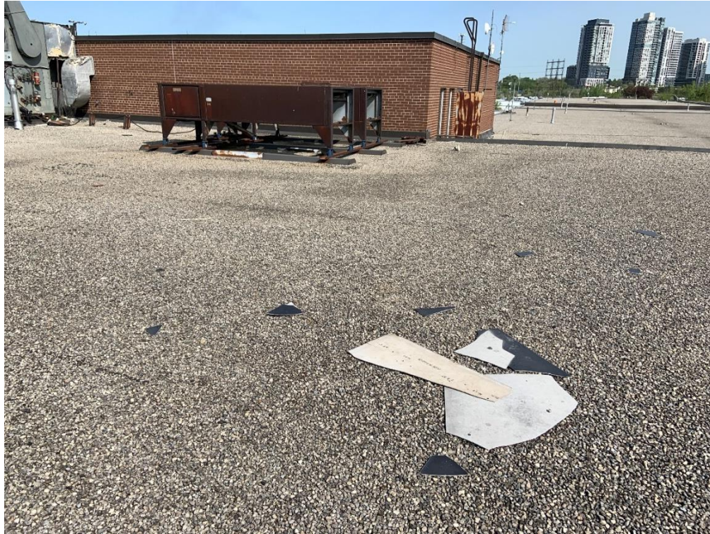
Photo 3: Pieces of damaged Transite Board observed on the roof.
