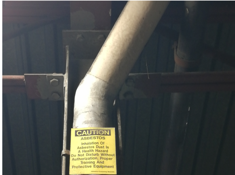
Rain leader in north warehouse with parging cement fitting
