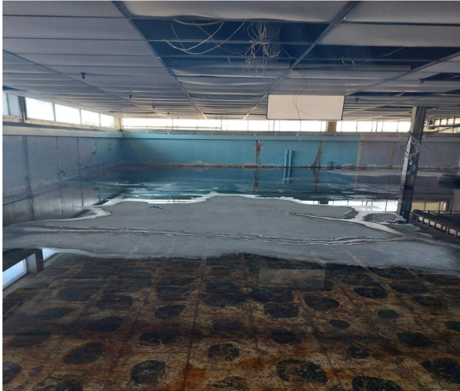
Photograph 9: View of the pooled water in the basement of the two-storey office building.
