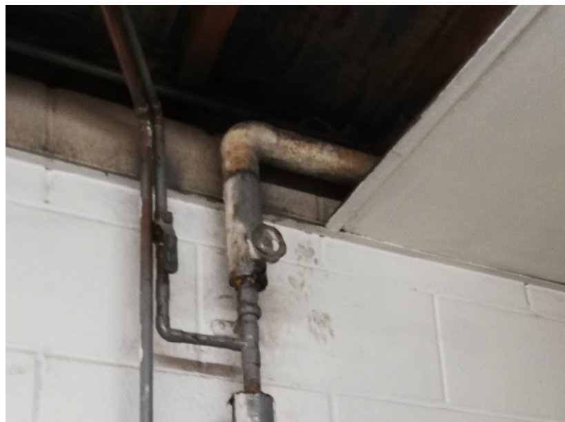
Water lines in the washrooms with parging cement fitting
