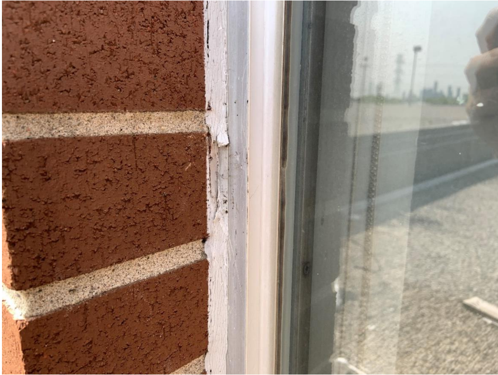
Photo 5: View of the asbestos-containing white caulking around the exterior of the windows and door frames.
