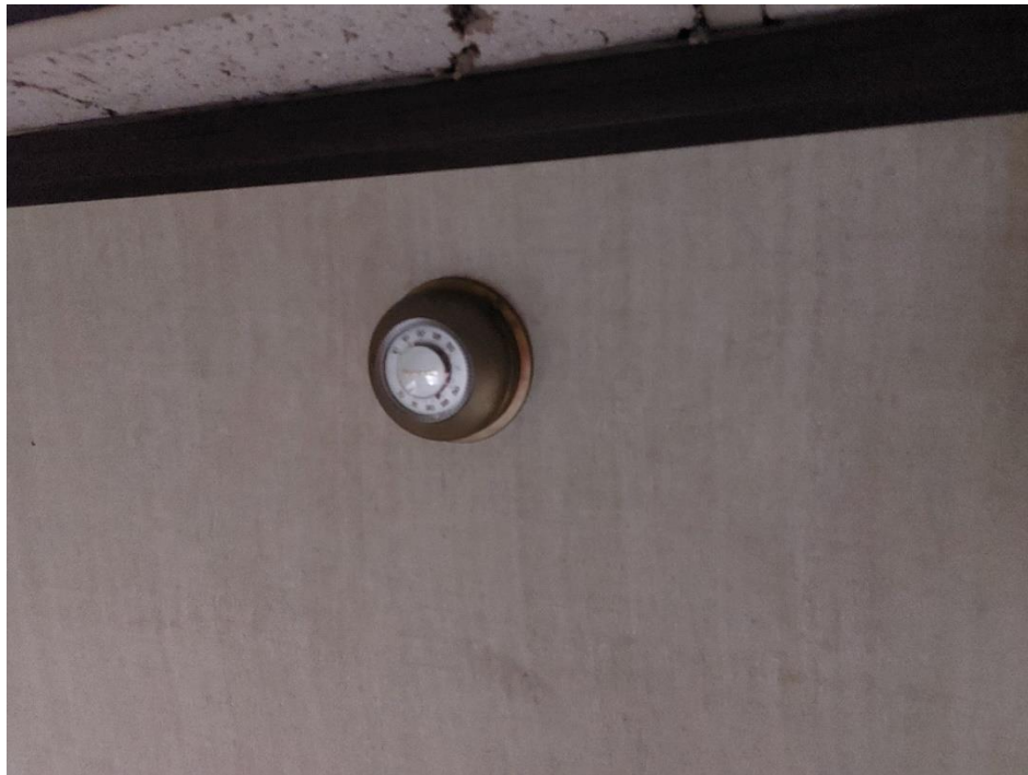
Photograph 10: View of a mercury-containing thermostat in the two-storey office building.
