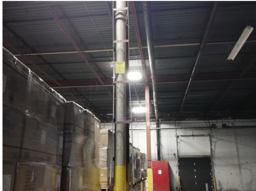
Transite Pipe Rain leader in south warehouse area
