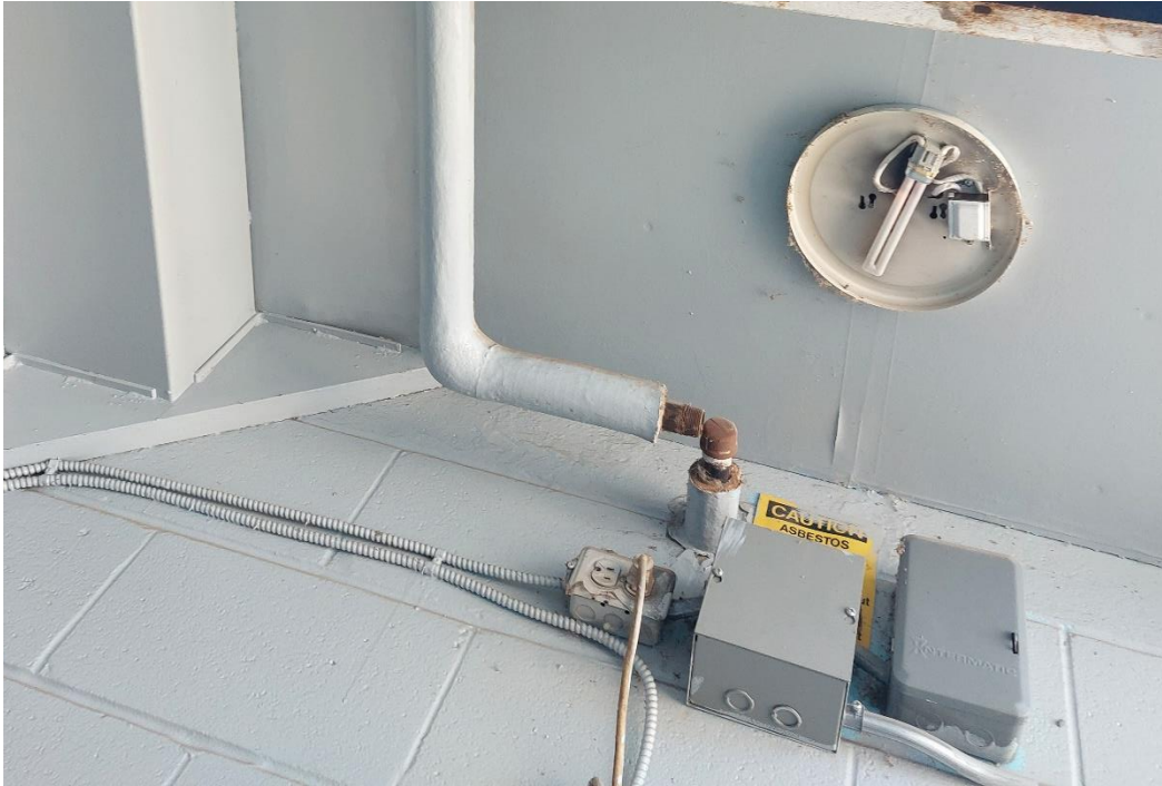
Photograph 7: View of the of the asbestos-containing parging cement fitting in stairwell 2-27.
