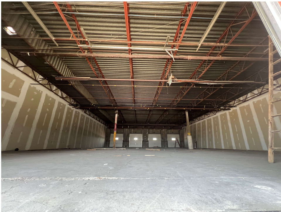
Photo #43: Typical View of Warehouse Interior, North of Office Building
