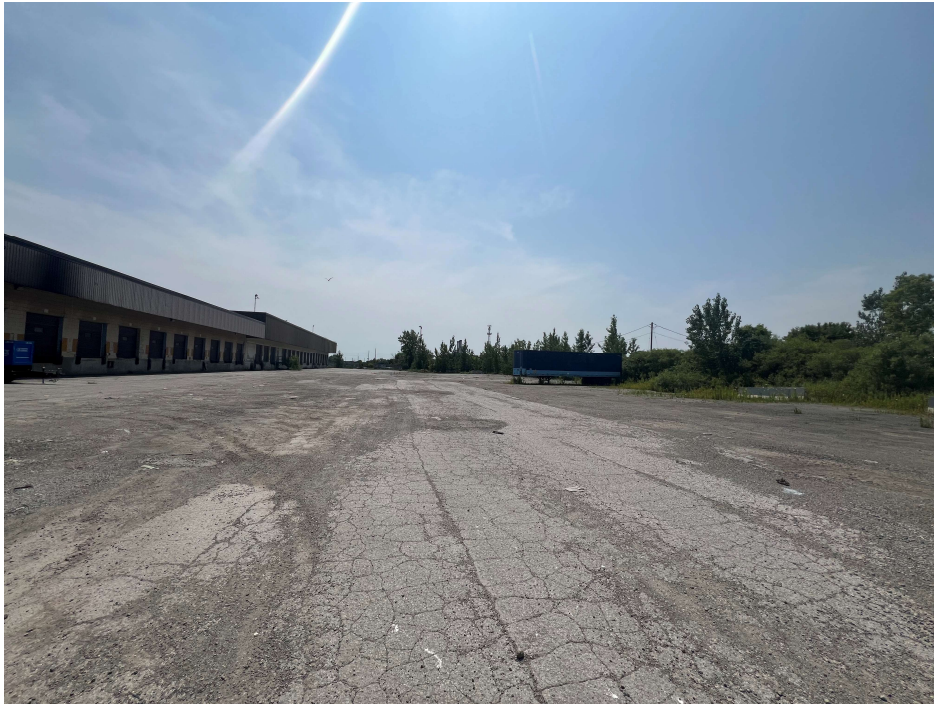
Photo #2: Overview Photo of West Elevation
