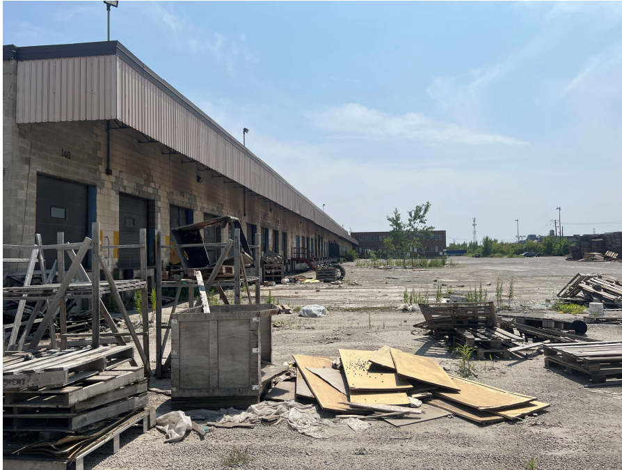
Photo #28: Typical Site Refuse at North Elevation
