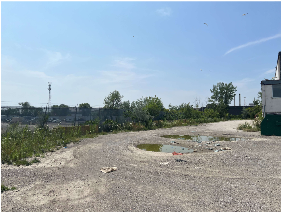
Photo #7: Overview of South Elevation
