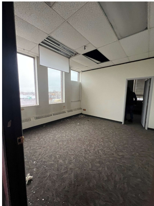
Photo #33: Typical View of Office Building Finishes
