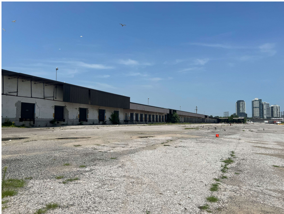
Photo #9: Overview of East Elevation
