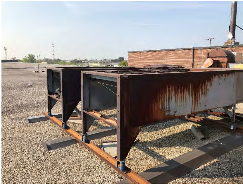
5. View of the roof of the site building located on the central portion of 30 Newbridge Road.
