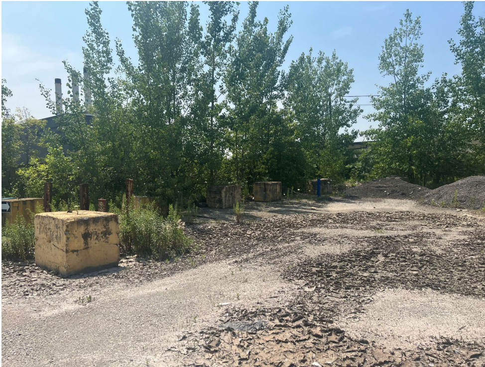
Photo #6: Typical Site Refuse at West Elevation
