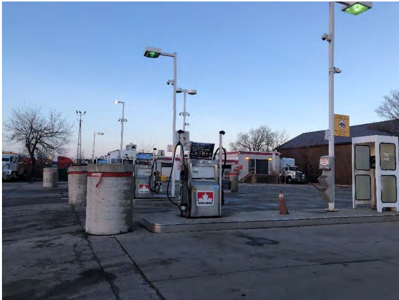
22. View of the gasoline service station located at 58 North Queen Street, to the west of the Site, facing north.
