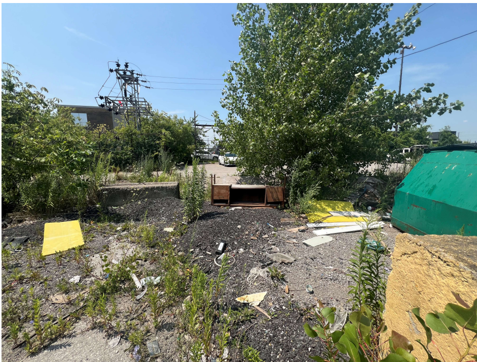
Photo #3: Typical Site Refuse at West Elevation
