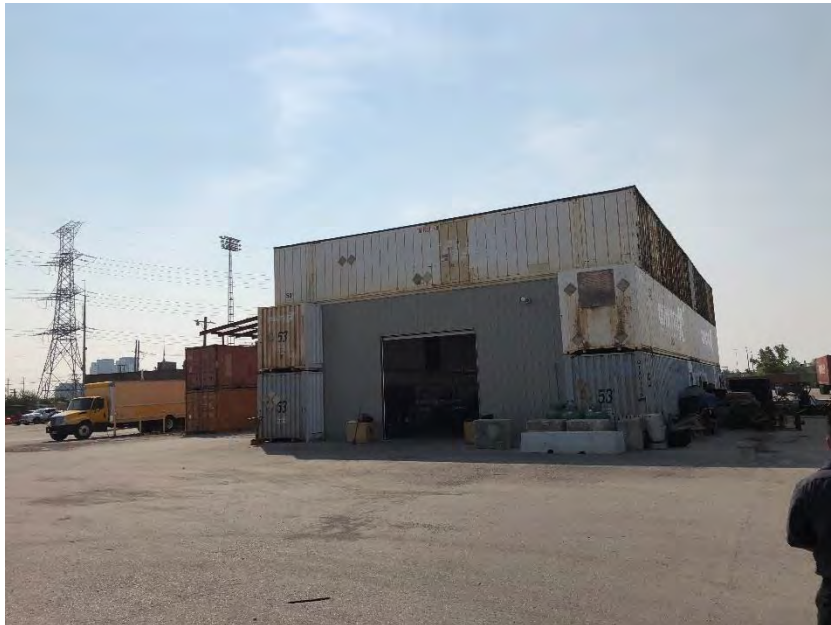
12. View of the auto garage located on the south central portion of 36 North Queen Street, facing northeast.
