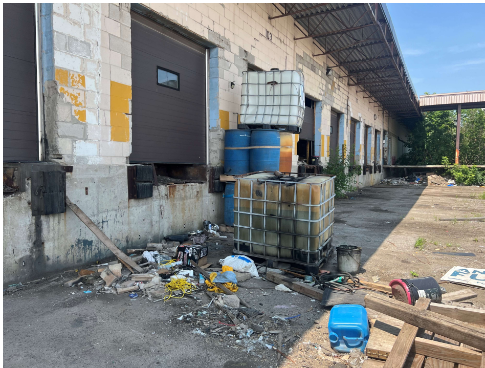
Photo #15: Typical Site Refuse at East Elevation
