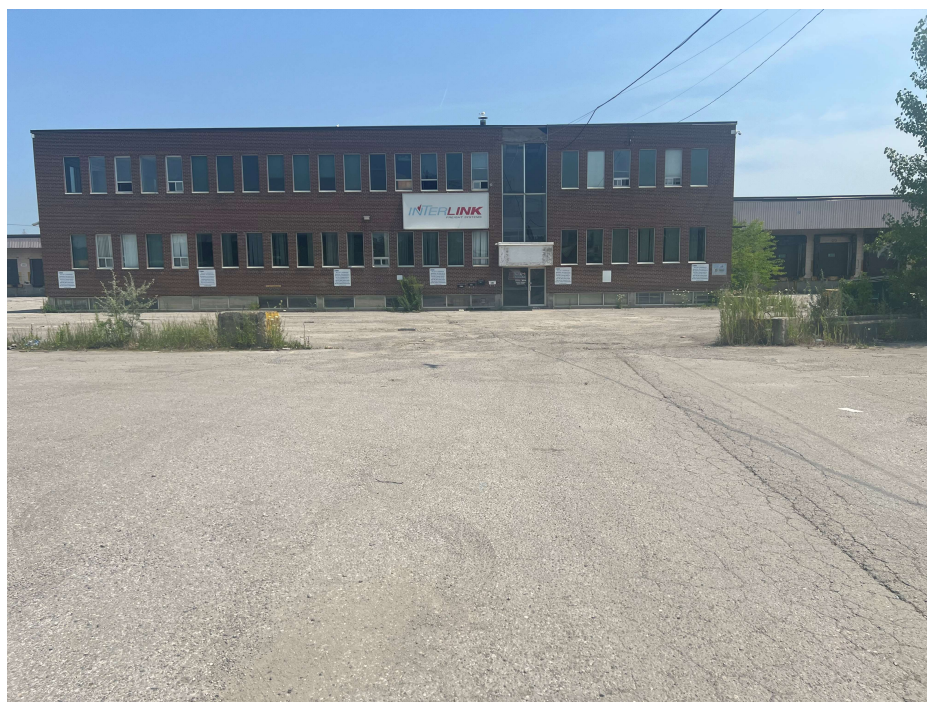
Photo #1: Typical View of Exterior Office Building
