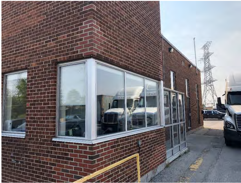
11. View of the building located on 36 North Queen Street, facing southeast.
