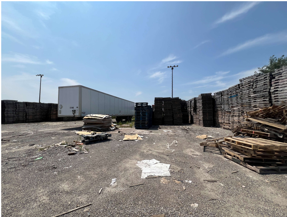
Photo #31: Typical Site Refuse at West Elevation
