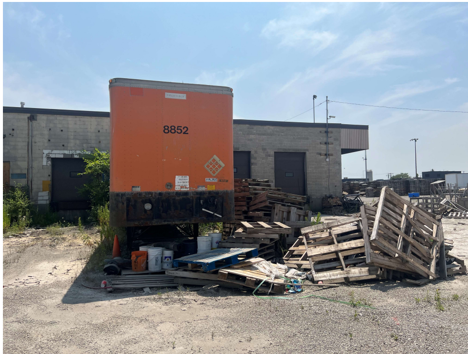
Photo #26: Typical Site Refuse at North Elevation
