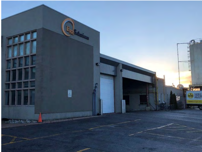
19. View of the west adjacent property, facing southwest.
