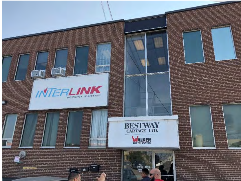
1. View of building located on the central portion of 30 Newbridge Road, facing northeast.
