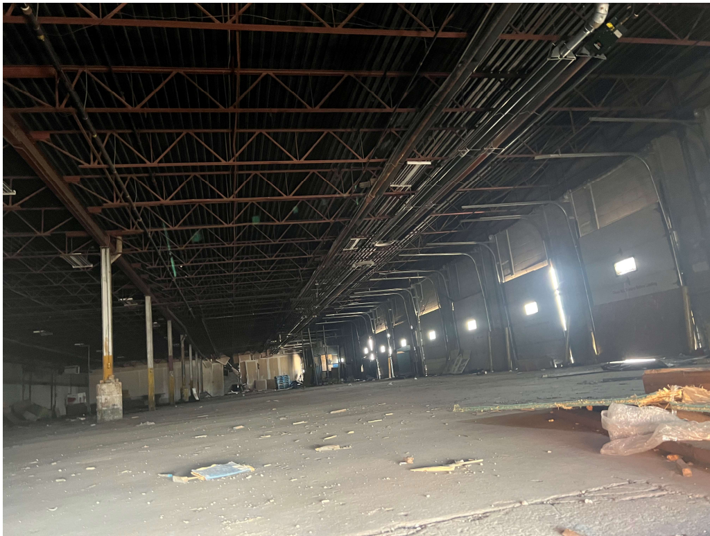
Photo #42: Typical View of Warehouse Interior, North of Office Building
