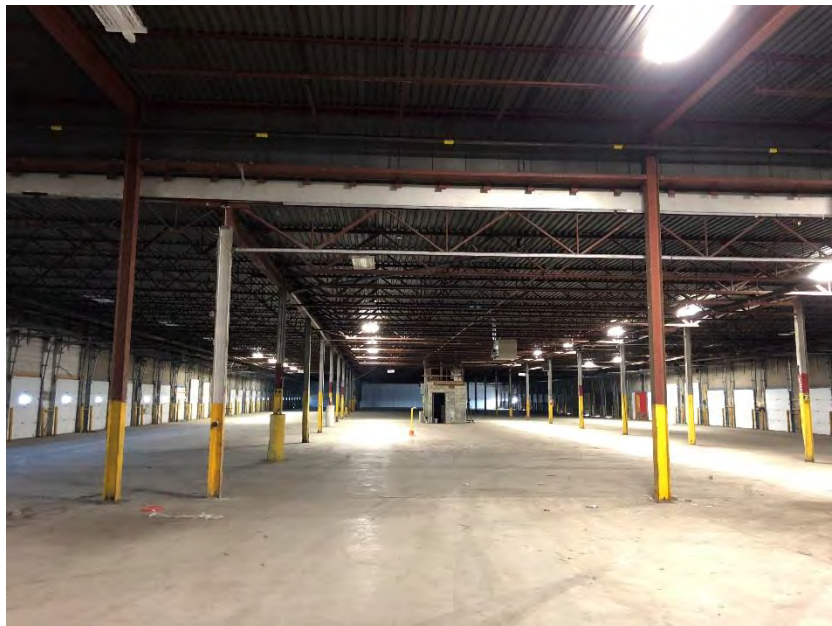
2. View of the interior of the southern portion of the warehouse located within the site building located on the central portion of 30 Newbridge Road.
