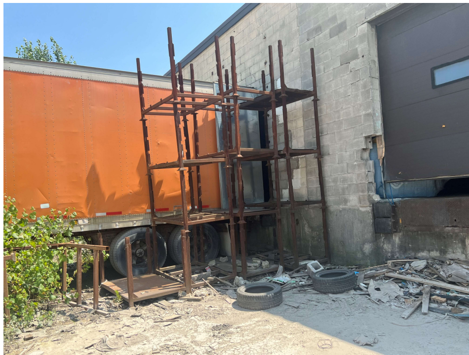
Photo #27: Typical Site Refuse at North Elevation
