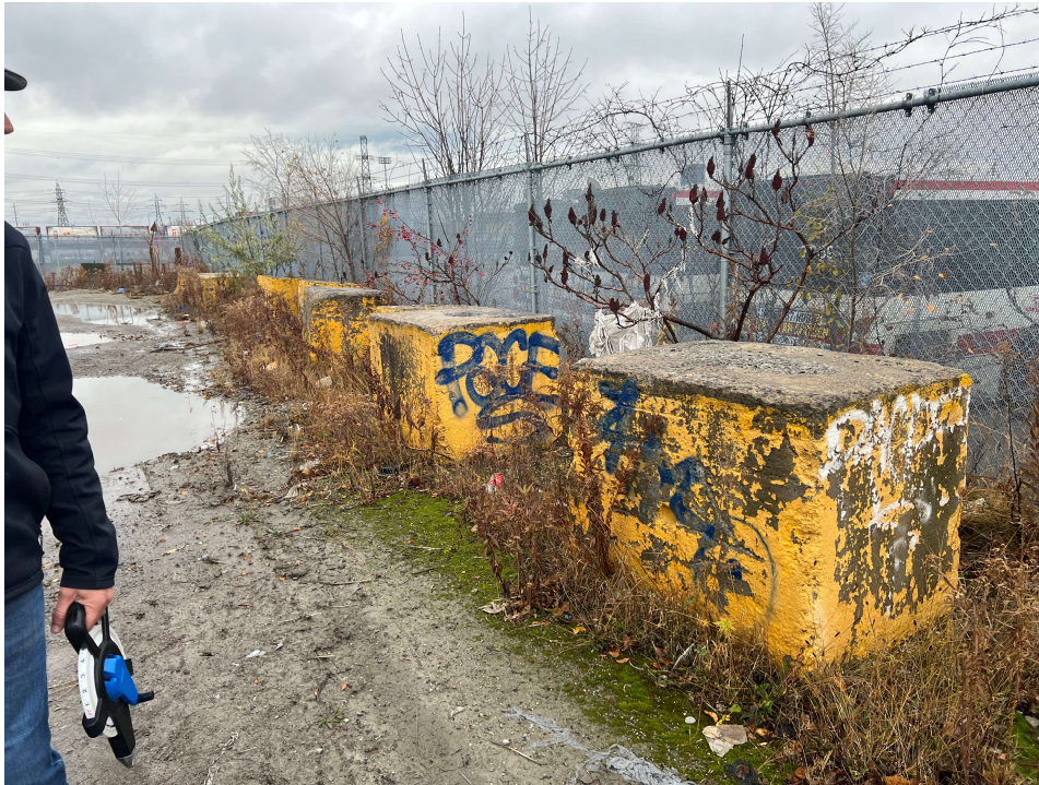
Photo #8: Typical Site Refuse at South Elevation
