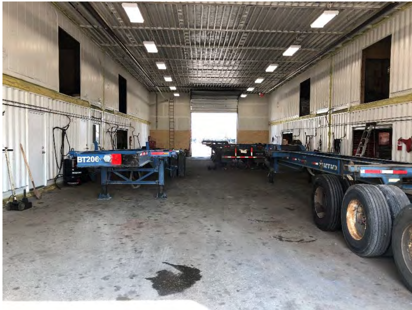
14. View of the interior of the on-site garage, facing east.
