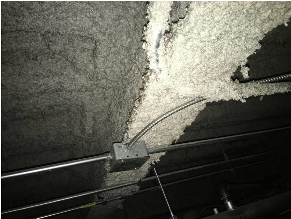
Photo 7 – View of the non-asbestos sprayed fire proofing observed in the ceiling space above Ceiling Tiles on the lower level.
