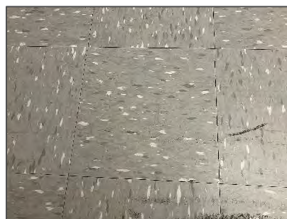
Non-asbestos vinyl floor tiles (VFT04).
