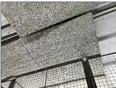
Non-asbestos tectum tiles – Storage Cages (Location B-002).
