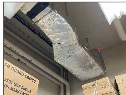
Duct insulated with fiberglass and jacketed in foil – Central Files Storage (Location B-007).
