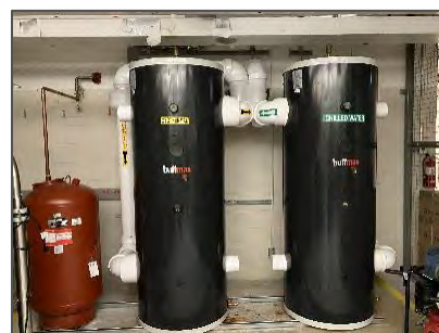
Hot water tanks insulated with fiberglass – Storage Cages (Location B-002).
