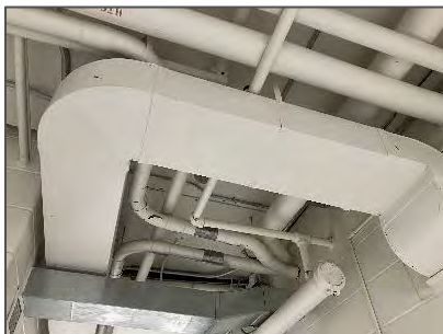
Uninsulated duct – Corridor (Location B-001).
