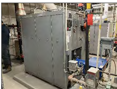
Uninsulated boiler – Boiler Room (Location B-014).
