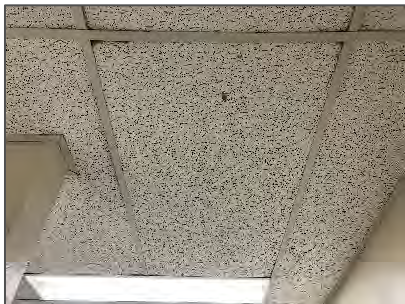
Non-asbestos acoustic ceiling tiles (ACT10).
