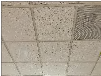
Non-asbestos acoustic ceiling tiles (ACT01).
