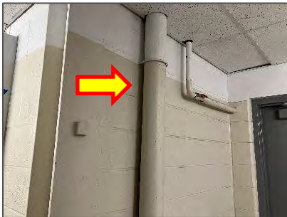
Presumed asbestos-containing Transite pipe – Corridor (Location 1-098).
