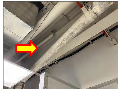
Presumed asbestos-containing Transite pipe – Men's / Women's Change Room (Location 2-145).
