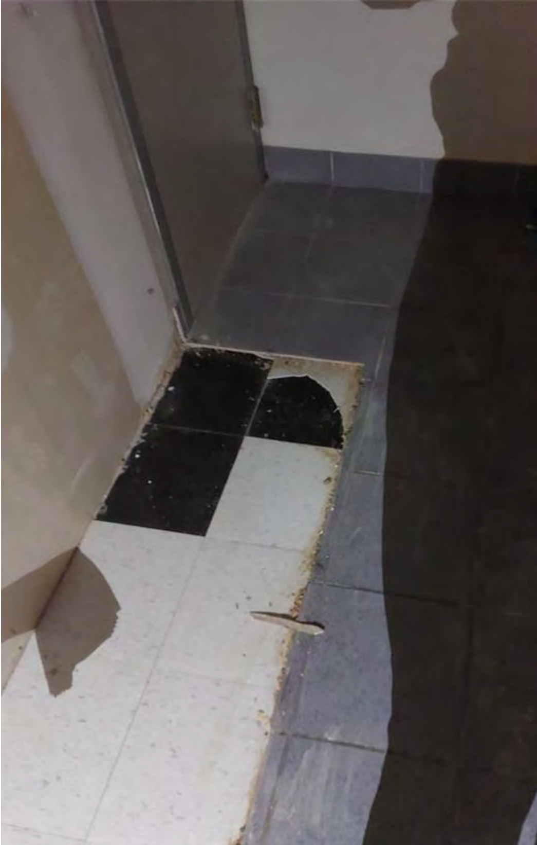
Photo 1 – View of the vinyl floor tile and mastic discovered under ceramic tile.
