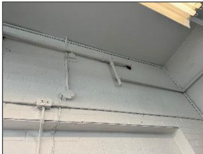
Uninsulated pipes – Storage Space (Location 1-01).
