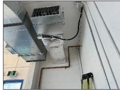
Duct insulated with fibreglass and jacketed in foil – Garage (Location 1-07).
