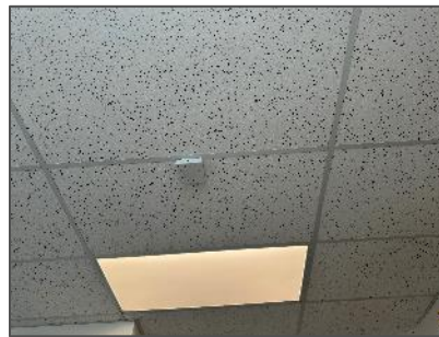
Non-asbestos acoustic ceiling tiles (ACT01).
