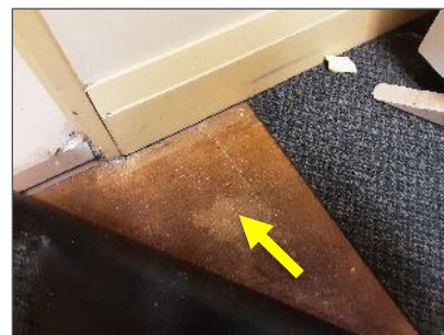
Non-asbestos yellow mastic under blue carpet in office areas, Membership and Guest Centre (HMIS Loc. 1).
