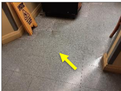
Non-asbestos VFT-01, 12"x12" light grey with white flakes, in C3 connection building, Membership and Guest Centre (HMIS Loc. 1).
