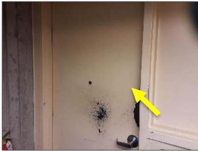
L0001, Yellow paint within insignificant lead content on metal door frame in office area, Membership and Guest Centre (HMIS Loc. 1).
