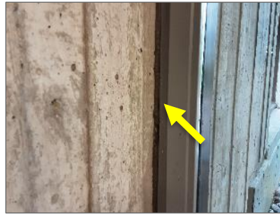
Non-asbestos black caulking on exterior guest entrance door frame, Membership and Guest Centre (HMIS Loc. 1).
