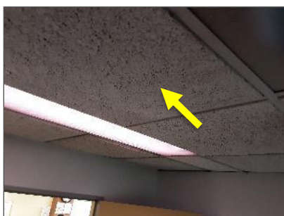
Non-asbestos ACT-01, 24"x48", lay-in, Textured finish Membership and Guest Centre (HMIS Loc. 1).
