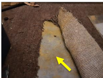
Non-asbestos yellow mastic under red carpet, Membership and Guest Centre (HMIS Loc. 1).
