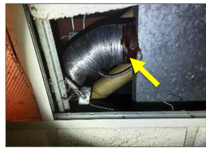
Asbestos-containing red mastic is present on ducts seams/joint, Membership and Guest Centre (HMIS Loc. 1).
