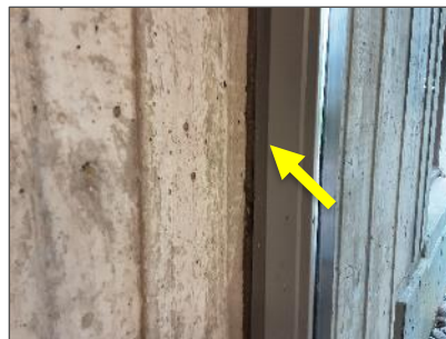
P0001, Non-PCB black caulking is present on metal door frame in guest entrance area, Membership and Guest Centre (HMIS Loc. 1).
