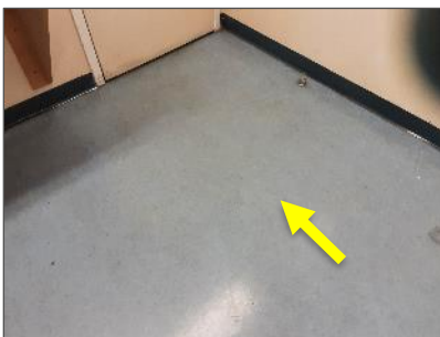
Non asbestos blue vinyl sheet flooring in accounting room S0006A-C, Membership and Guest Centre (HMIS Loc. 1).
