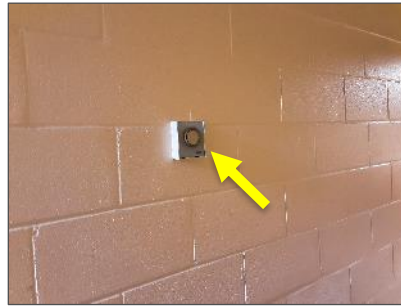
Thermostat ampules is present in C3 connection building, Membership and Guest Centre (HMIS Loc. 1).
