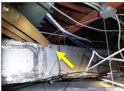
Foil-faced fiberglass insulated duct, Membership and Guest Centre (HMIS Loc. 1).
