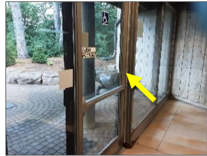
L0003, Grey paint with low-level lead content on metal door frame in guest entrance door, Membership and Guest Centre (HMIS Loc. 1).
