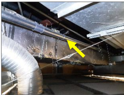
Uninsulated pipe, Membership and Guest Centre (HMIS Loc. 1).
