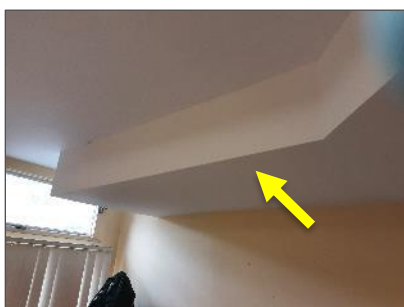
Non-asbestos drywall joint compound on bulkhead in GR Supervisor room S0005A-C, Membership and Guest Centre (HMIS Loc. 1).
