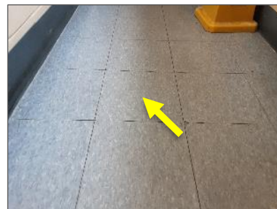
Non-asbestos VFT-02, 12"x12" light blue with white flakes in Lunch area, Membership and Guest Centre (HMIS Loc. 1).
