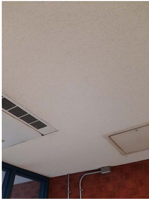
Photograph No. 4 – Texture coat ceilings were observed within the lobby and main entrance vestibule. The texture coat was sampled (S03A,B,C) and found to be non-asbestos.
