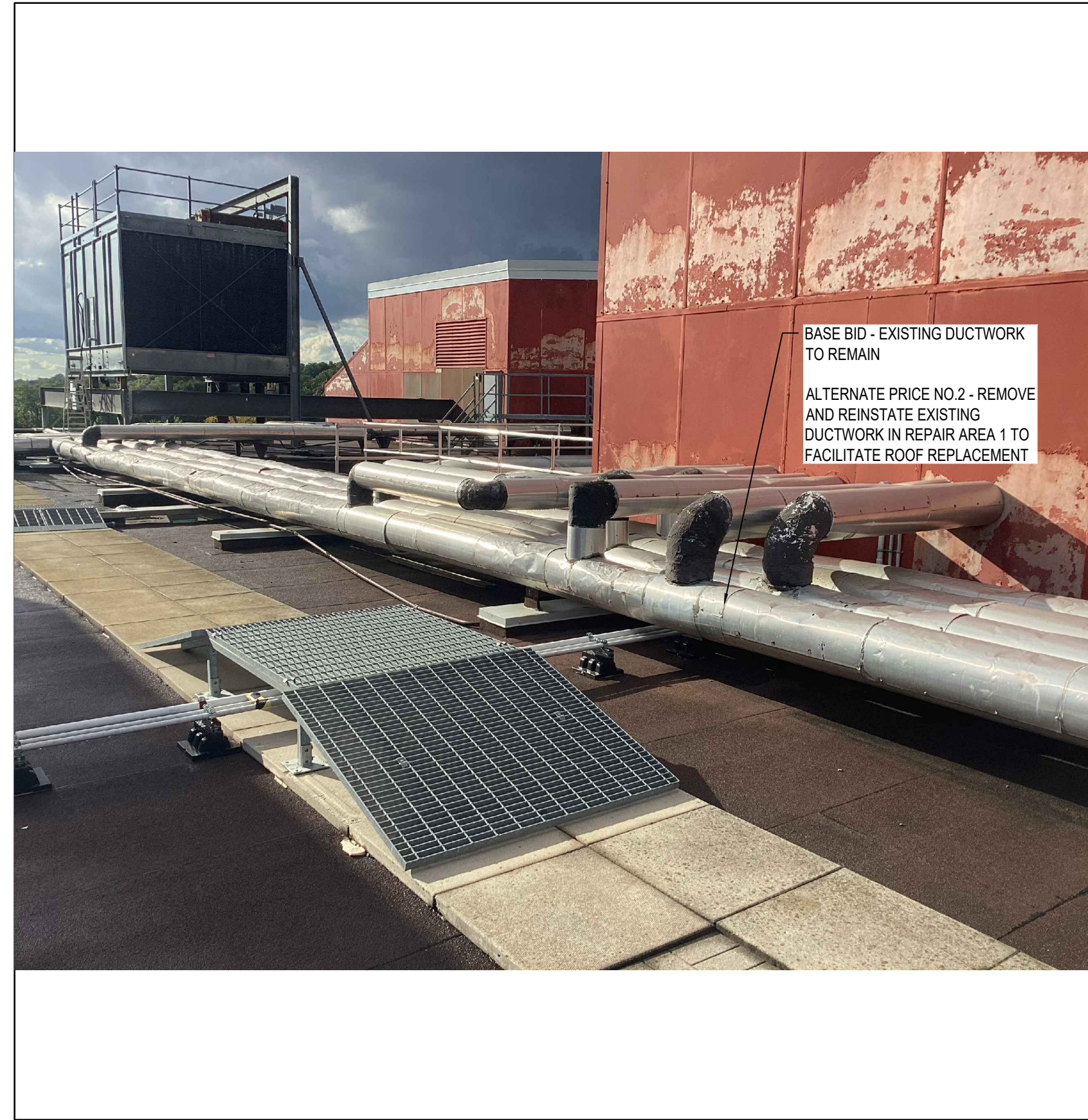
2 VIEW OF ROOF C (REPAIR AREA 1) R600
