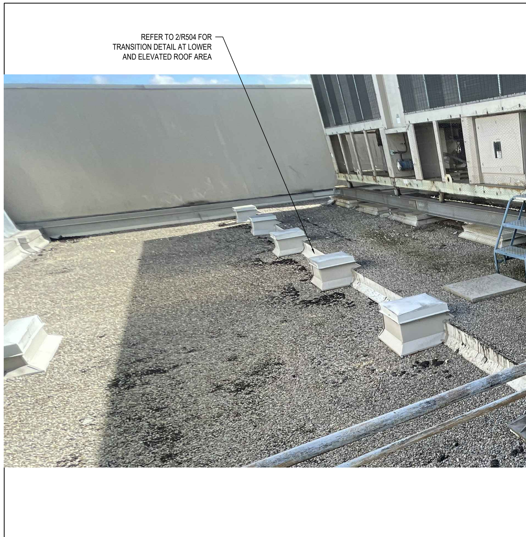
3 VIEW OF ELEVATED ROOF AREA R602
