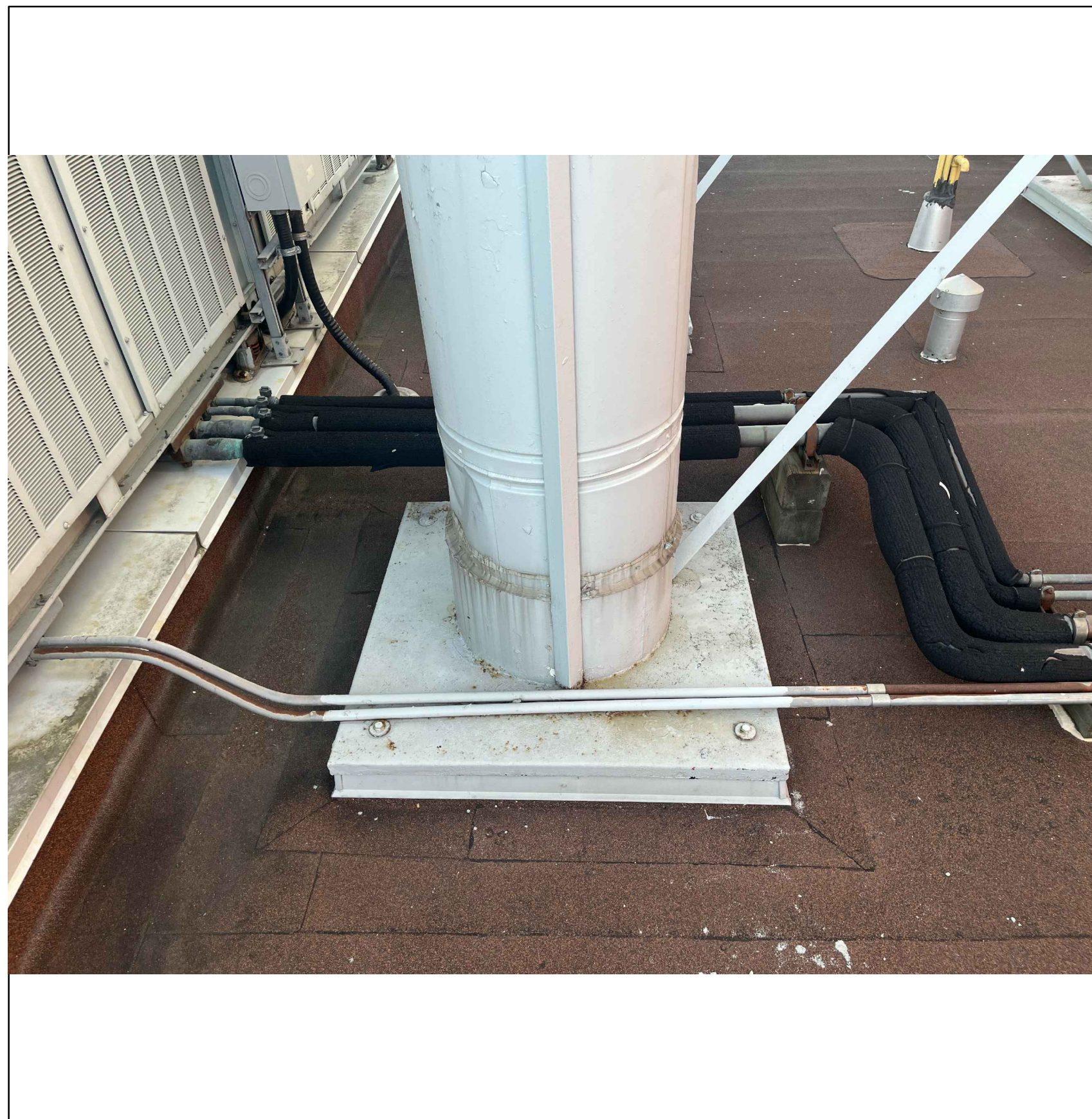
4 BOILER VENT BASE FLASHING R601
