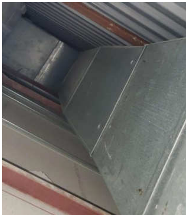
Duct, All, Not Insulated, Cafeteria (Location #: 103)
