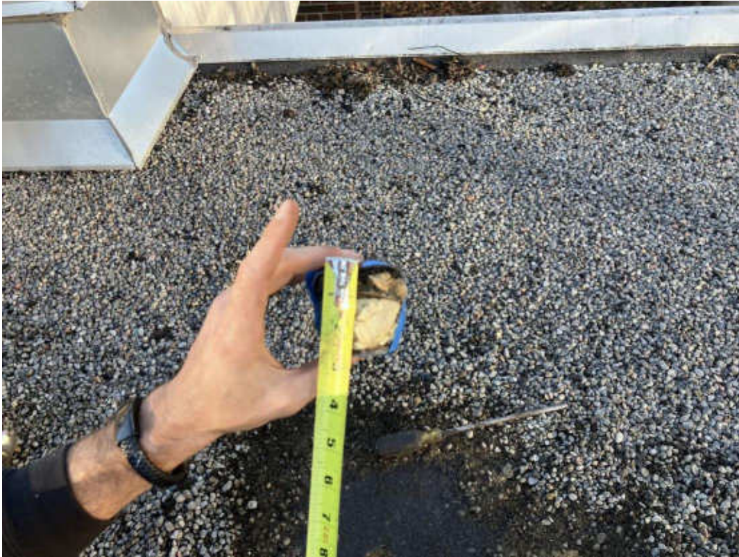
S1019A (Non-asbestos), Roofing materials, Roof E (Location #: 214)
