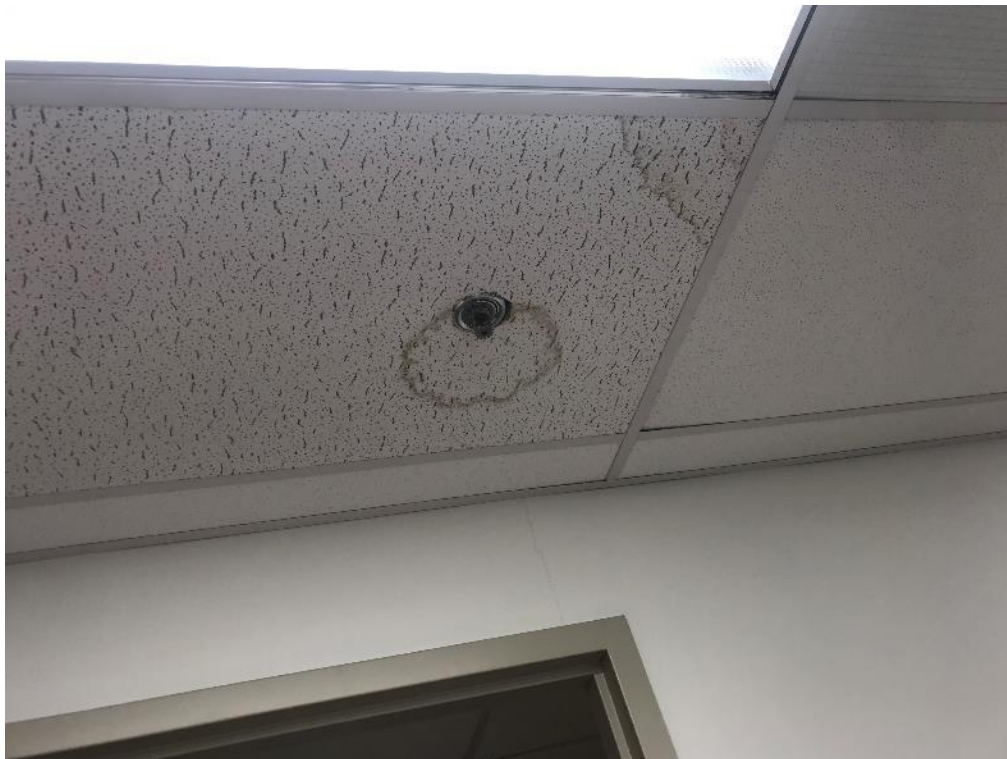
Photos 13, 14 – View of water staining on non-asbestos containing ceiling tile in Meeting Room, 1-048.
