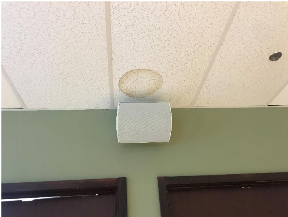
Photos 17, 18 – View of water staining on non-asbestos containing ceiling tile in Chapel, 1-068.
