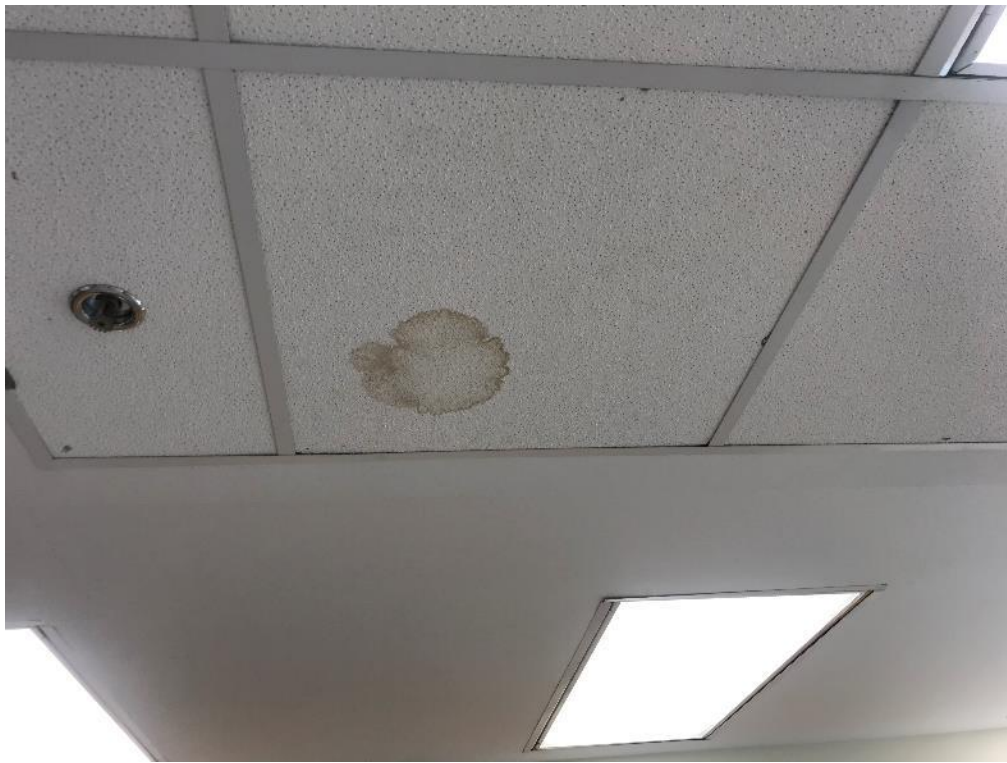
Photos 23, 24 – View of water staining on non-asbestos containing ceiling tiles in Program Centre, 4-047.
