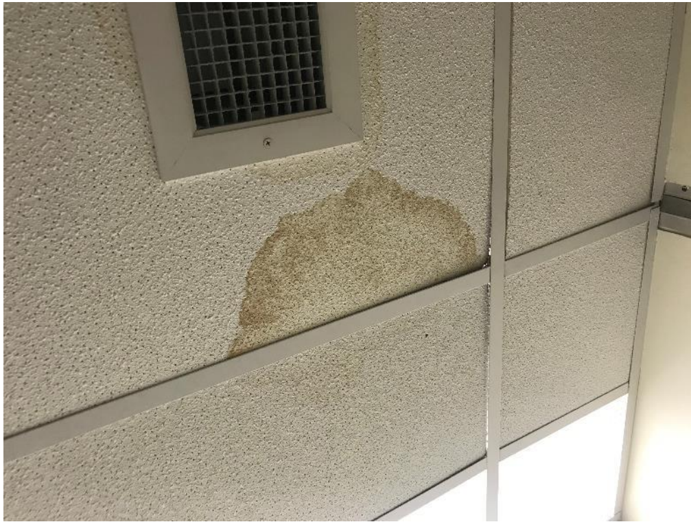
Photos 25, 26 – View of water staining on non-asbestos containing ceiling tiles in Washroom, 4-053.
