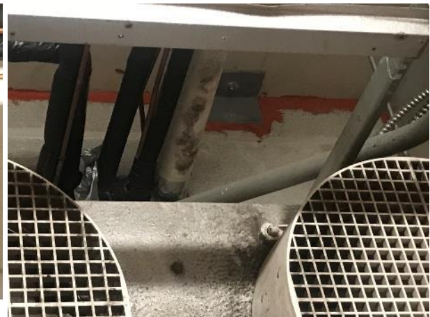
Photos 3 to 8 – View of mould growth on fibreglass pipe insulation in Garbage Room, 1-026.
