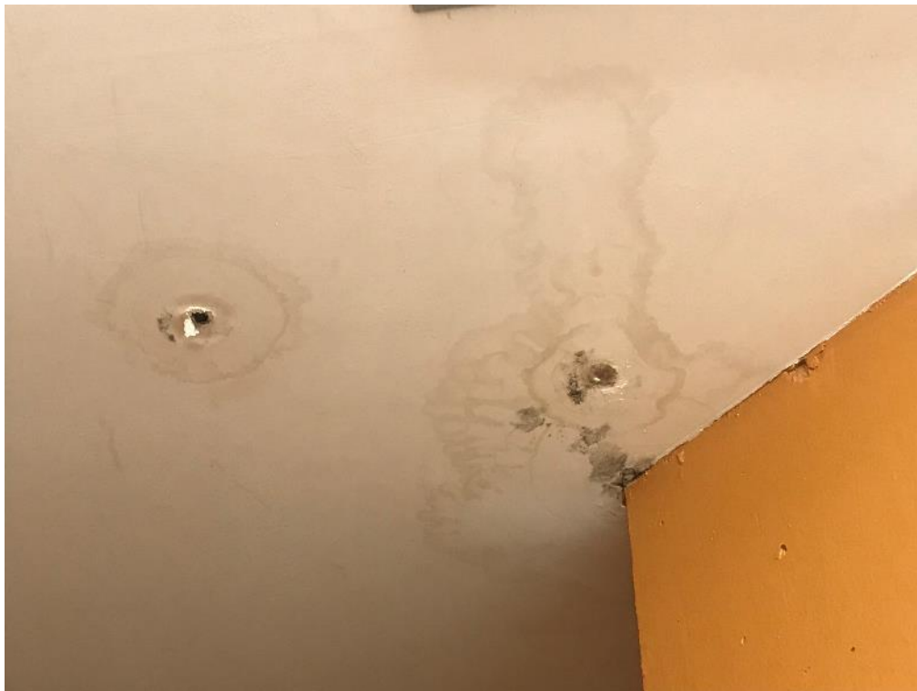
Photos 1, 2 – View of mould growth on non-asbestos containing drywall ceiling in Soiled Linen, 1-025.
