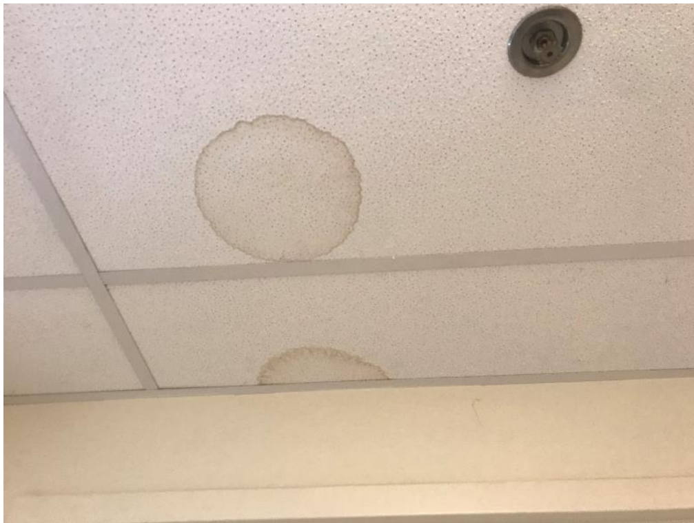
Photos 27, 28 – View of water staining on non-asbestos containing ceiling tiles in the North Corridor, 4-098.
