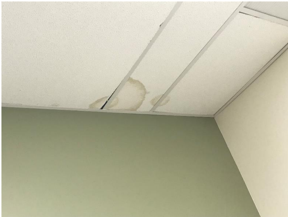
Photos 15, 16 – View of water staining on non-asbestos containing ceiling tiles in Staff Lounge, 1-064.
