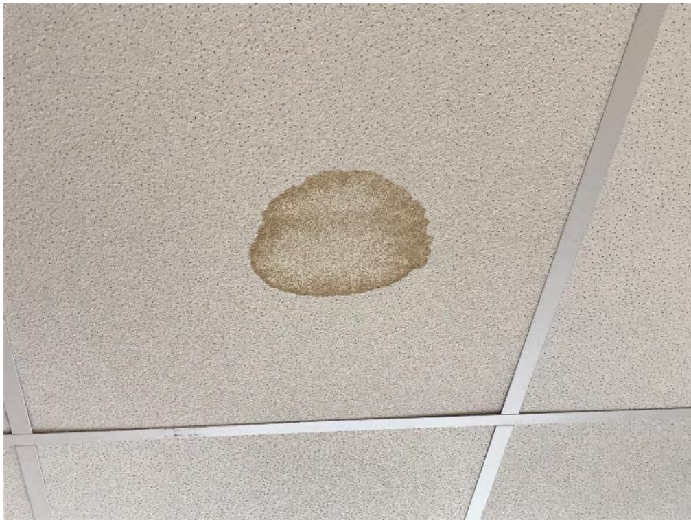
Photos 11, 12 – View of water staining on non-asbestos containing ceiling tile in Beauty Salon, 1-043.
