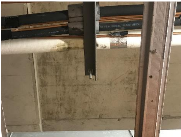
Photos 3 to 8 – View of mould growth on fibreglass pipe insulation in Garbage Room, 1-026.
