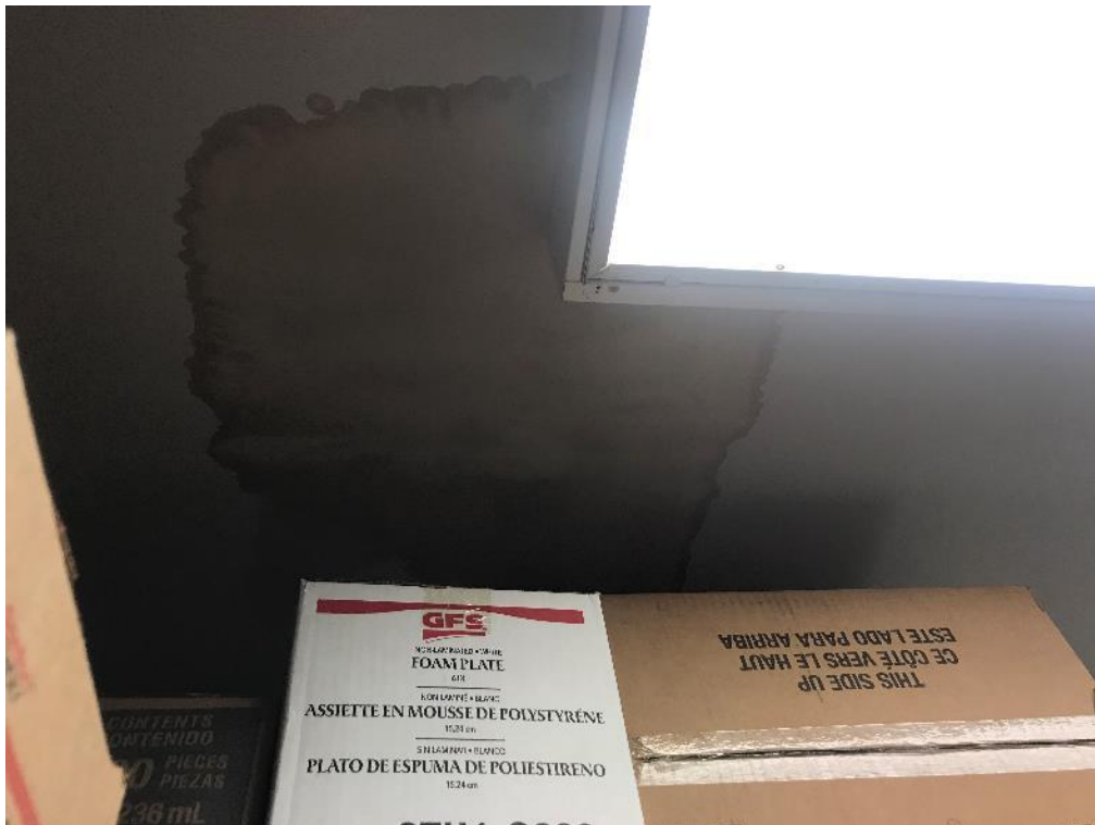
Photos 19, 20 - View of water staining on non-asbestos containing drywall ceiling in Storage, 4-099.
