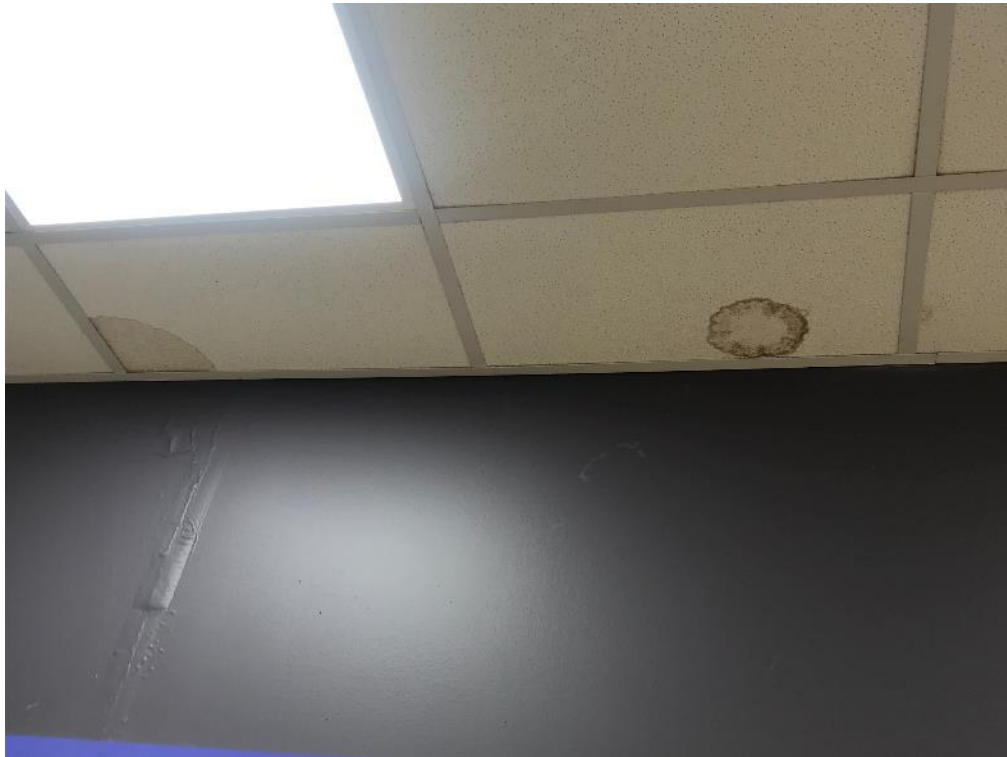
Photos 9, 10 – View of water staining on non-asbestos containing ceiling tiles in Town Hall, 1-065.
