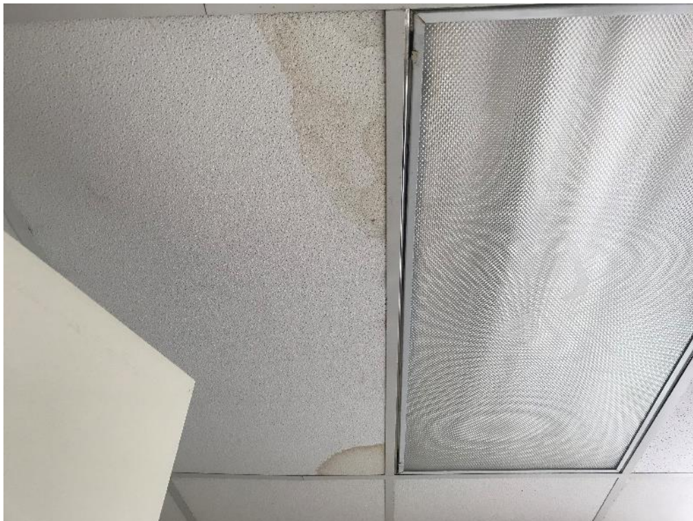
Photos 21, 22 – View of water staining on non-asbestos containing ceiling tiles in Office, 4-026.
