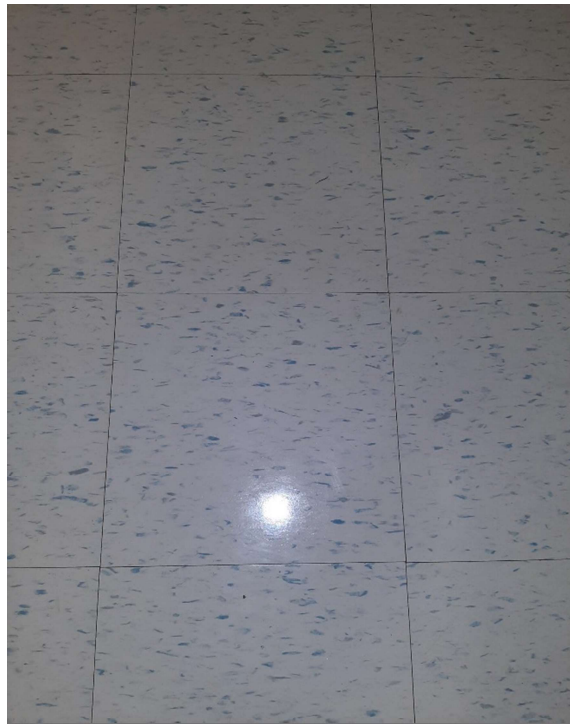
Photograph No. 2 – 12”x12” White with blue fleck vinyl floor tiles observed in Room 167 were sampled (S01A,B,C). The tiles and mastic are non-asbestos.
