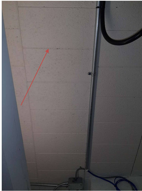
Photograph No. 3 – The concrete mortar on the ceiling of room 167 was sampled (S02A,B,C) and is not asbestos-containing.
