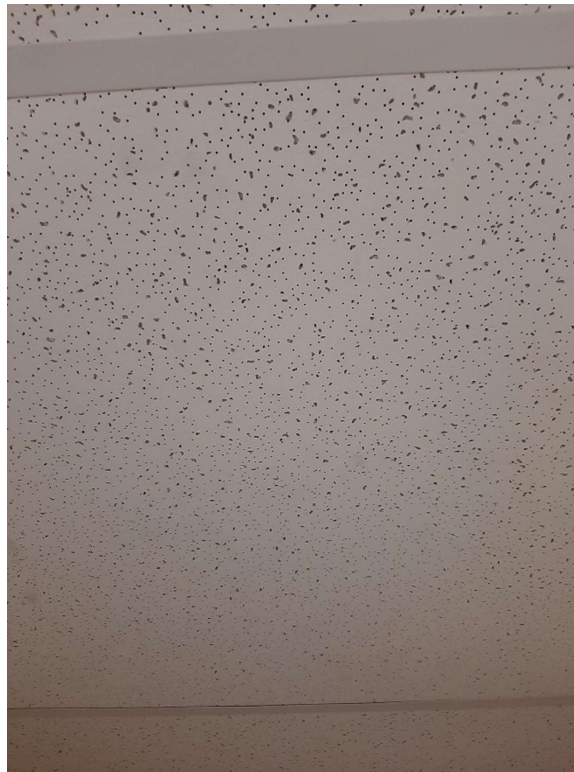
Photograph No. 4 – 2'x4' small fissure random pinhole ceiling tiles were observed in room 102 and were sampled (S04A,B,C). The ceiling tiles are not asbestos-containing.
