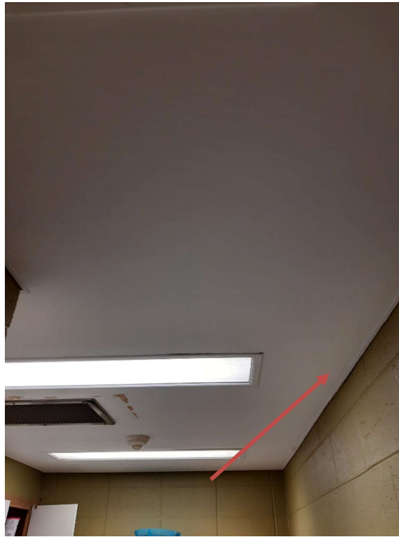
Photograph No. 1 – Drywall joint compound on the ceiling of the Staff Room Kitchen was sampled (S05A,B,C). The joint compound contains asbestos.
