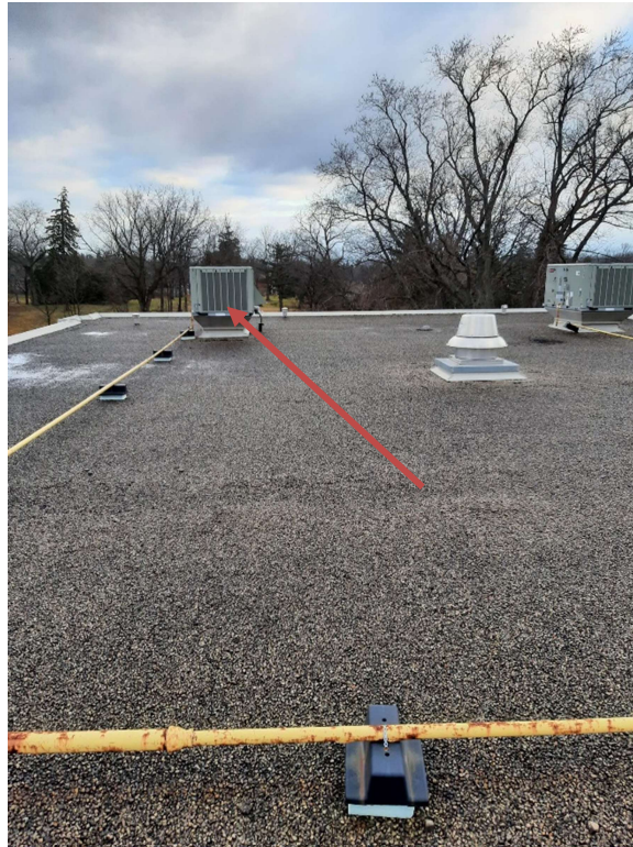
Photograph No. 7 – Rooftop air handling units were observed and are assumed to contain ozone depleting substances.
