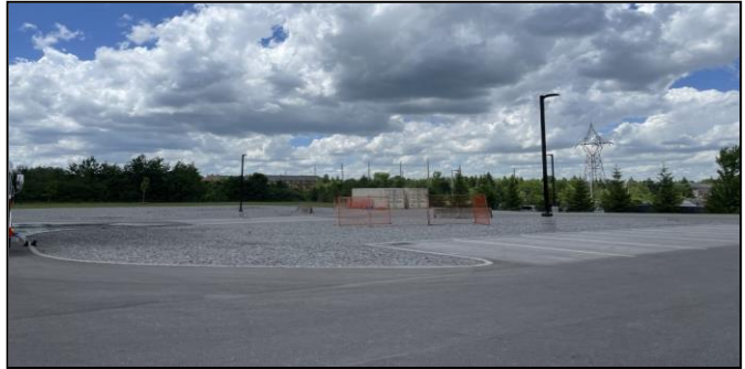
General view of work area
