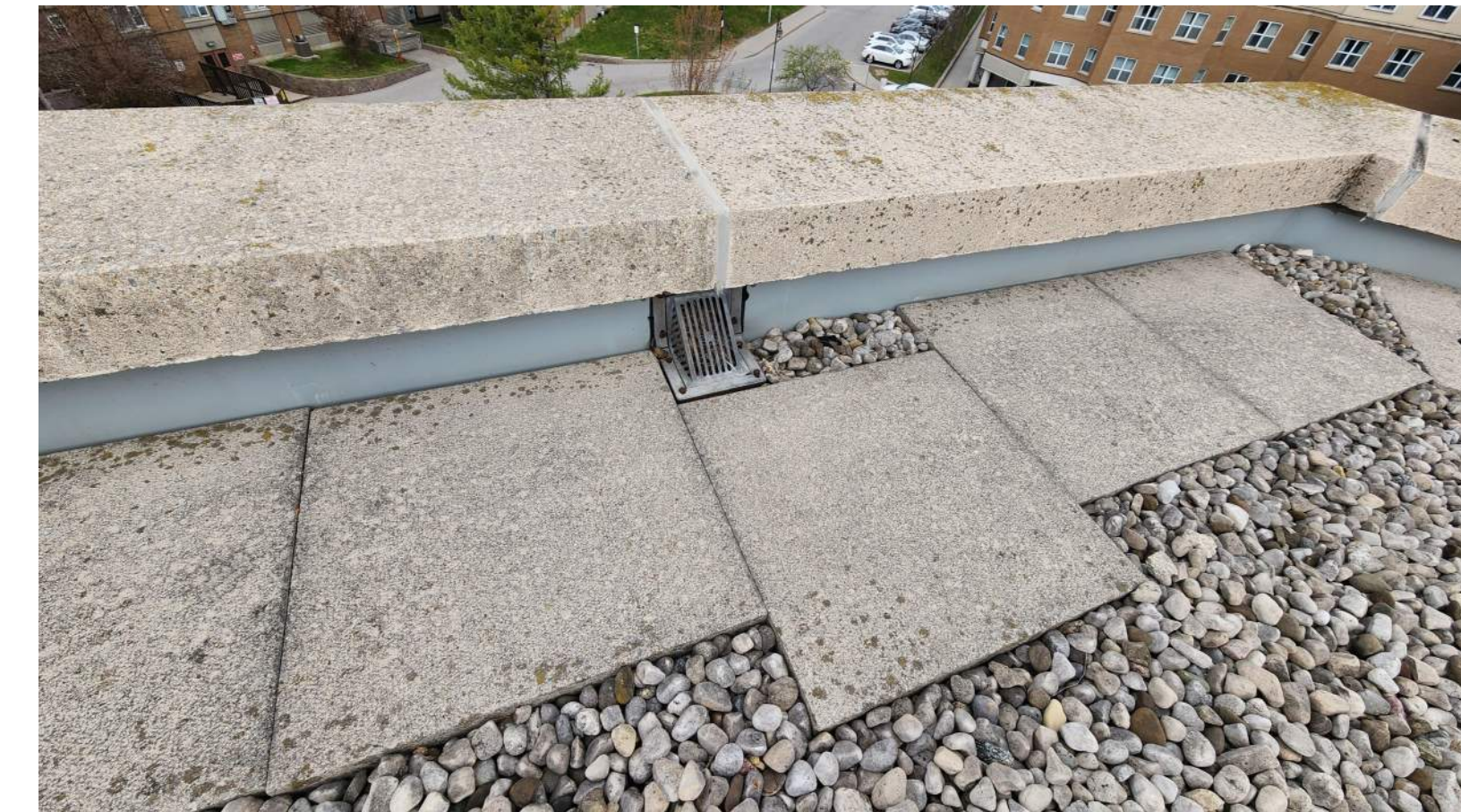
ECP #10_TYPICAL OVERFLOW SCUPPER ECP #10_TYPICAL PARAPET
