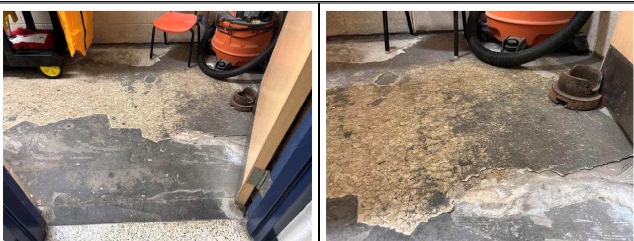
**Figure 1:** View of ACM vinyl sheet flooring in 2<sup>nd</sup> Floor Custodian Room.
