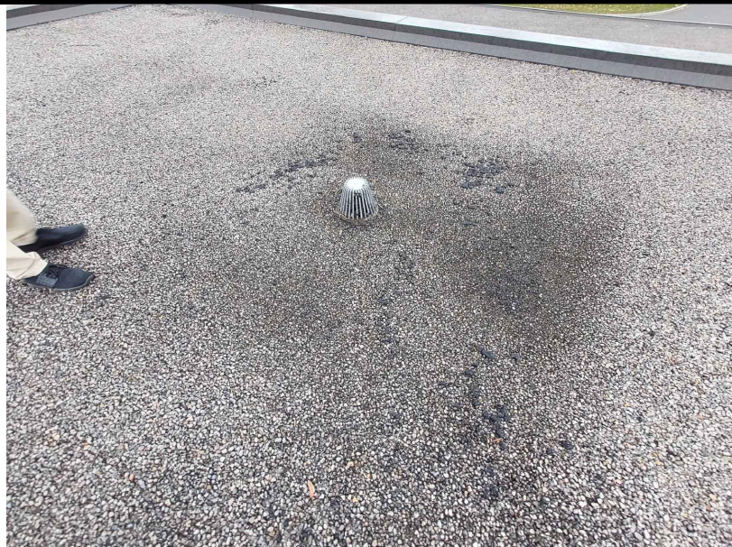
4. GYM ROOF DRAIN
