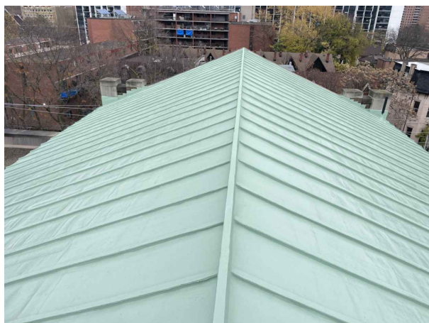
16. SOUTH VIEW OF SLOPED ROOF
