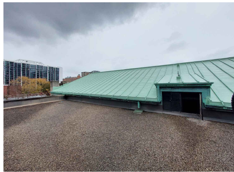
1. PARTIAL NORTH VIEW OF SLOPED ROOF
