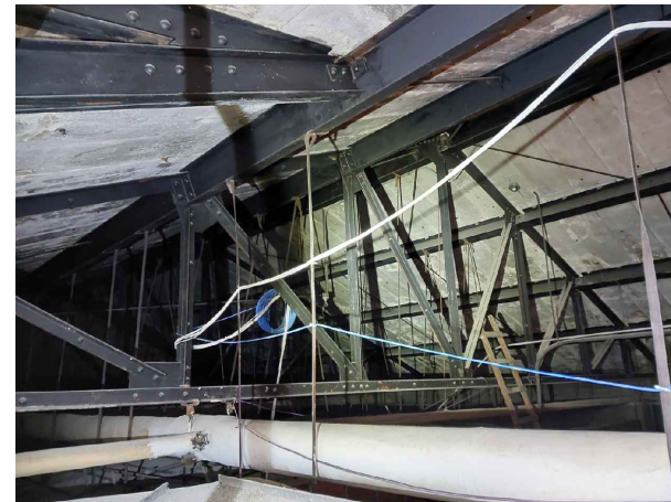
6. ROOF METAL (TRUSSES) AND FRAMING
