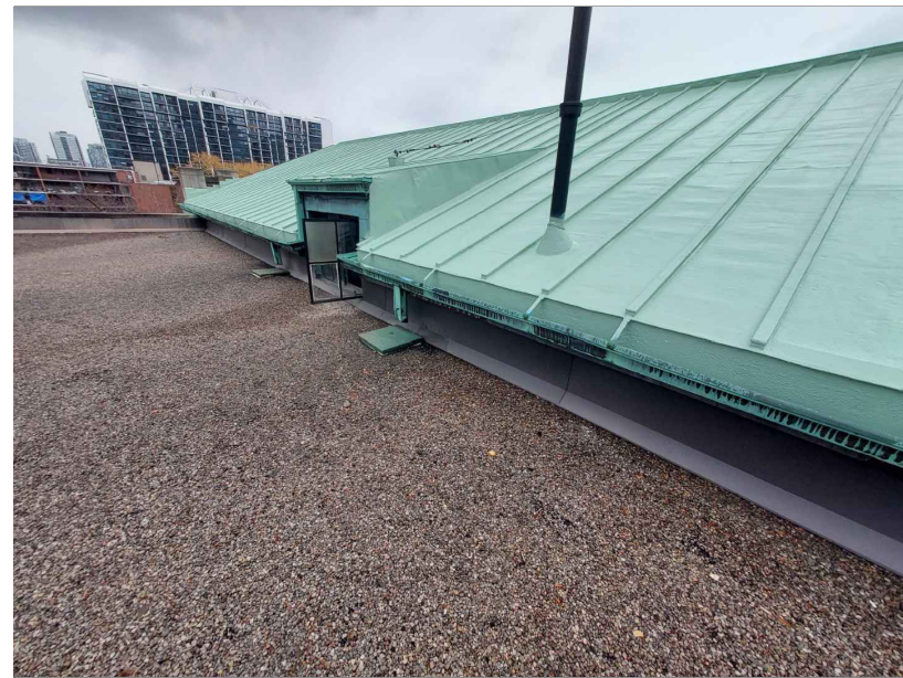
3. NORTH VIEW OF SLOPED ROOF
