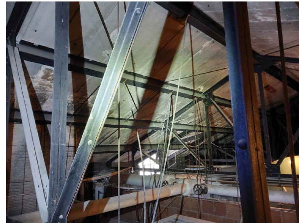
9. ATTIC SPACE BELOW SLOPED ROOF
