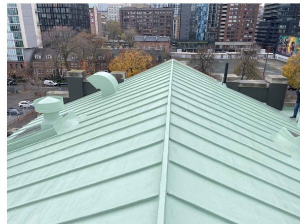
14. WEST VIEW OF SLOPED ROOF
