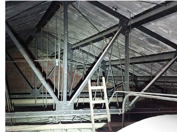
11. SLOPED ROOF METAL TRUSSES
