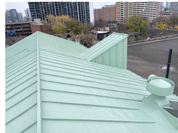
15. SOUTHWEST VIEW OF SLOPED ROOF
