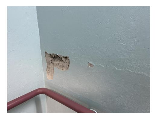
Photo 2: Black stain on the concrete wall in the Stairwell 6 (Loc. 1-102).
