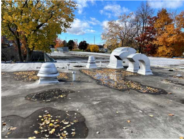
Roof over Washrooms (cont.)
