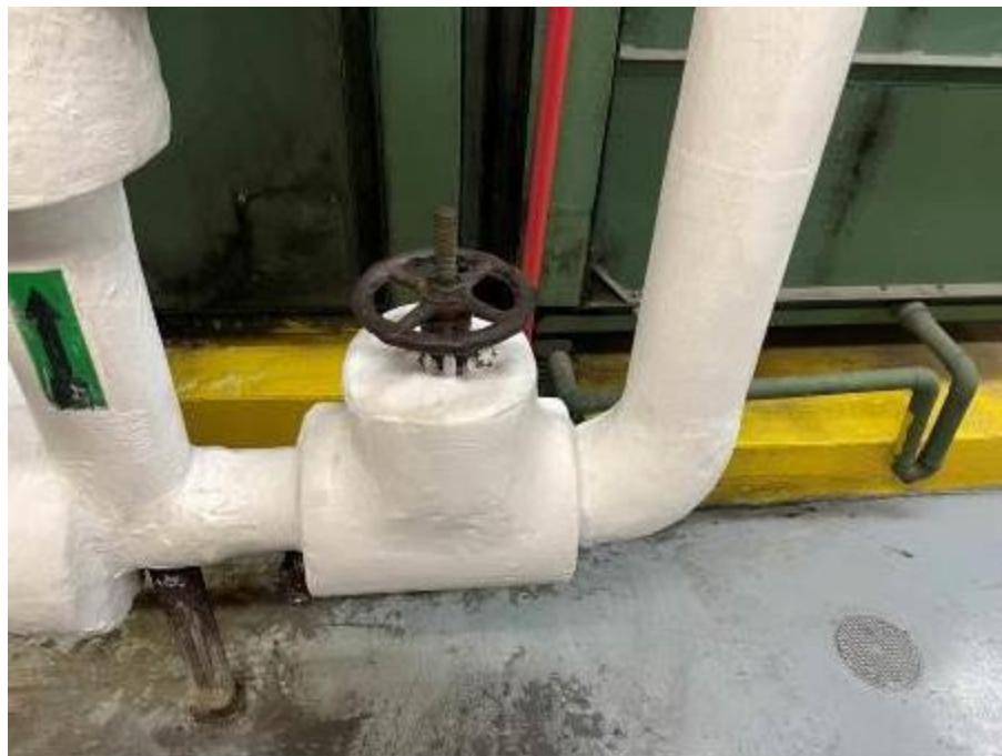
Photos 5 and 6: Post abatement view of the pipe fittings in the East Mechanical Room (B-053).
