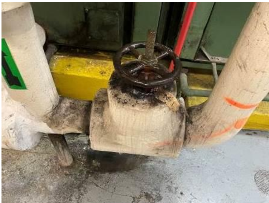
Photos 3 and 4: View of the mould-impacted fittings before the abatement work.
