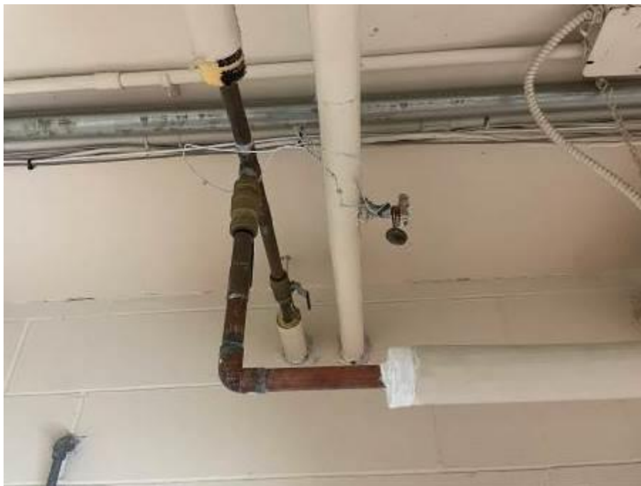
Photo 10: Post-abatement view of the fitting in the Laundry Room (B-007).
