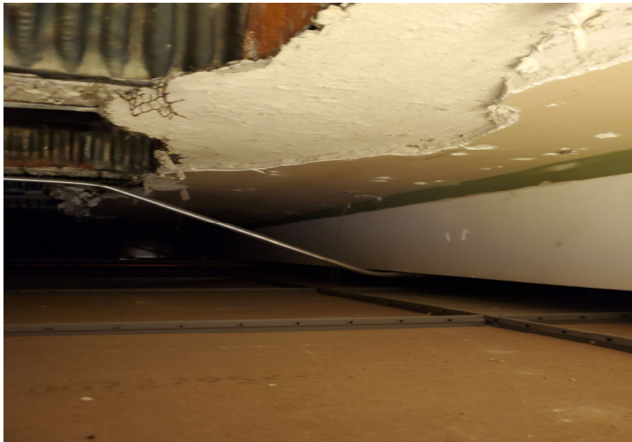
Location #112B (Classroom) – Smooth plaster remains around the perimeter of the room
