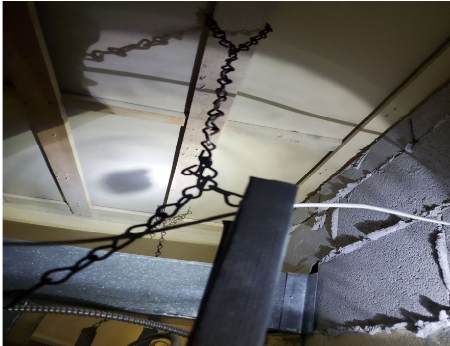
Location #348 (Men's Washroom) – Smooth plaster in GOOD condition. Reinforced with wood strapping
