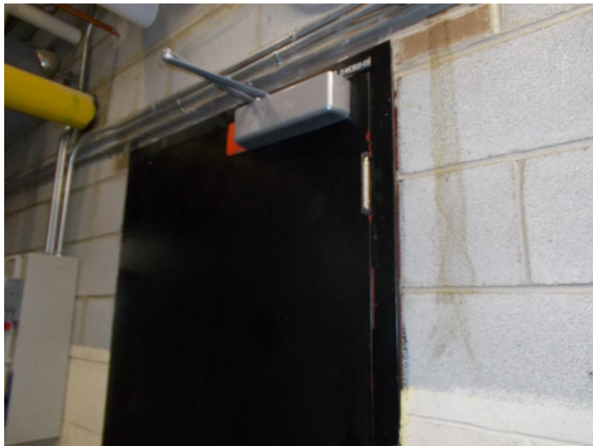
Photograph 6: View of the lead-containing brown paint observed on the door in Room MC-B22 at the Subject Location.
