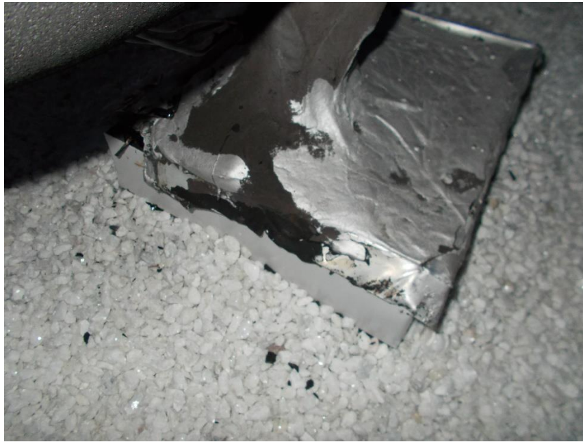
Photograph 1: View of the asbestos-containing black tar observed on the roof at the Subject Location.
