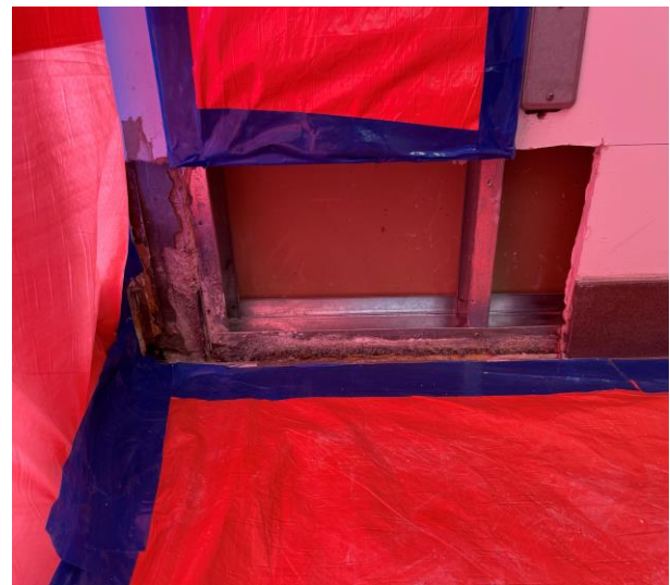
Photo 4: Drywall on west wall after abatement (Loc. 1037)
