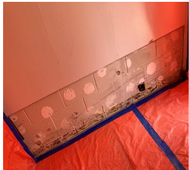
Photo 6: Drywall on east wall after abatement (Loc. 1037)
