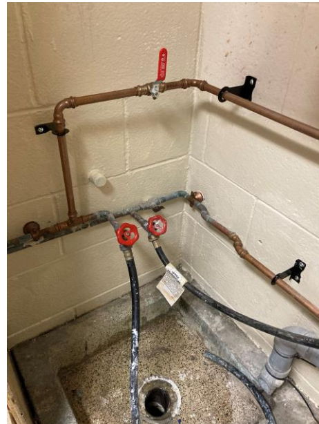
Photo 2: Concrete block wall after abatement (Loc. JC-12)
