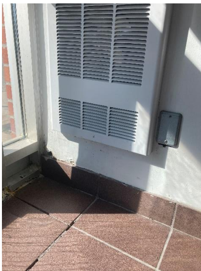
Photo 3: Water-damaged drywall on west wall prior to abatement (Loc. 1037)
