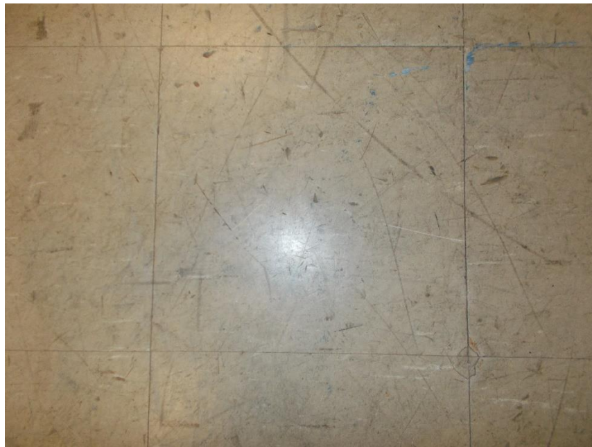
Photograph 4: View of the asbestos-containing VFTs observed in Room 2002 at the Subject Location
