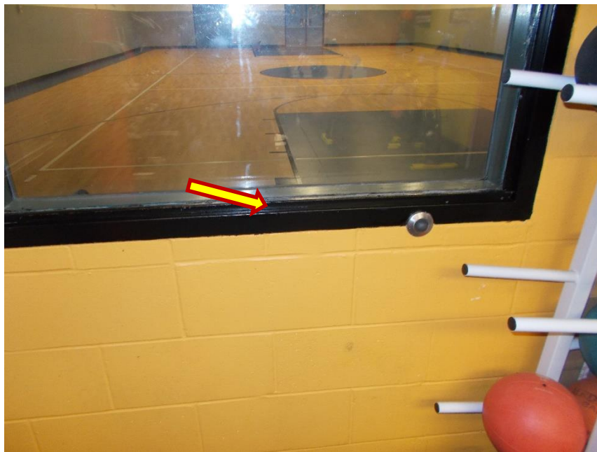
Photograph 2: View of the asbestos-containing caulking observed in Room 2002 at the Subject Location.
