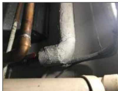
Photo 2: Non-asbestos paring cement – Mechanical Room (Location 1-04).
