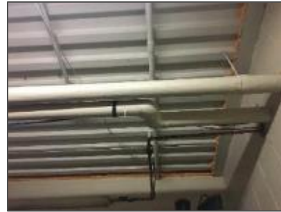
Photo 4: Pipe insulated with fiberglass – Equipment Storage (Location 1-05).
