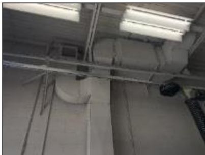
Photo 5: Uninsulated duct – Fire Apparatus Bay (Location 1-01).
