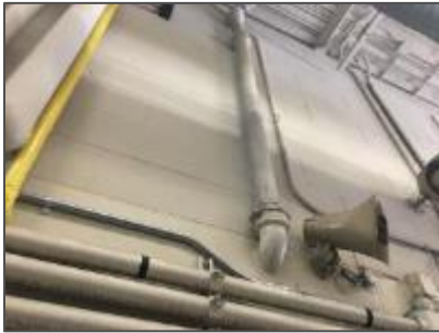
Photo 3: Uninsulated pipe – Fire Apparatus Bay (Location 1-01).
