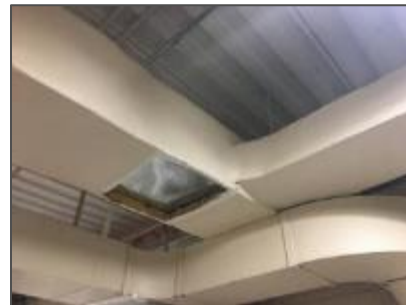
Photo 6: Duct insulated with fiberglass – Supply Room (Location 1-03).
