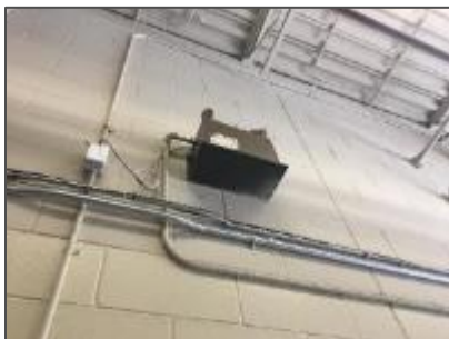
Photo 11: Emergency lighting – Fire Apparatus Bay (Location 1-01).
