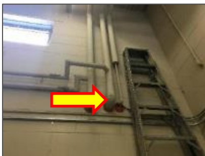
Photo 1: Non-asbestos paring cement – Fire Apparatus Bay (Location 1-01).
