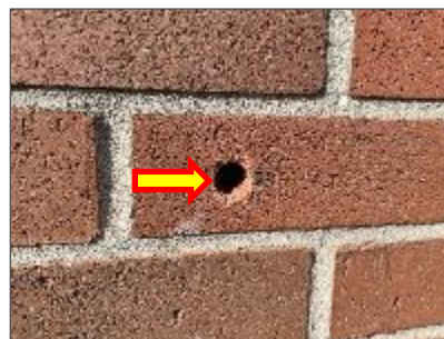
Vermiculite drill on exterior brick wall, Exterior (Loc. 1-27).
