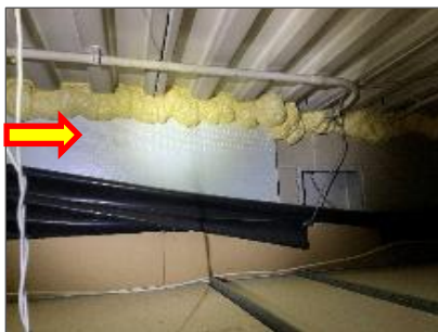
Presumed asbestos Transite panel at Dormitory Room and Kitchen/lounge walls above ceiling (Loc.1-09, 1-08).
