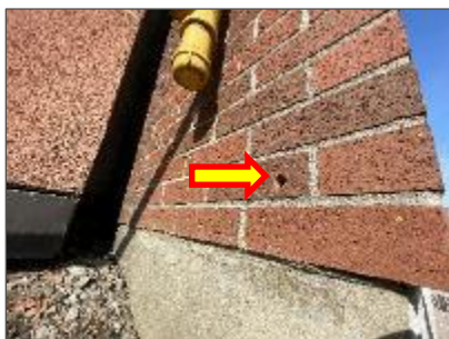
Vermiculite drill on exterior brick wall, Exterior (Loc. 1-27).
