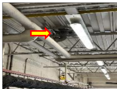
Presumed asbestos Transite rainwater leader pipe in the Fire Apparatus Bay area (Loc. 1-01).
