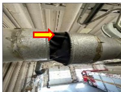
Presumed textile vibration damper present in the Fire Apparatus Bay area (Loc.1-01).
