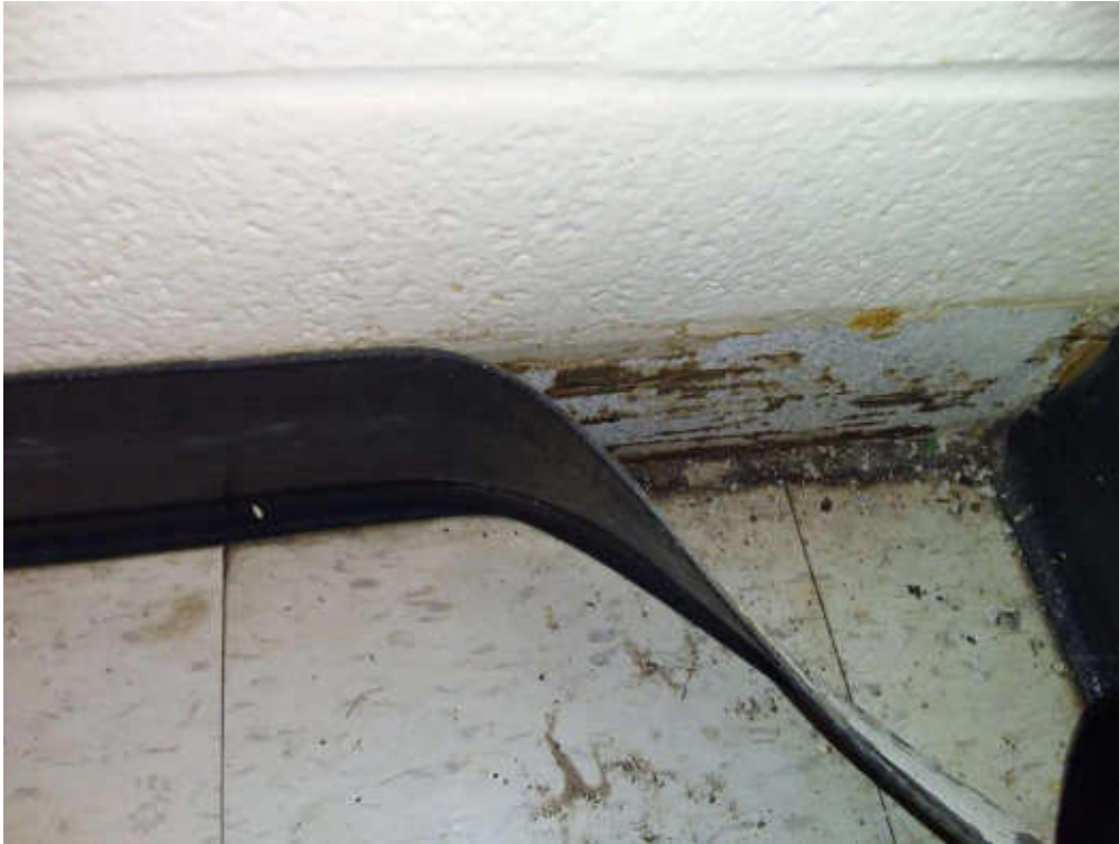
S0032A (Confirmed Asbestos on wall paint phase C ), Brown adhesive black vinyl trim on asbestos-containing primer paint, Wall, Adhesive/mastic, GIRLS WASHROOM (Location #: 53)
