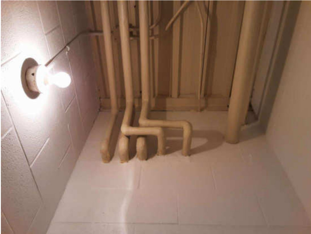
V0003 (Confirmed Asbestos), Parging Cement on Pipe Fittings, CUSTODIAN CLOSET (Location #: 54)
