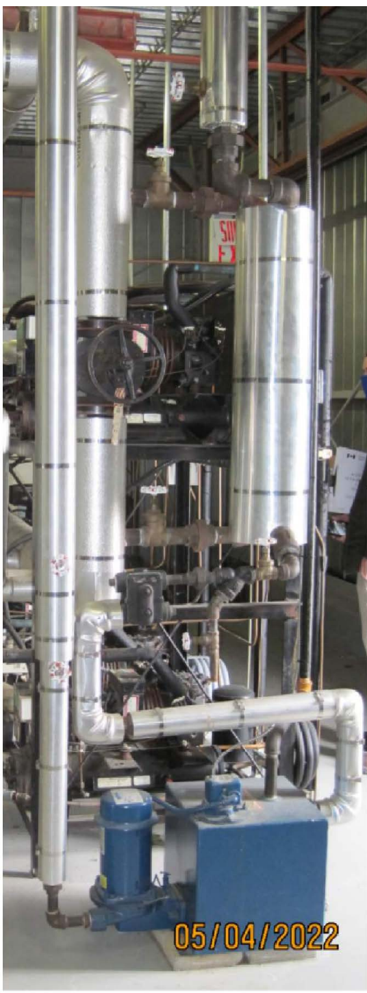
PHOTO 3: EXISTING STEAM-WATER REHEAT SYSTEM FOR CONDENSING WATER (REFER TO DRAWING 404 FOR SYSTEM LOCATION)
