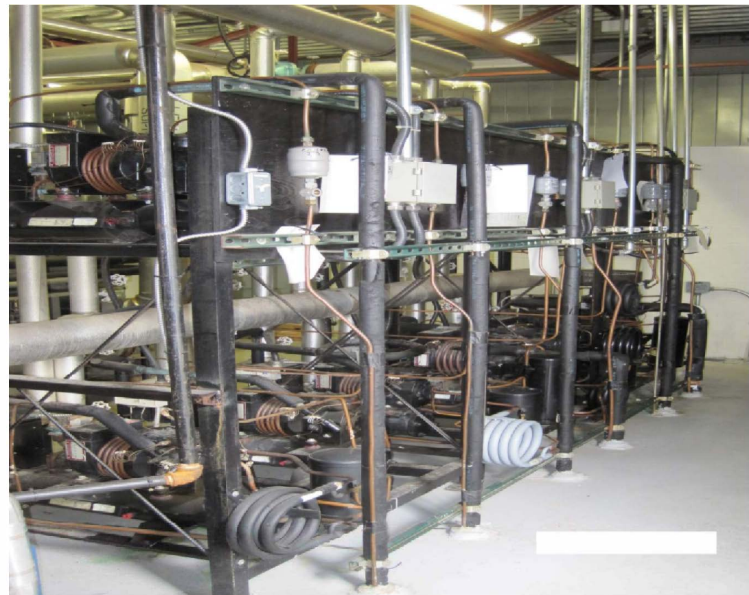
PHOTO 2: EXISTING COMPRESSOR/CONDENSING UNITS ON RACK (REFER TO DRAWING 404 FOR SYSTEM LOCATION)
