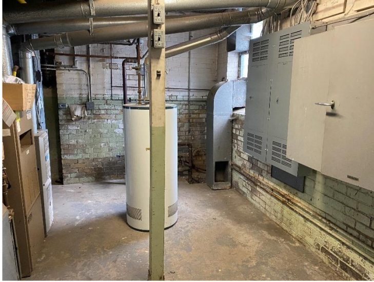
Picture 16: Elevated level of lead-containing white paint with yellow back layer on the basement wall.
