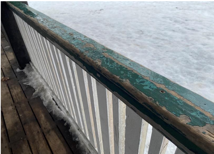
Picture 17: Elevated level of lead-containing green paint on the exterior structure.
