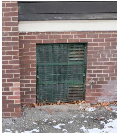
E15 – Window openings with ventilation louvers. Sill below grade for westernmost opening (asphalt surfacing). Windows to be restored. Refer to note E06
