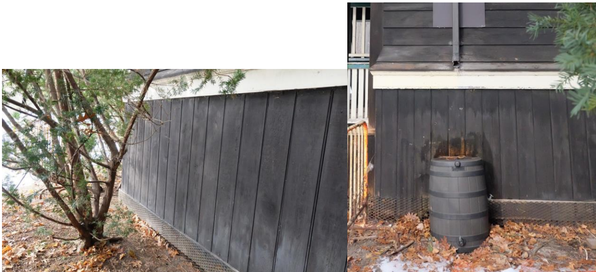
E32F - All vertically-oriented wood sheeting cladding on building perimeter in poor condition, to be removed and replaced. Sheeting damaged by weather and wildlife.
