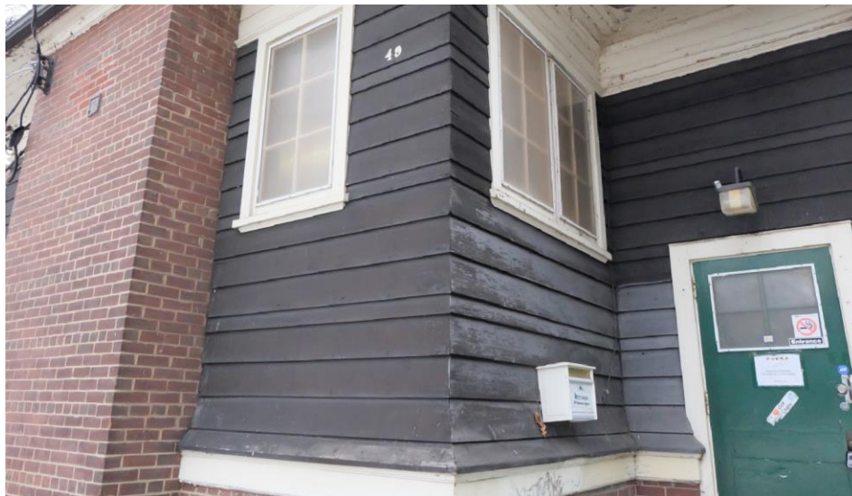
E16 - Horizontal wood siding – 2 lowest boards are patched at outside corner. Splintered boards along outside corner to be patched or replaced as needed. All rotten boards are to be replaced. Board species and profiles to match existing. Prime and paint.
