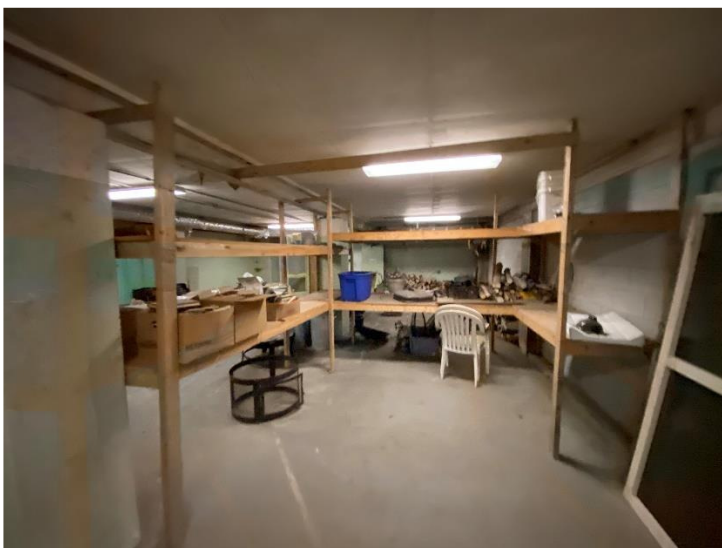
Picture 15: Elevated level of lead-containing light grey paint on the concrete floor of basement.
