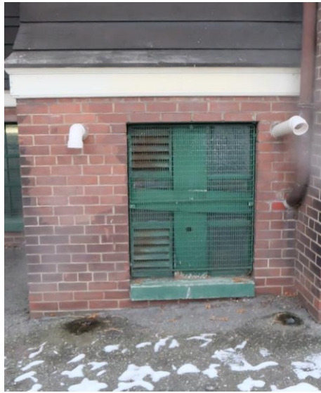
E15 – Window openings with ventilation louvers. Sill below grade for westernmost opening (asphalt surfacing). Windows to be restored. Refer to note E06
