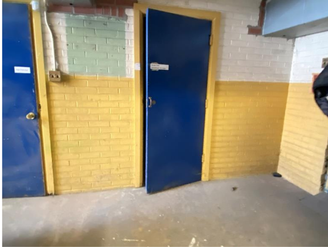
Picture 13: Elevated level of lead-containing yellow paint on a basement wall.
