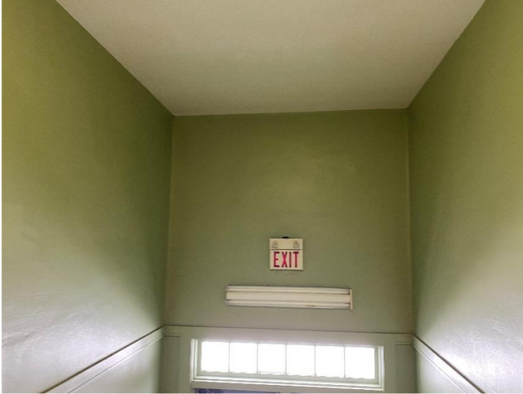
Picture 19: Elevated level of lead-containing light green paint on the wall.
