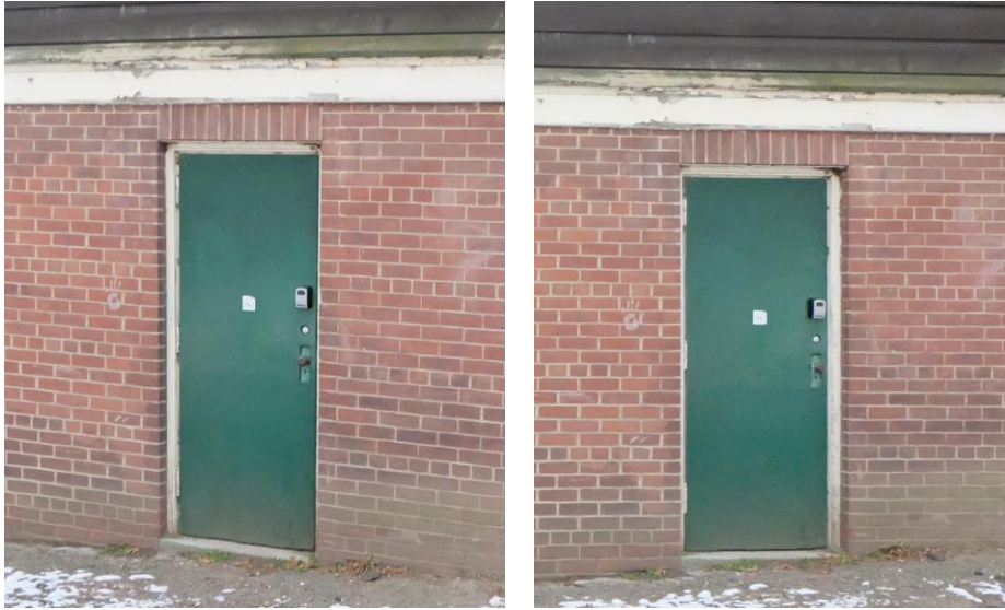
E27 – Existing metal storage room door and frame in poor condition - to be removed and replaced. Prime and paint.
