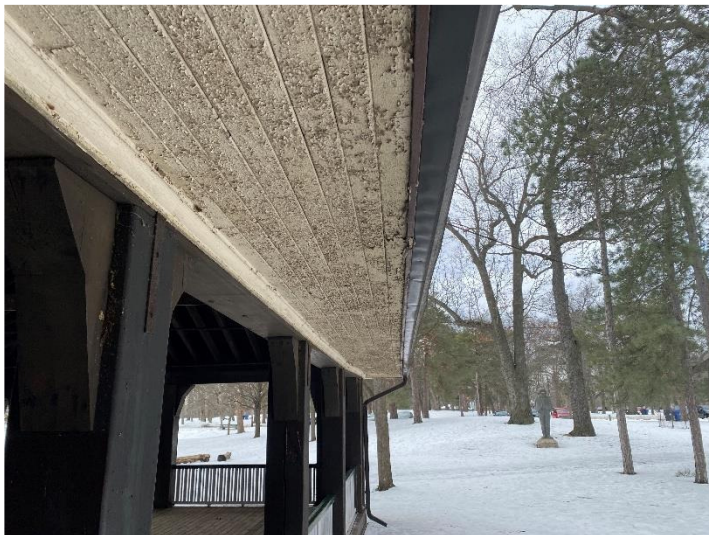
Picture 18: Elevated level of lead-containing white paint on the soffit.
