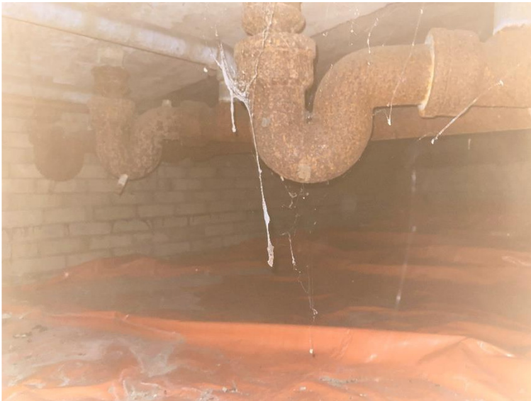
Picture 29: A view of non insulated pipe within the crawl space.
