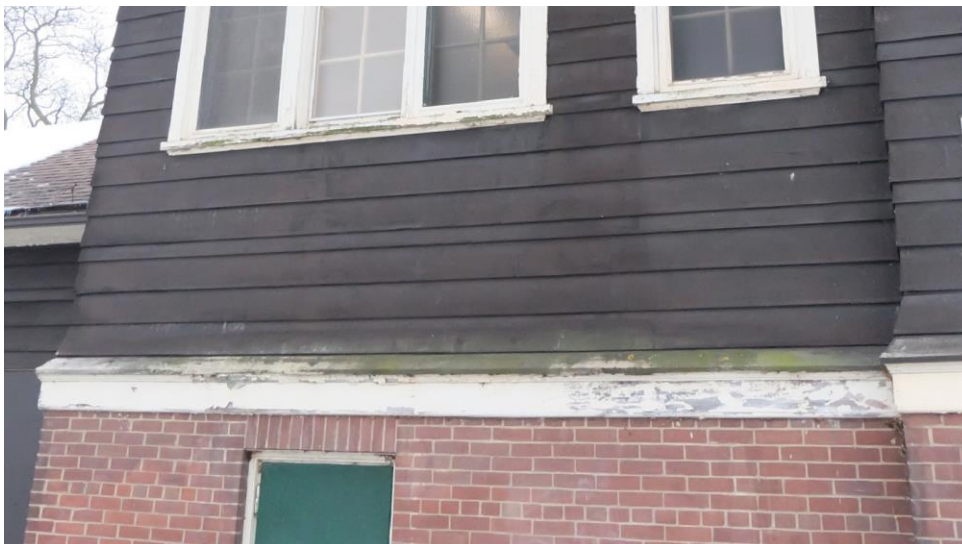
E28 – Horizontal wood siding – 2 lowest boards are moisture damaged. Splintered boards along outside corner to be replaced for full heights. Skirt board below siding appears to be moisture damaged. Boards to be replaced. Board species and profile to match existing. Prime and paint.
