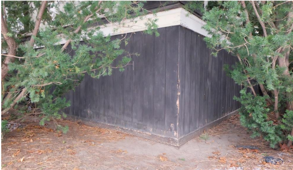
E32F & E32H- All vertically-oriented wood sheeting cladding on building perimeter in poor condition, to be removed and replaced. Sheeting damaged by weather and wildlife.
