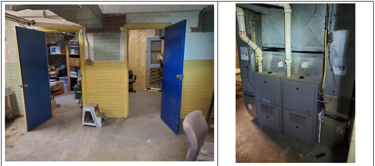
Figure 4: During testing interior doors within the test zone were propped open and forced air heating system was turned off.
