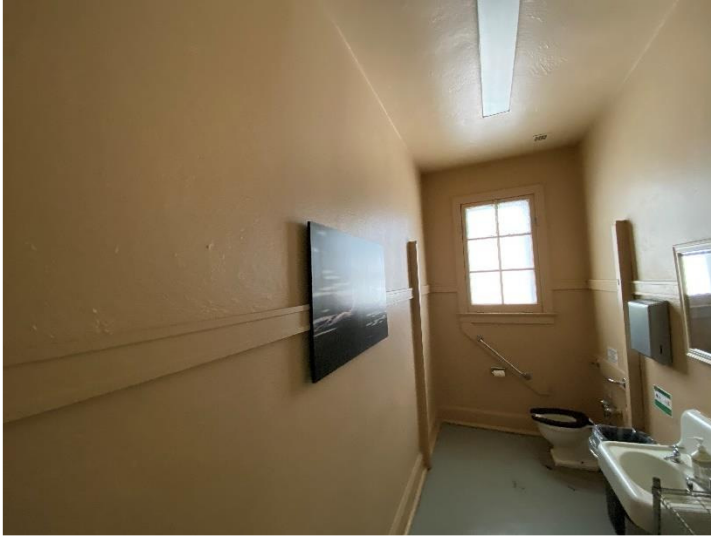
Picture 10: Elevated level of lead-containing brown paint on a wall in the washroom.
