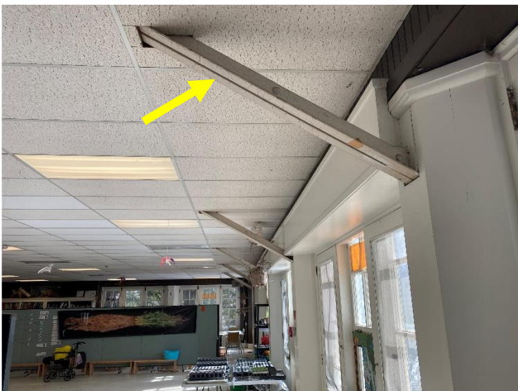
Picture 12: Elevated level of lead-containing white paint on the structural frames at the Site.
