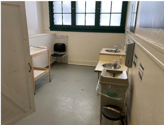
Picture 14: Elevated level of lead-containing dark grey paint on the concrete floor of washroom.
