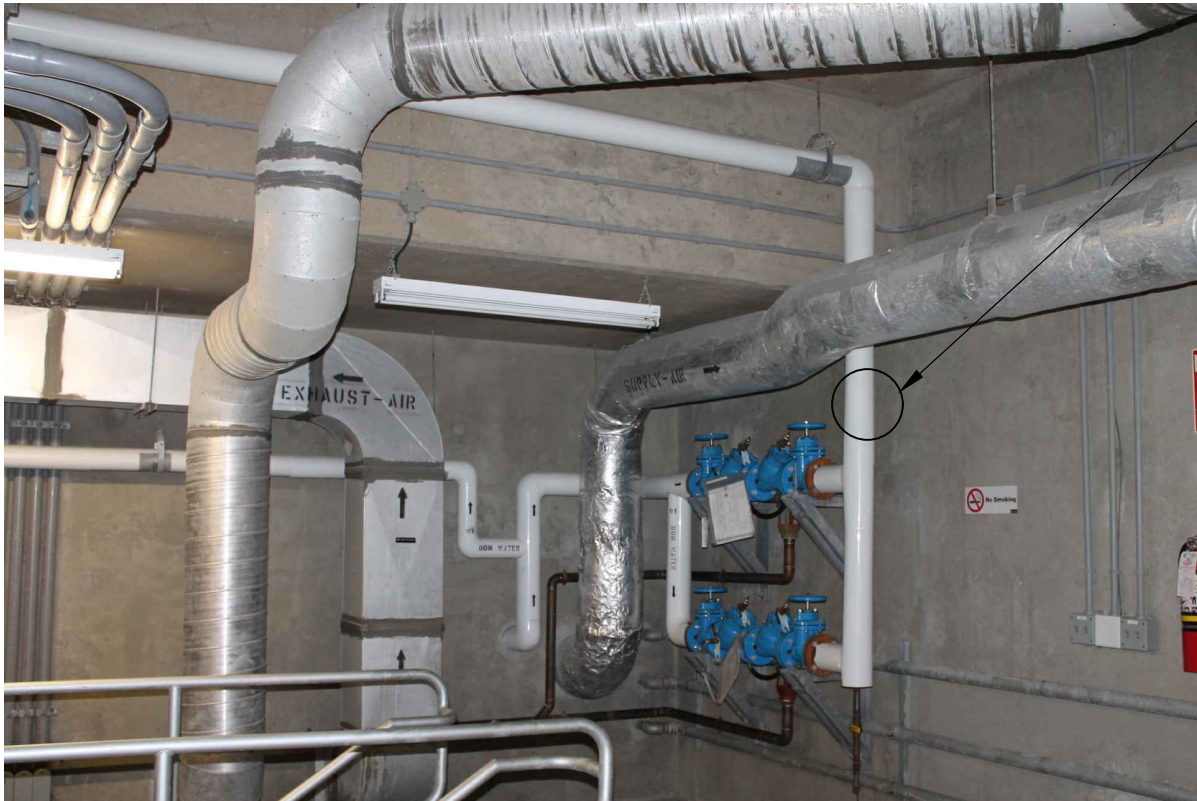
PHOTO 1 - SW CORNER OF PIPE GALLERY N.T.S.
