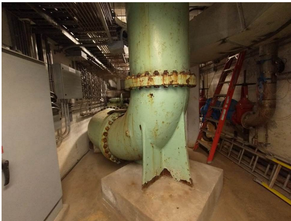
Photograph 30: View of the lead-containing green paint observed on pipe in the basement of the scrubber area in the Filter Building.
