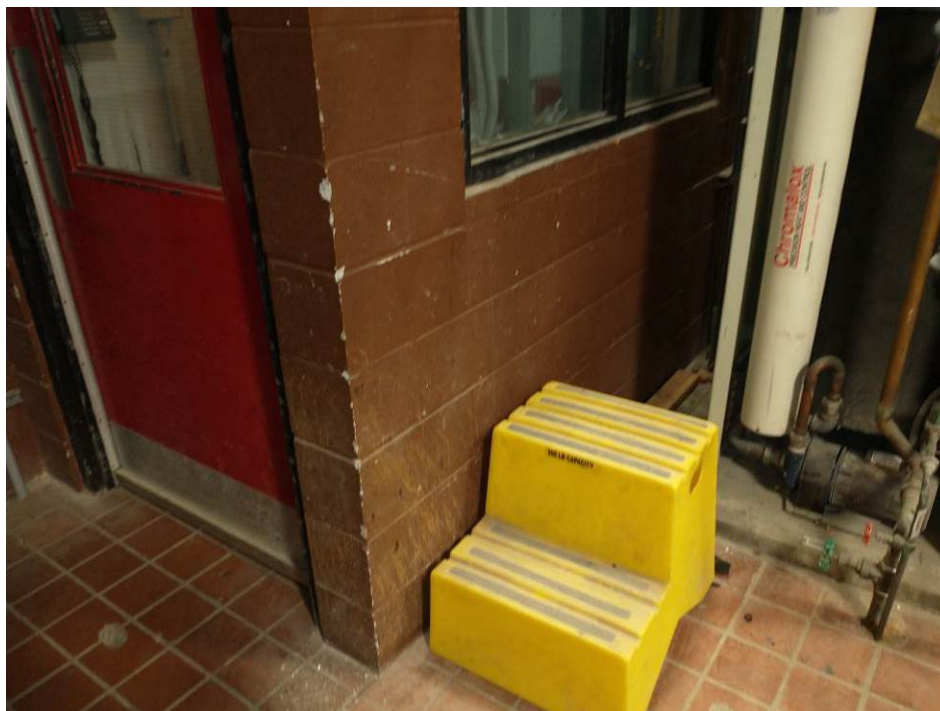
Photograph 29: View of the lead-containing brown paint observed on the concrete block wall on the ground floor of the Chlorine Storage Room in the Filter Building.
