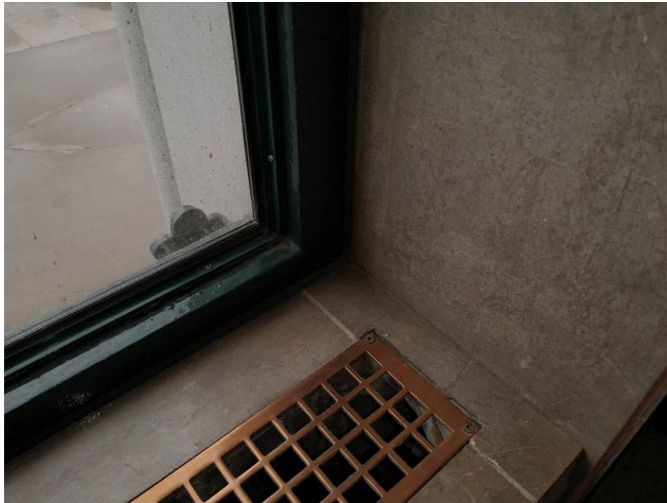
Photograph 7: View of the asbestos-containing grey interior window caulking observed in the stairwell on the 1 st floor of the Filter Building.
