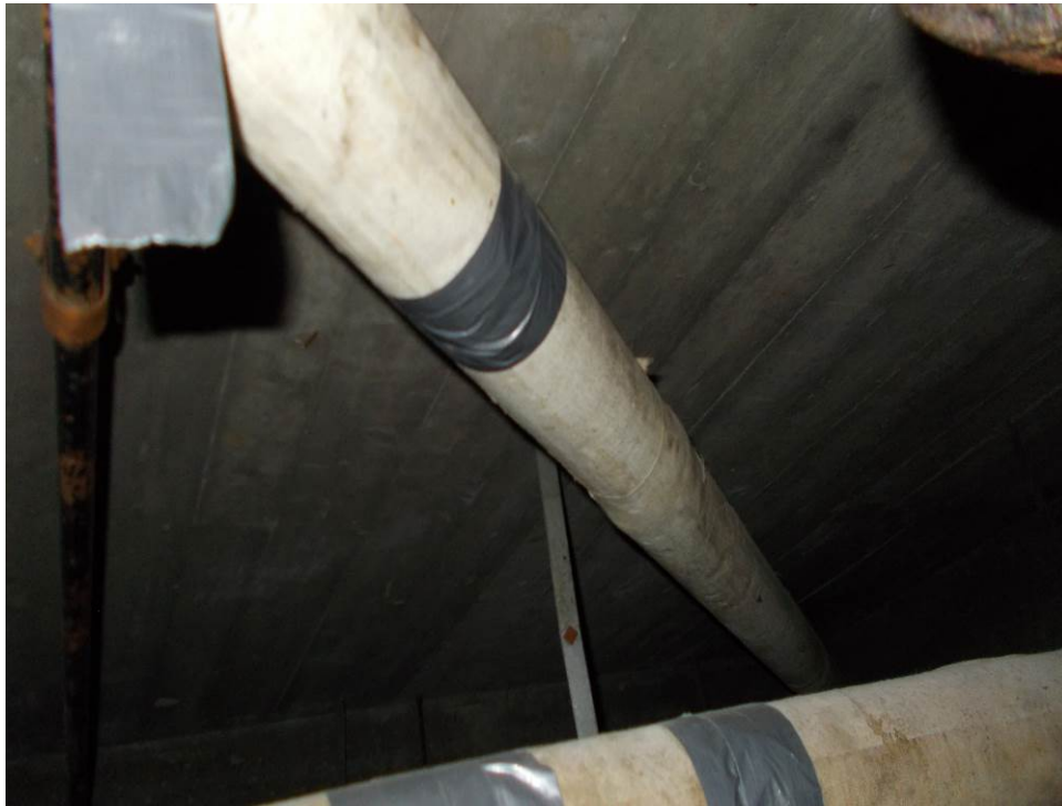
Photograph 9: Previous view of the asbestos-containing mechanical systems insulation in the form of air-cel present in the ceiling space (ceiling space now covered with drywall) in the lobby on the 1 st floor in the Administration Building (Filter Building).
