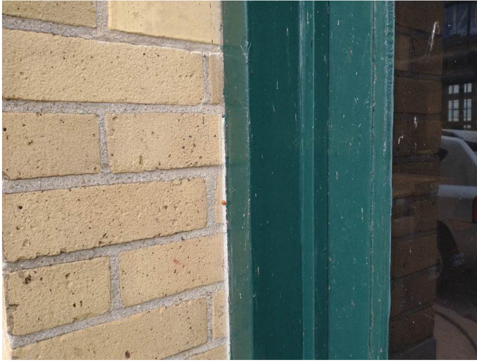
Photograph 25: View of the asbestos-containing white caulking observed around the exterior side of the door frame of boiler room of the Service Building.
