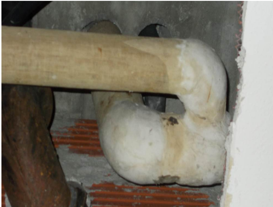
Photograph 20: View of the suspect asbestos-containing mechanical system pipe insulation previously observed concealed above the drywall ceiling at the entrance to the men's washroom in the hallway on the 2 nd floor of the Service Building.
