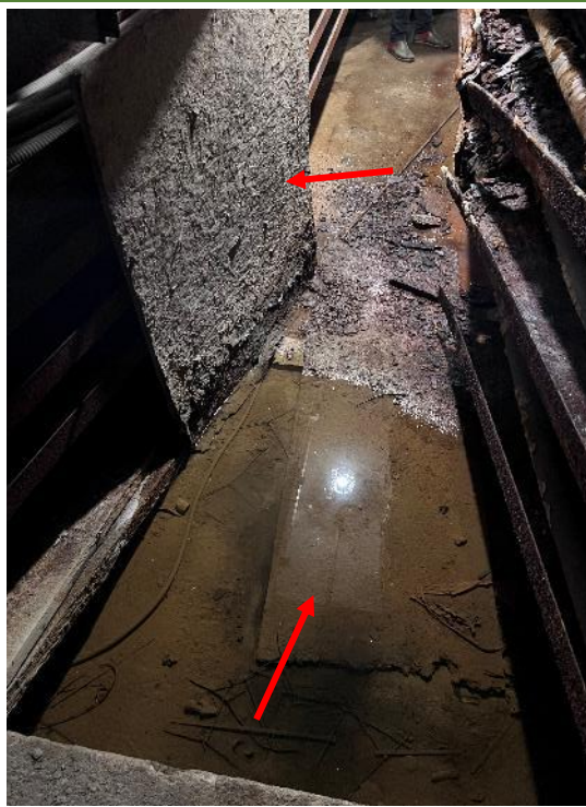
Photo 4: Representative photograph of mould-impacted and water-damaged wooden boards used to restrain water movement in the Tunnel Area.
