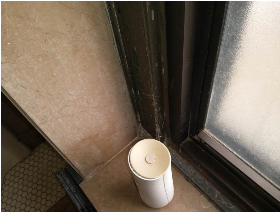
Photograph 6: View of the window in the 1 st floor washroom in the Filter Building. The previously reported damaged asbestos-containing window caulking was not observed directly since it was covered with new finishes.
