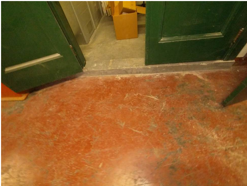
Photograph 16: View of the asbestos-containing red flooring with black layer on the floor of the storage room on the 1 st floor of the Pump Building.
