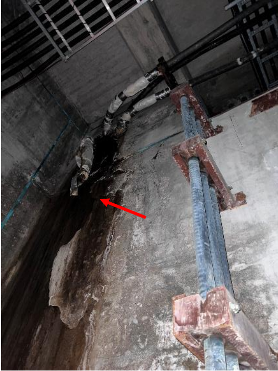
Photo 5: Representative photograph of mould-impacted concrete wall in the Tunnel Area.
