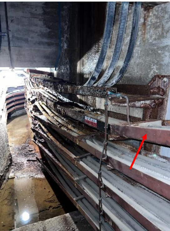
Photo 3: Representative photograph of lead-based reddish brown paint on cable trays.
