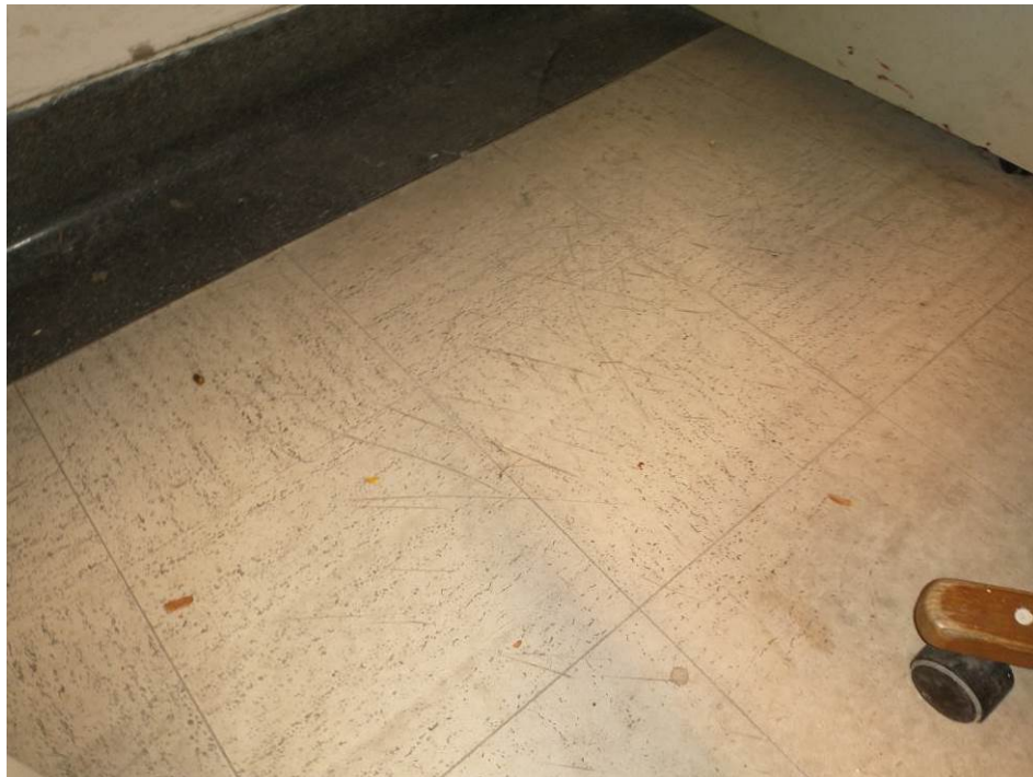
Photograph 14: View of the asbestos-containing 12" x 12" vinyl floor tiles observed in the west end office on the 1 st floor of the Pump Building.
