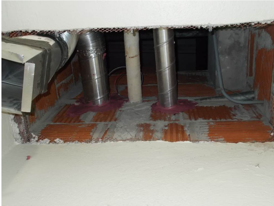
Photograph 17: Previous view of the asbestos-containing mechanical system insulation in form of magnesia block (covered with drywall) observed on the pipe straights in the men's washroom on 2 nd floor of the Pump Building.
