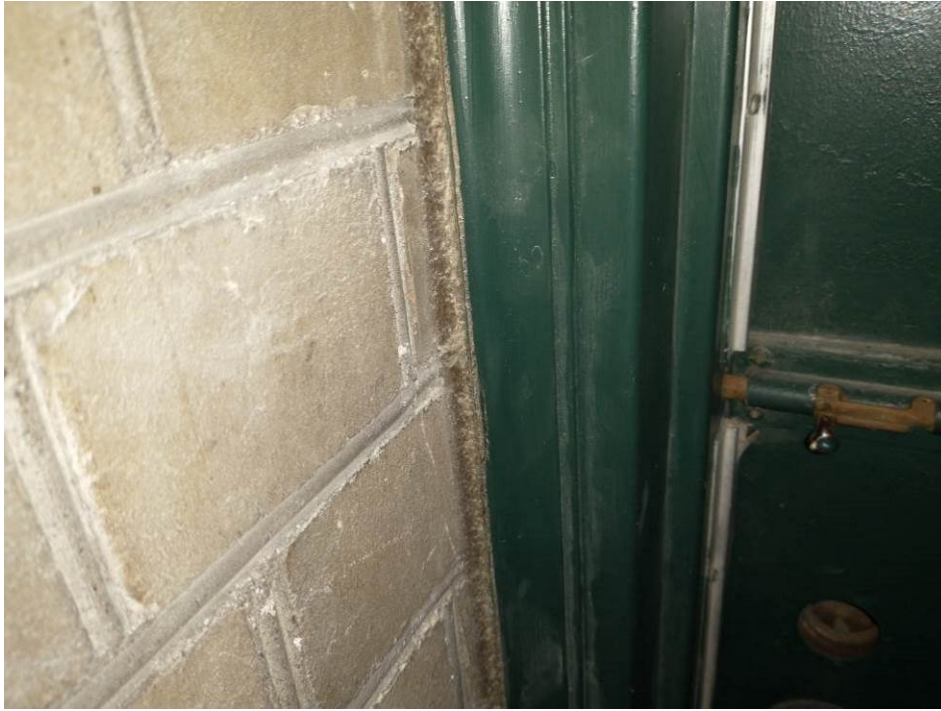
Photograph 21: View of the asbestos-containing black caulking between the door frame and the masonry wall observed on the 3 rd floor of the Service Building.
