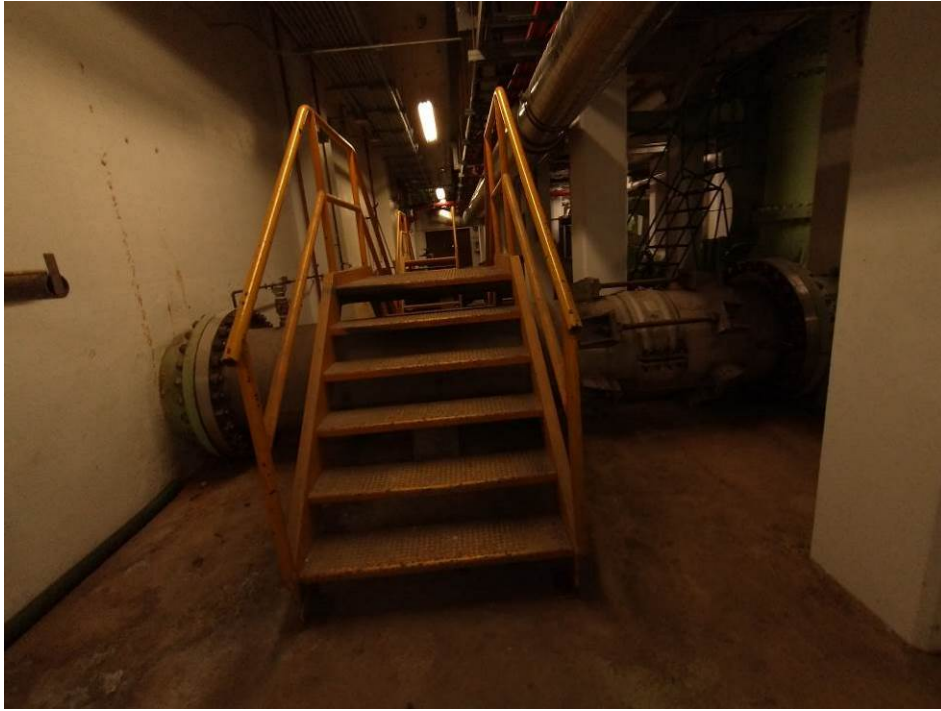
Photograph 27: View of the lead-containing yellow stair paint observed in the treated water pump room in the basement of the Pump Building.
