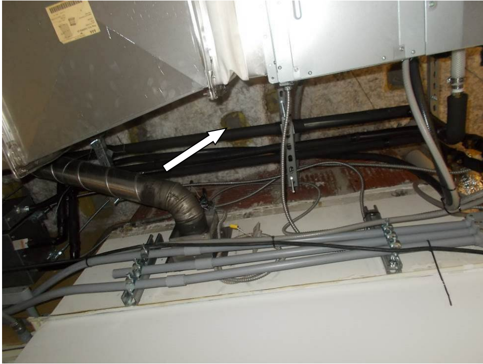
Photograph 1: View of the asbestos-containing mechanical linear pipe insulation observed in the hallway on the 2 nd floor of the Filter Building.
