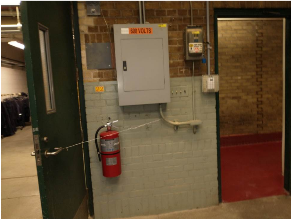
Photograph 26: View of the lead-containing green paint (newly painted) observed on the door of the storage room on the 1 st floor of the Service Building.
