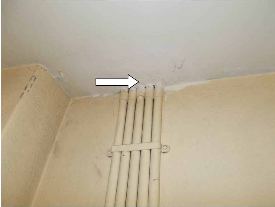
Photograph 19: Previous view of the asbestos-containing patch on the ceiling around the conduit penetrations into the ceiling of the storage room on the 1 st floor of the Pump Building.
