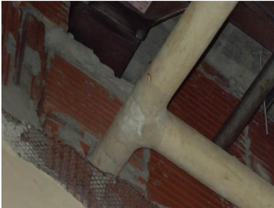
Photograph 18: Previous view of the asbestos-containing mechanical system insulation in form of parging cement (covered with drywall) observed on the pipe fittings in the men's washroom on the 2 nd floor of the Pump Building.
