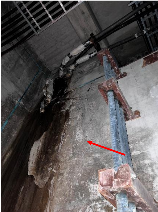
Photo 1: Representative photograph of non-asbestos plaster patching on concrete wall.
