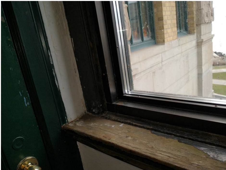
Photograph 2: View of the asbestos-containing interior window caulking painted brown observed in the hallway on the 2 nd floor of the Filter Building.
