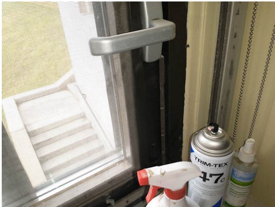
Photograph 10: View of the new windows where asbestos-containing window caulking is still potentially present in the control room of the Filter Building.
