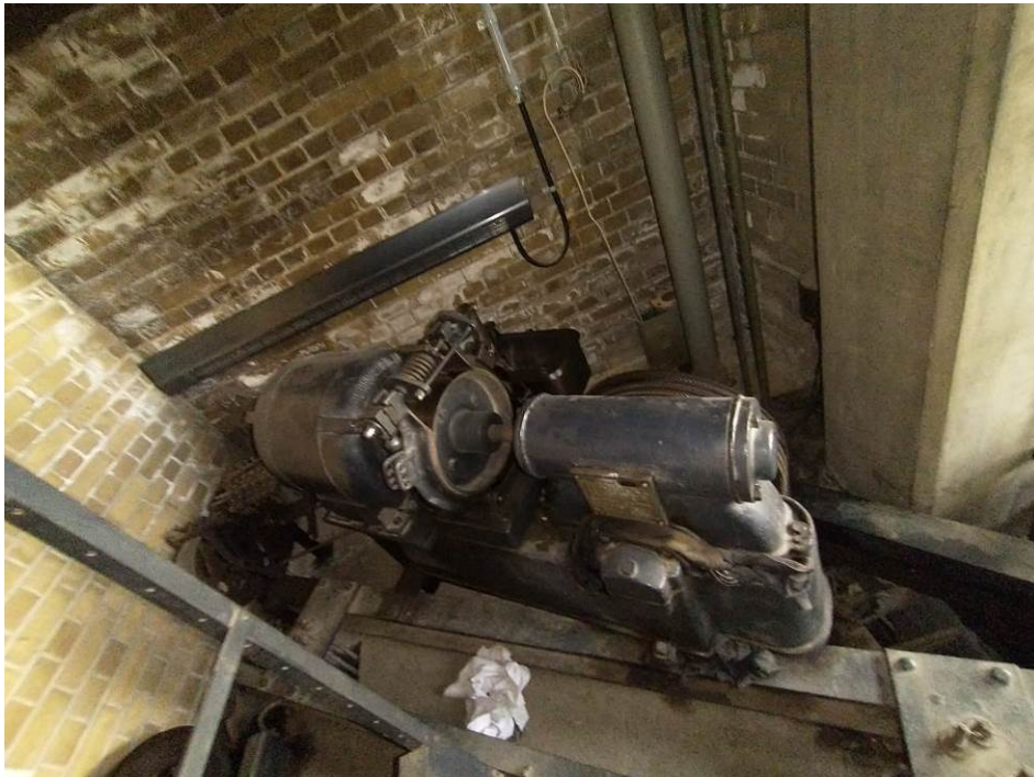
Photograph 24: View of the suspect asbestos-containing elevator brake pads observed on the 5 th floor of the Service Building.
