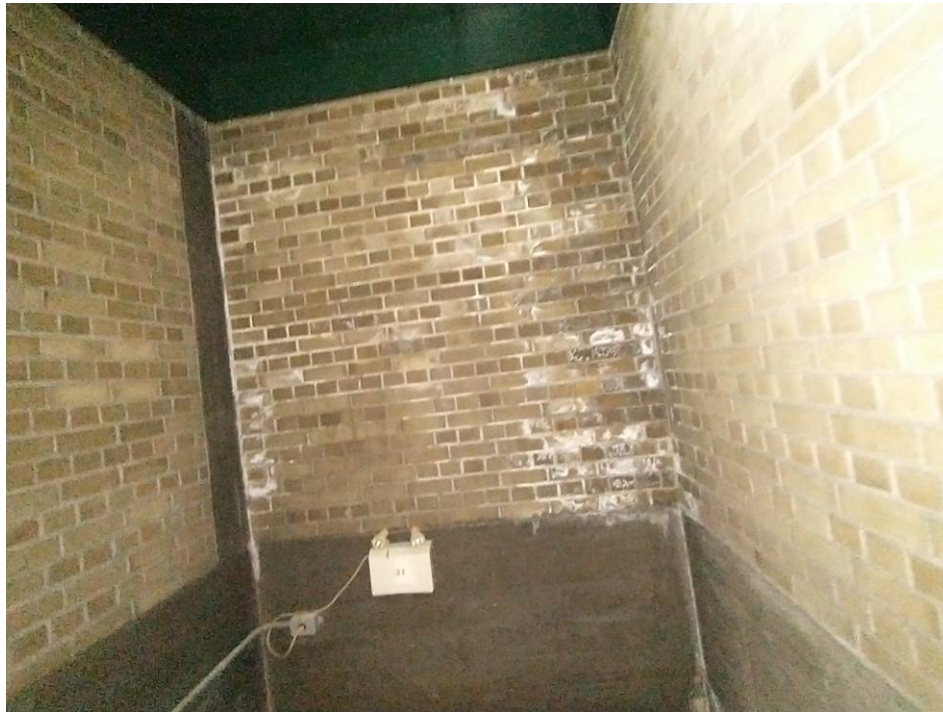
Photograph 31: View of the water damage (i.e. staining and efflorescence) observed on the wall in the stairwell on the 4 th floor of the Service Building.
