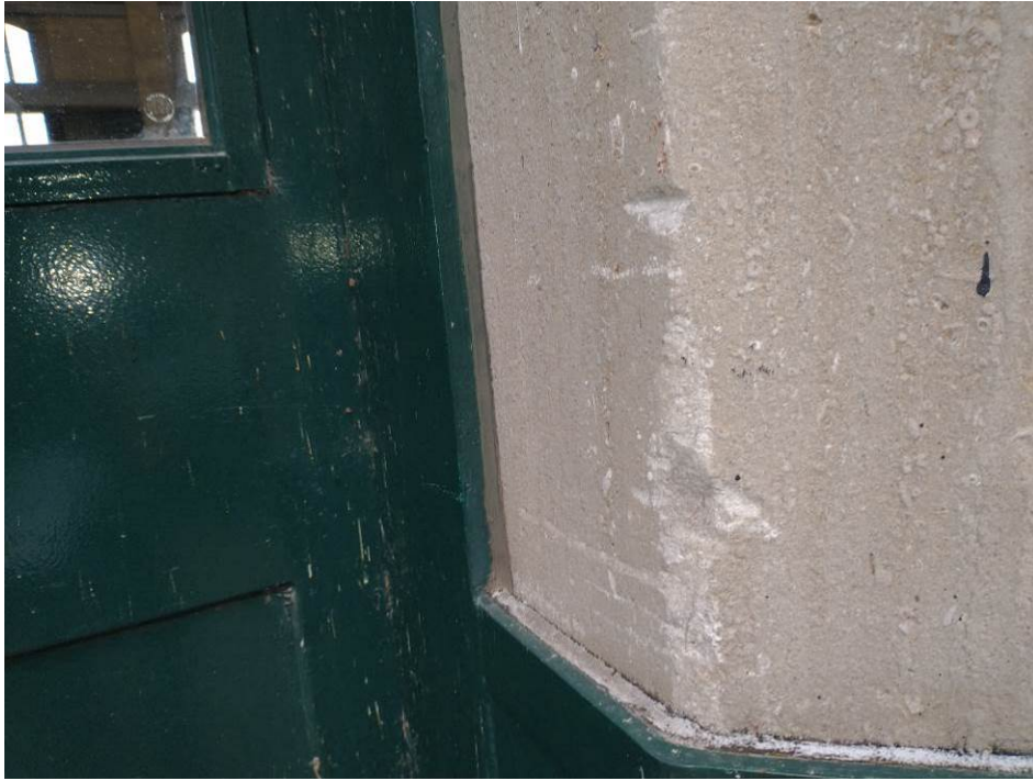
Photograph 15: View of the asbestos-containing grey window caulking observed on the exterior of the Pump Building.
