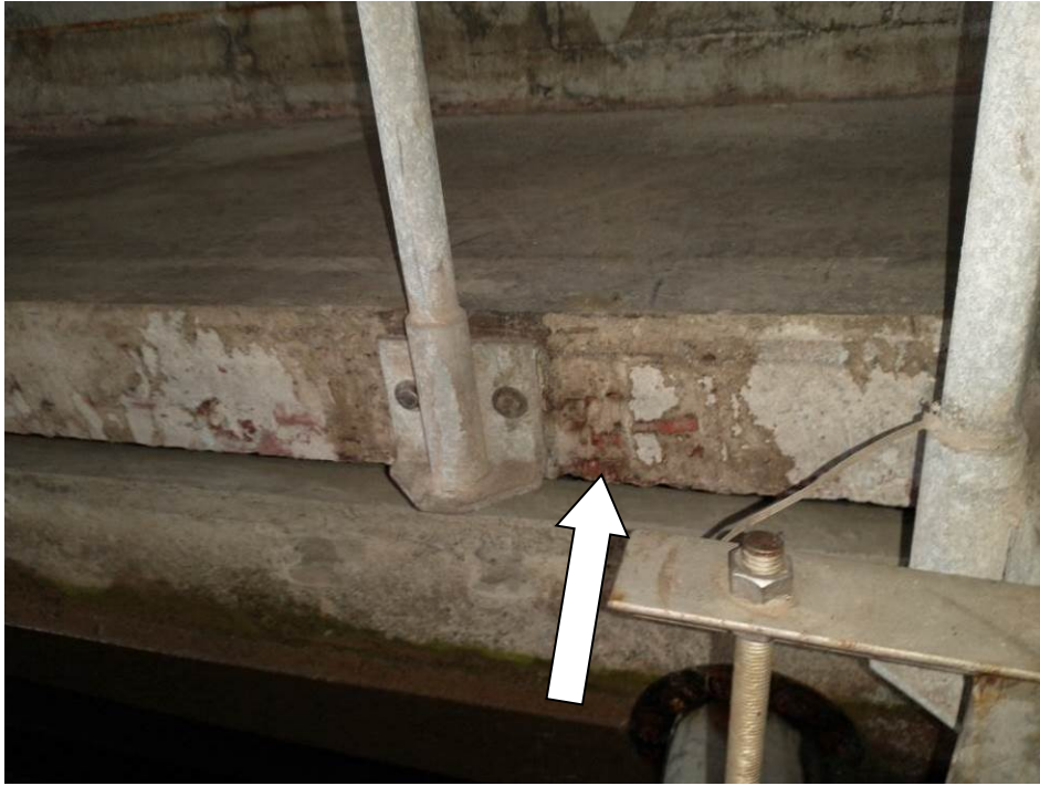
Photograph 11: View of the remnants of red floor coating observed in the northwest filter gallery of the Filtration Building.
