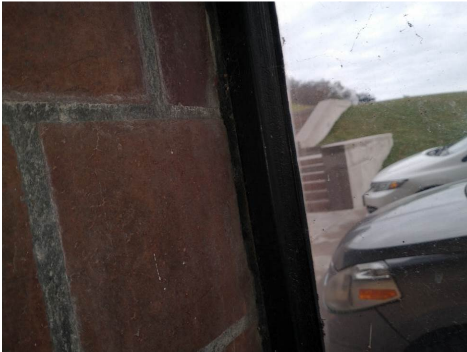
Photograph 22: View of the asbestos-containing interior window caulking observed on the 4 th floor of the Service Building.
