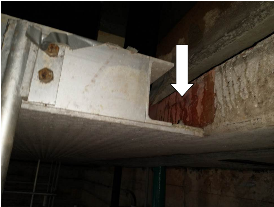
Photograph 12: View of the remnants of red floor coating observed in the southwest filter gallery of the Filtration Building.
