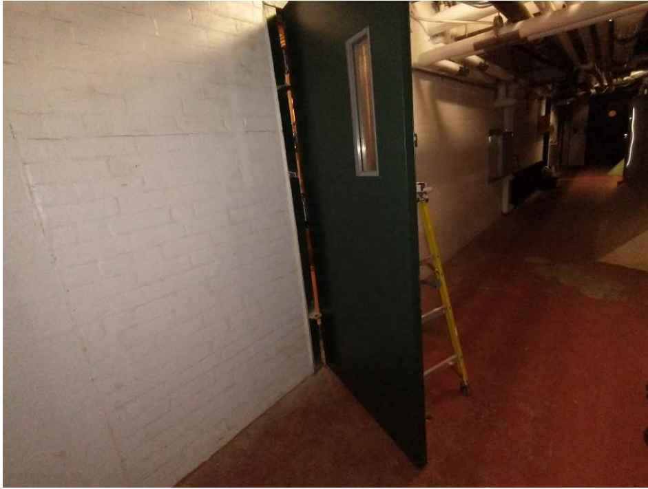
Photograph 5: View of the suspect asbestos-containing fire rated door observed in the basement corridor of the Filter Building.
