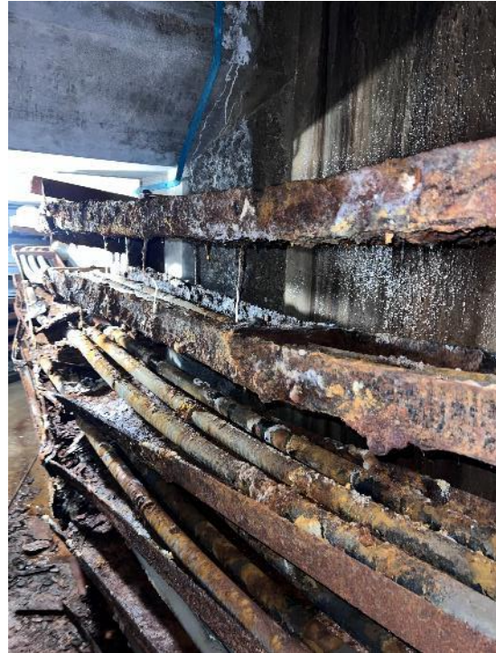
Photo 6: Representative photograph of water-damaged cable trays and mould-impacted concrete wall in the Tunnel Area.
