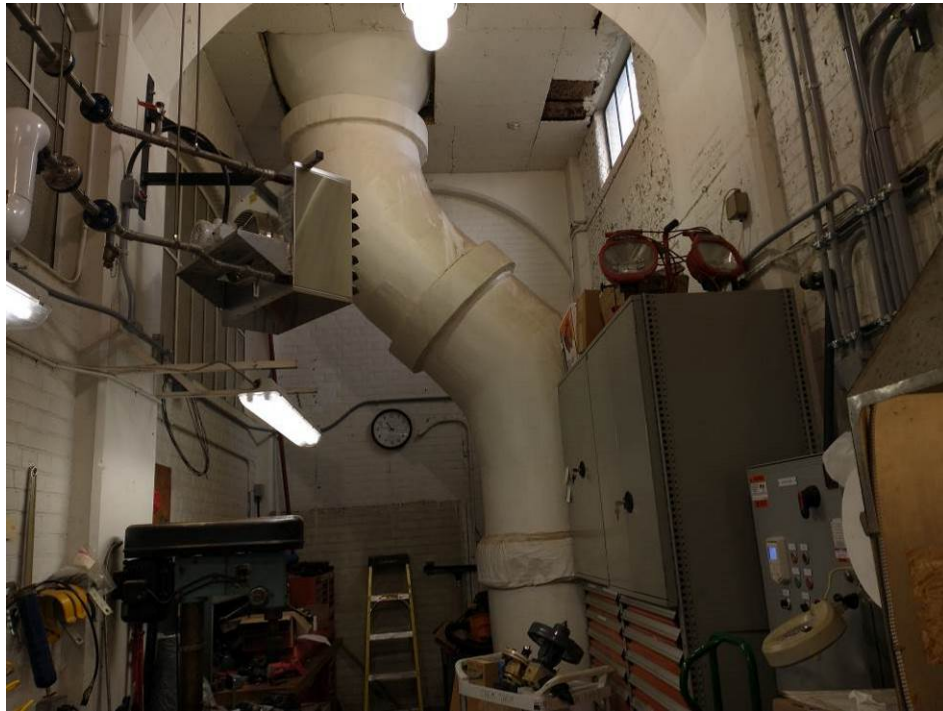
Photograph 13: View of a pipe reported by onsite staff to have mechanical systems insulation suspected of containing asbestos observed in the workshop in the Filtration Building.
