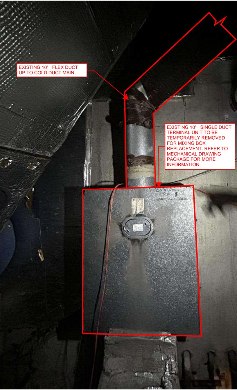
EXISTING MIXING BOX TO BE REMOVED AND REPLACED AS PER MECHANICAL DRAWING PACKAGE. (MIXING BOX APPROXIMATELY WHERE RED BOARDER IS SHOWN.)
