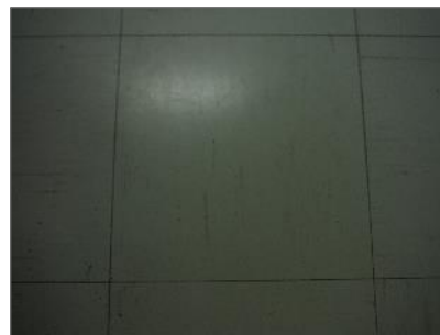
Photo 4: Asbestos-containing VFT03 (mastic is non-asbestos).
