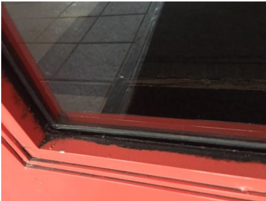
Photos 1, 2 – View of the asbestos-containing black putty in the door between frame and glass.
