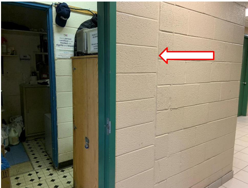
Photo 1 & 2: ACM – Tan caulking along the joint of the block walls.
