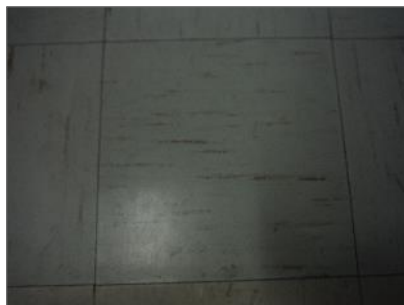
Photo 3: Asbestos-containing VFT01 (mastic is non-asbestos).
