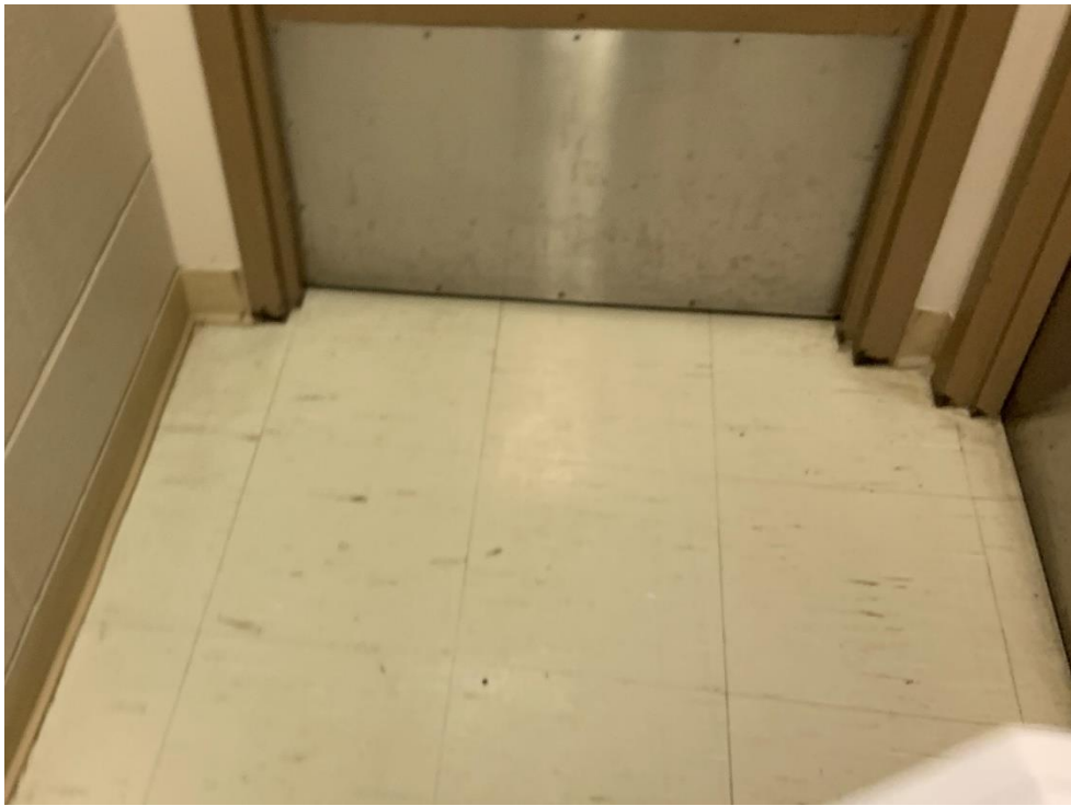
Photo 1: View of the asbestos-containing vinyl floor tile (12"x12" Beige with White and Brown Streak) in the basement corridor.
