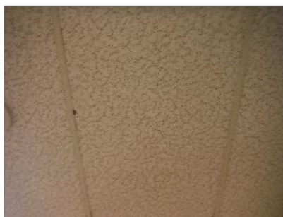
Photo 2: Assumed asbestos-containing ACT02.
