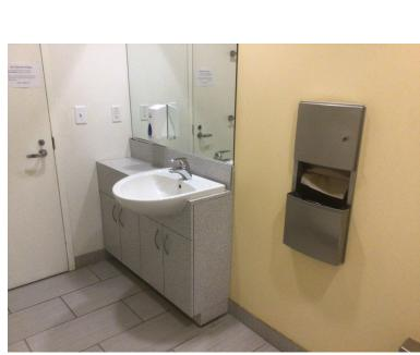
PHOTO 4: REMOVE EXISTING MILLWORK, SINK AND THE MIRROR
