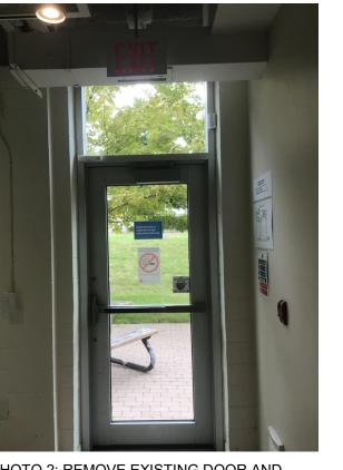
PHOTO 2: REMOVE EXISTING DOOR AND WIDEN THE OPENING TO RECEIVE NEW
