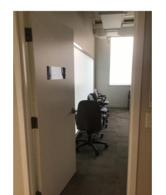
PHOTO 3: REMOVE EXISTING DOOR AND WIDEN THE OPENING TO RECEIVE NEW DOOR AT ROOM 207
